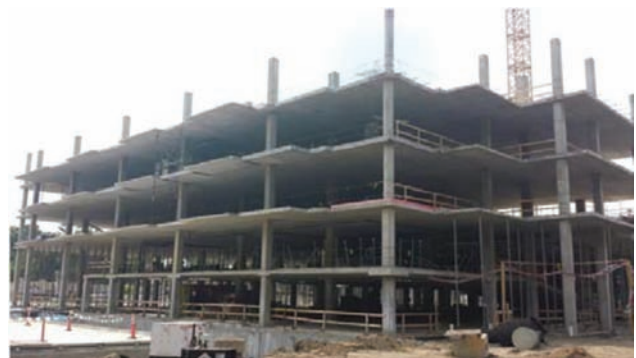
Figure 3.7 Reinforced concrete structure. (Source: https://www.designingbuildings.co.uk/wiki/Concrete_frame )
