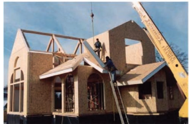
Figure 3.1 Structural insulated panels. (Source: https://www.cascadetimberframes.com/sip-panels/ )
