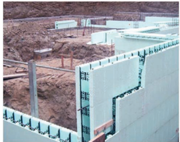
Figure 3.9 Insulated concrete form structure. (Source: https://decentralizedinc.com/the-anatomy-of-an-icf-wall/ )
