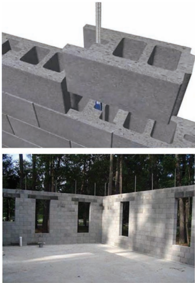
Figure 3.8 FlexLock block structure. (Source: https://www.seminarsonly.com/Civil_Engineering/mortarless-system.php )
