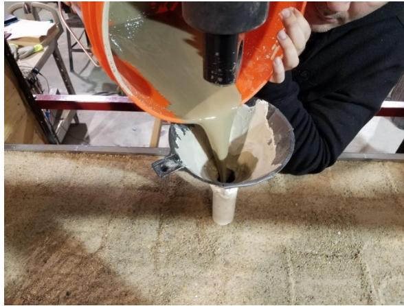
Figure 5.5: Pouring grout into the annulus through a drop tube
