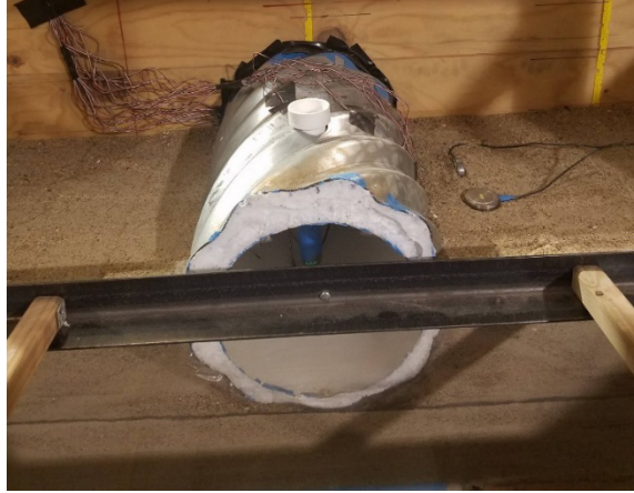
Figure 5.4: Placed steel pipe and liner
