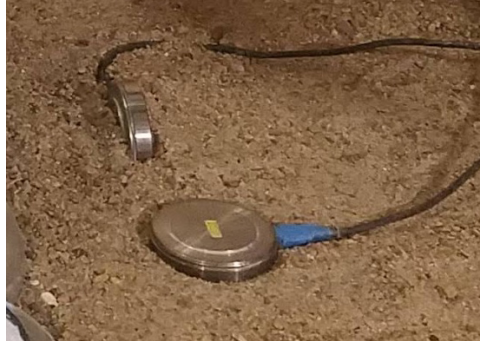
Figure 5.2: Earth pressure cells
