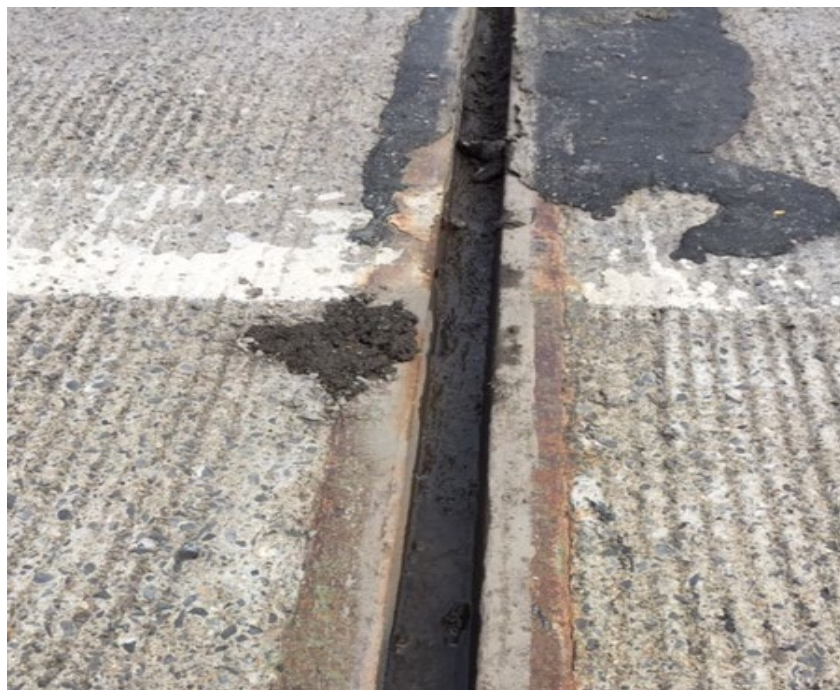
Figure 14. Bridge expansion joint after cleaning
