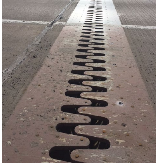
Figure 1. Interlaced finger type bridge expansion joint
