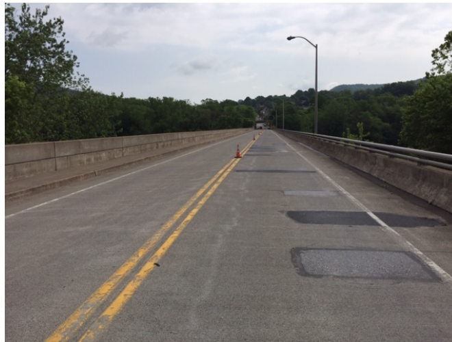
Figure 10. Demonstration site, Route 17 Bridge, Millerstown, PA
