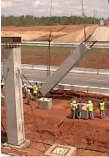
(a) example of full-height precast column
