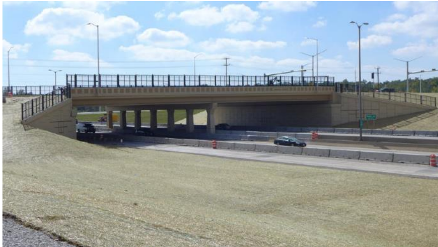
Figure 2-79: Completed Rawson Avenue Bridge (Olivia 2014)
