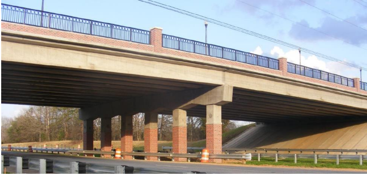
Figure 2-40: Elevation of New Moore's Mill Bridge after construction (City of Auburn 2019)
