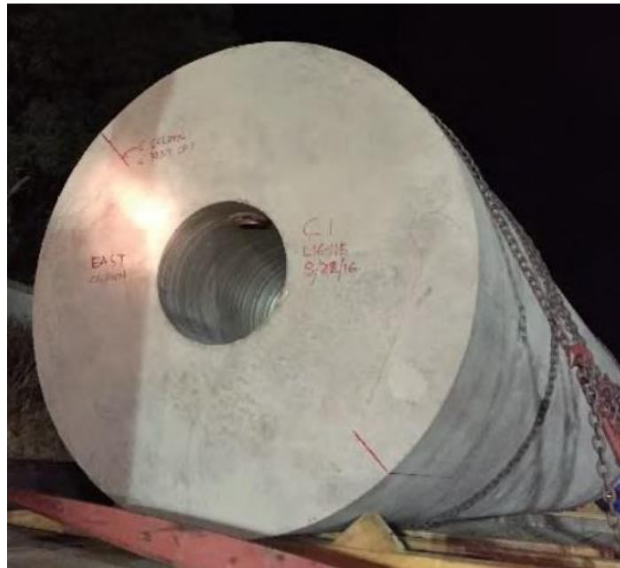
Figure 2-41: Precast column in Laurel Street Overcrossing (Mellon 2018)
