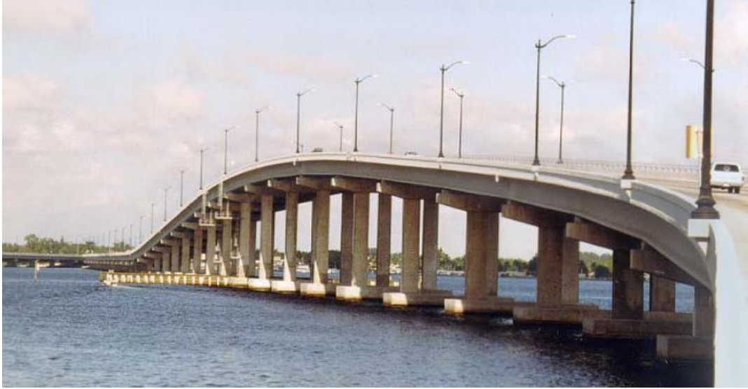
Figure 2-48: Edison Bridge after the completion of construction (FHWA 2009)
