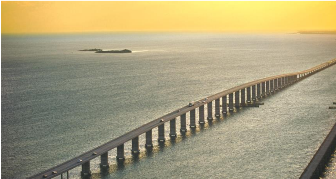
Figure 2-45: Seven Mile Bridge after construction (FIGG Bridge Group- www.figgbridge.com )
