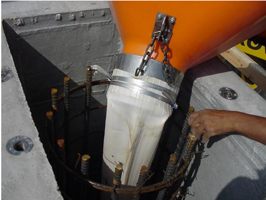
Figure 2-69: Precast column shells before core filling, LP 340 over IH 35 (Wolf 2005)
