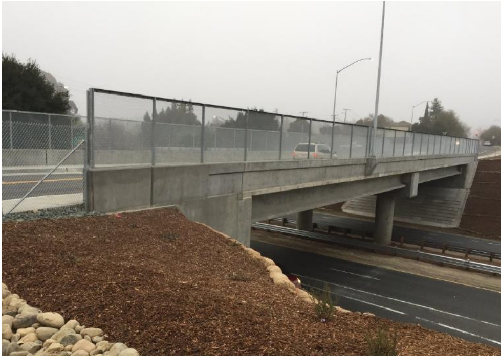
Figure 2-44: Laurel Street Overcrossing after construction (Mellon 2018)
