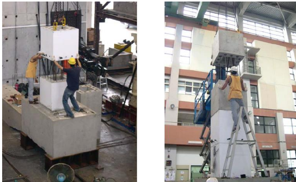
Figure 2-30: Construction of precast column specimen tested by Yu-Chen (2007)
