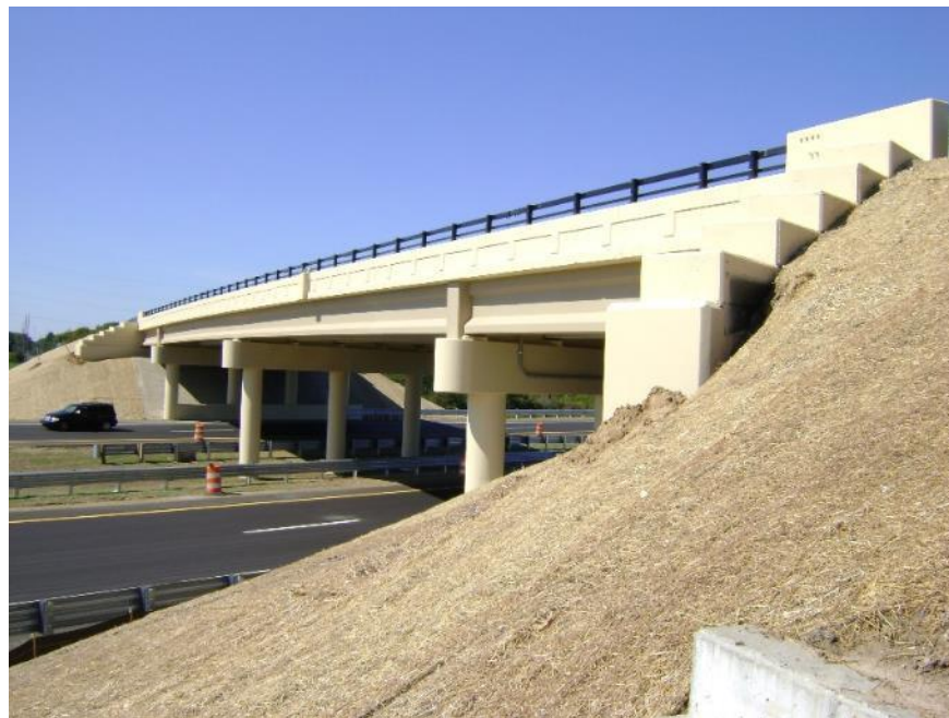
Figure 2-59: Parkview Avenue Bridge in service (Attanyake et al. 2012)
