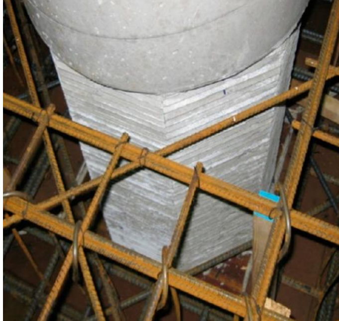
Figure 2-28: Socket connection proposed by Haraldsson et al. (2013)
