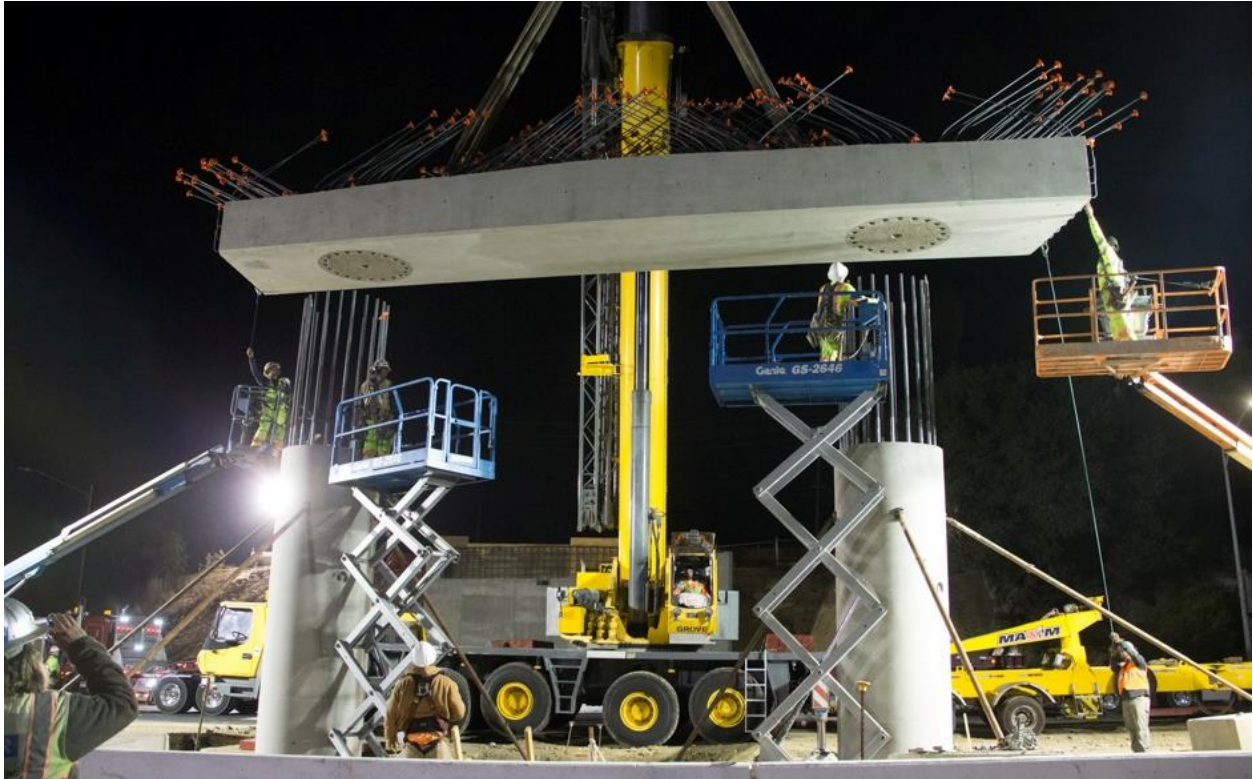
Figure 2-43: Erection of precast bent cap in Laurel Street Overcrossing (Mellon 2018)
