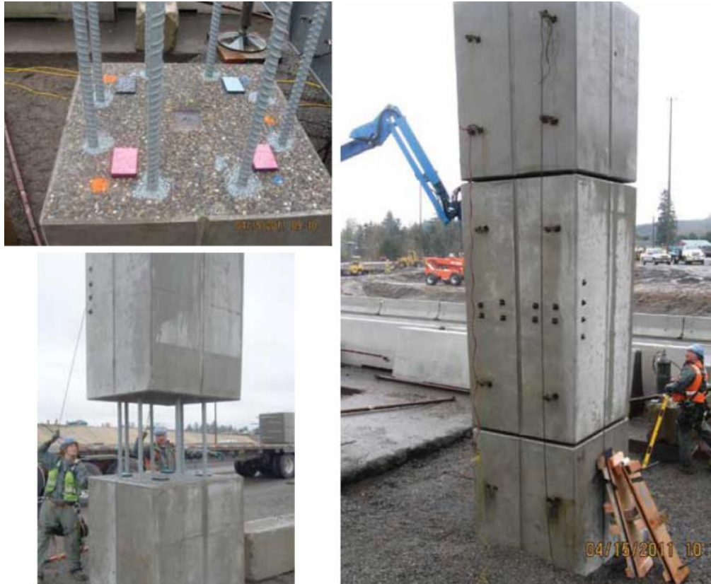
Figure 2-77: Placement of column segments in US 12 bridge (Khalegi et al. 2012)
