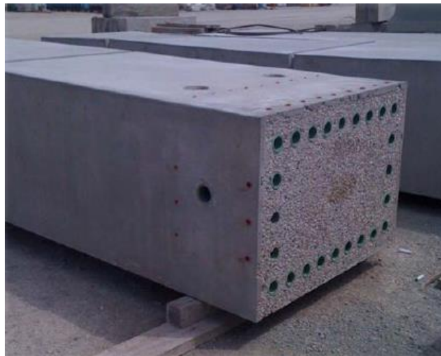
Figure 2-82: Precast column in Rawson Avenue (Olivia 2014)
