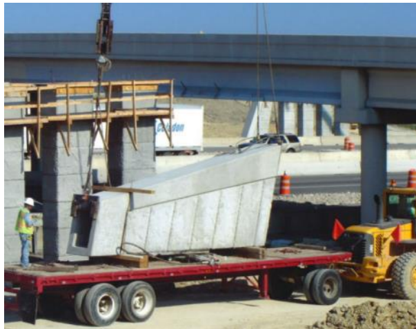
Figure 2-66: Shipping precast column shells into place, LP 340 over IH 35 (Wolf 2005)
