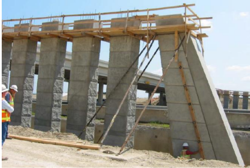
Figure 2-68: Precast column shells before core filling, LP 340 over IH 35 (Wolf 2005)
