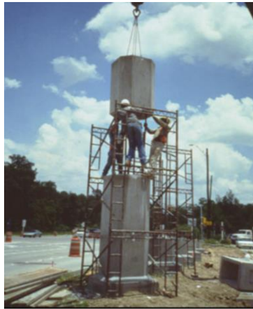
Figure 2-64: Assembly of Precast Segmental Columns in Louetta Road Overpass (Hewes 2013)
