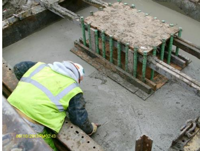
Figure 2-81: Bars extended from the footing in Rawson Avenue (Olivia 2014)
