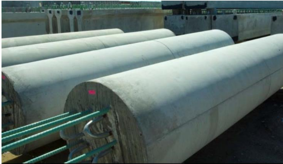
Figure 2-56: Precast columns in casting yard in Parkview Avenue Bridge (Attanyake et al. 2012)
