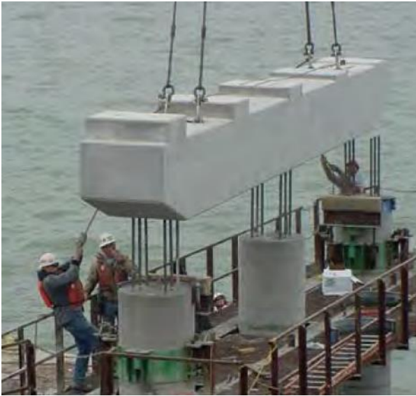
(b) Placement of precast concrete bent cap
