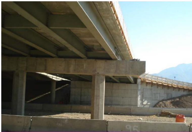
Figure 2-74: Riverdale Road Bridge in Utah (Burns 2008)
