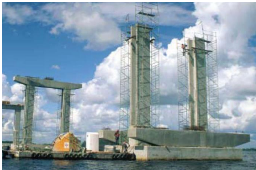
Figure 2-47: Erection of Precast Bents on Edison Bridge (Ericson 2005)
