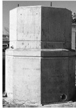
(b) Base joint cast in place
