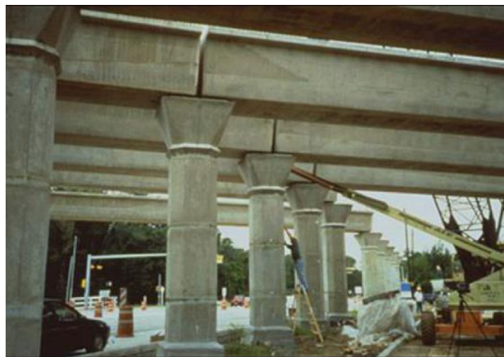
Figure 2-65: Completed Precast Columns and Cap in Louetta Road Overpass (Hewes 2013)
