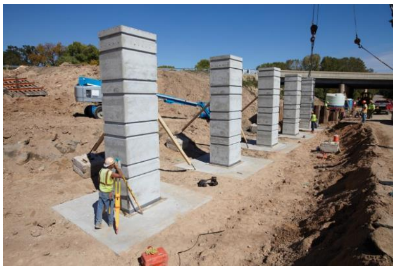
Figure 2-85: Precast columns after being erected, Siggelkow Road Bridge (source: www.countymaterials.com )
