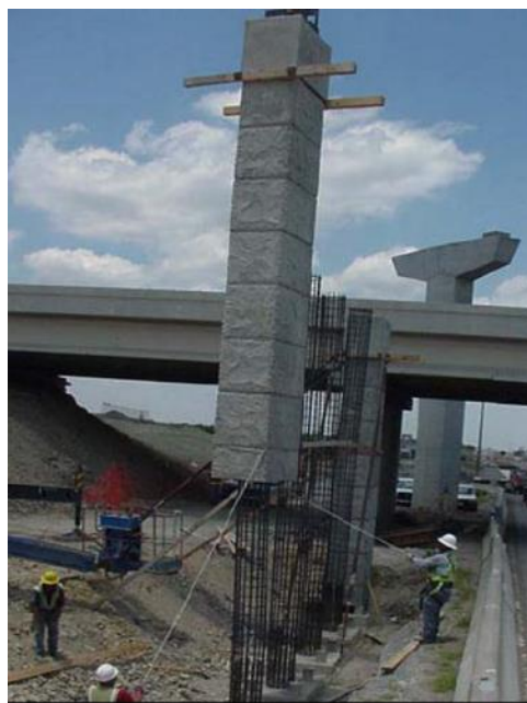
Figure 2-67: Lifting precast column shells into place, LP 340 over IH 35 (Wolf 2005)
