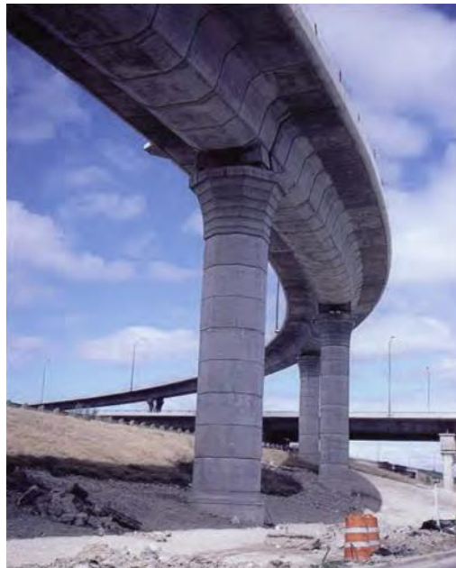
Figure 2-71: Completed US 183 Elevated Highway (Billington et al. 1998)
