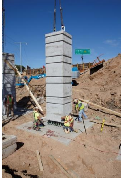
Figure 2-84: Precast column during placement, Siggelkow Road Bridge (source: www.countymaterials.com )
