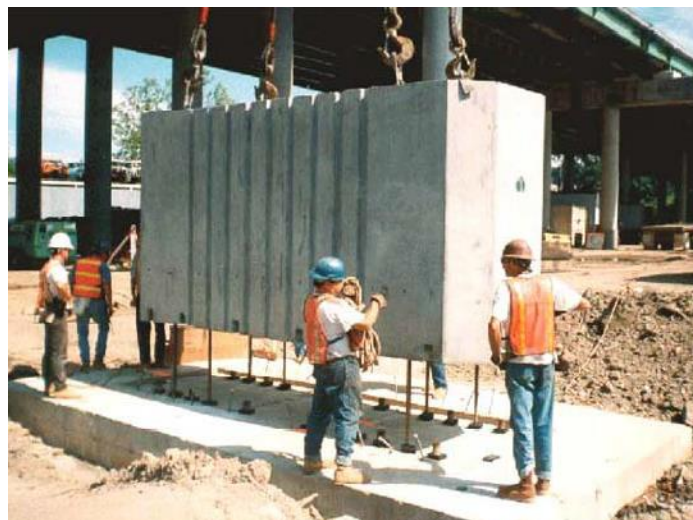
Figure 2-61: Pier-footing connection in Cross Westchester Expressway Viaduct (FHWA 2009)
