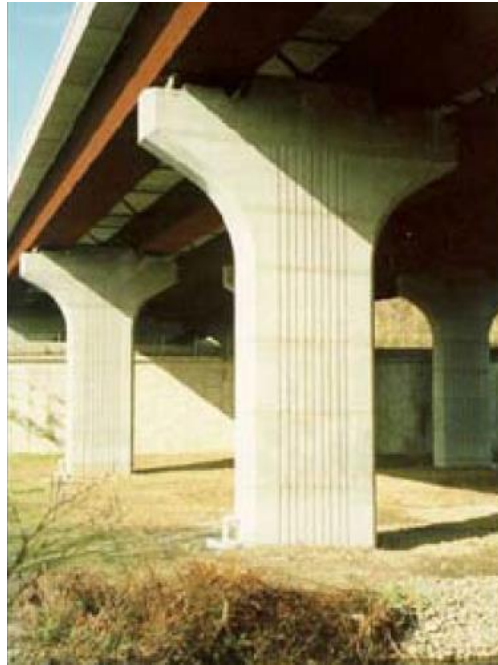
Figure 2-60: Pier after construction in Cross Westchester Expressway Viaduct (FHWA 2009)
