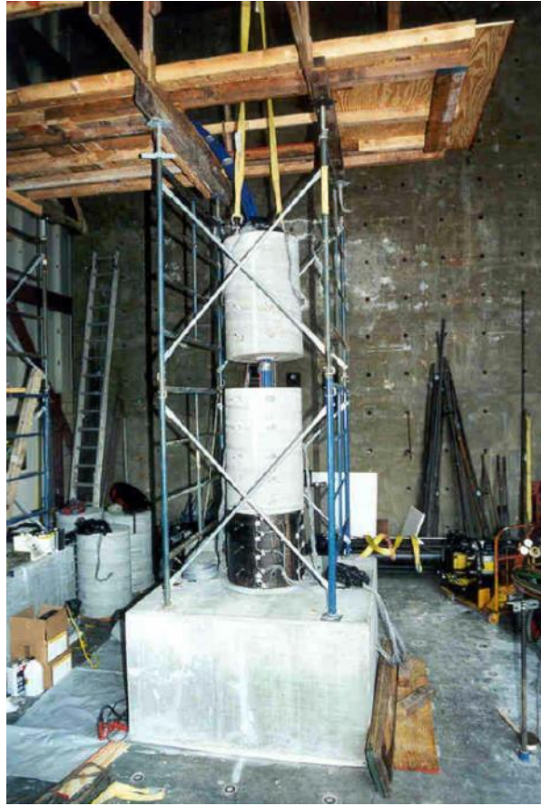
Figure 2-6: Construction of precast column tested by Hewes and Priestley (2002)
