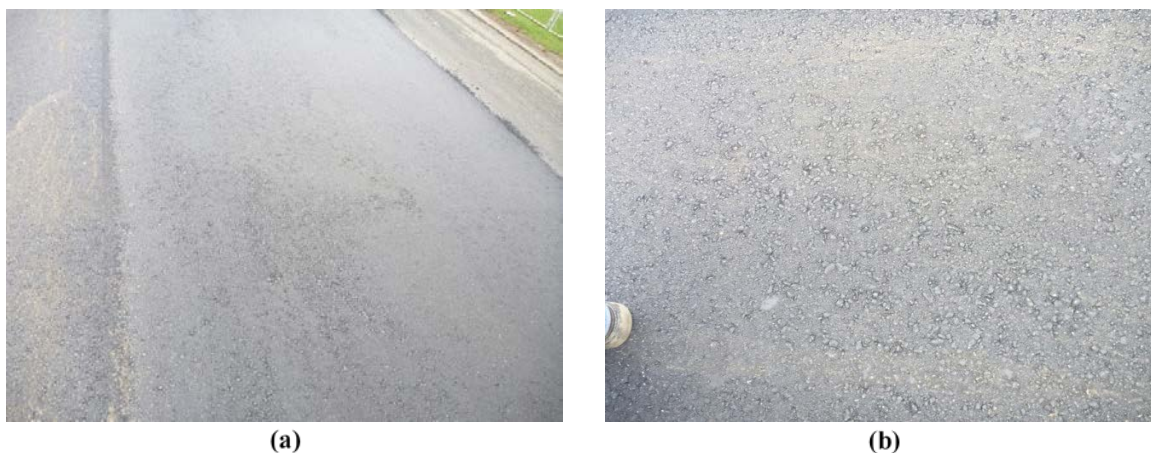
Figure 3. Example of Segregation Observed: (a) 30% RAP mixture; (b) 40% RAP mixture. RAP = reclaimed asphalt pavement.
