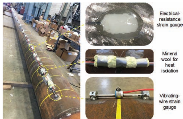
Figure 3.3 Instrumentation details of the closed-ended test pile. (Modified after Han, Ganju, Salgado, & Prezzi, in press b.)
