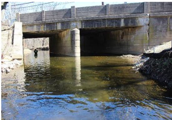
First On-Site Inspection
