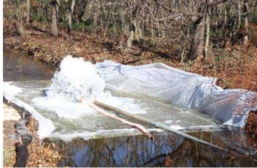
Photo 18 Downstream Energy Dissipater
