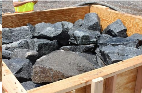
Photo 8 Final Rock Placement in the Form
