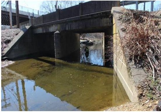
First On-Site Inspection
