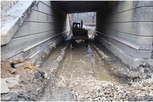
Photo 25 Placing AASHTO Number 1 Course Aggregate
