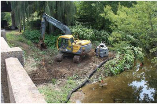
Photo 16 Upstream Construction Entrance
