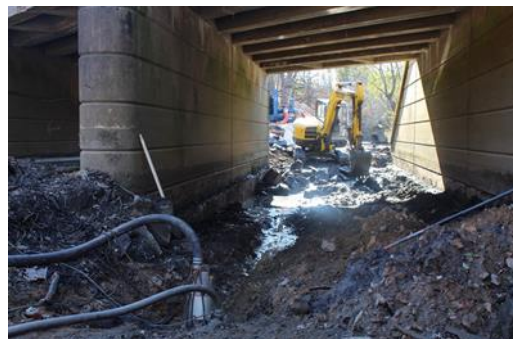
Photo 24 Removal of Existing Rocks in Span 1
