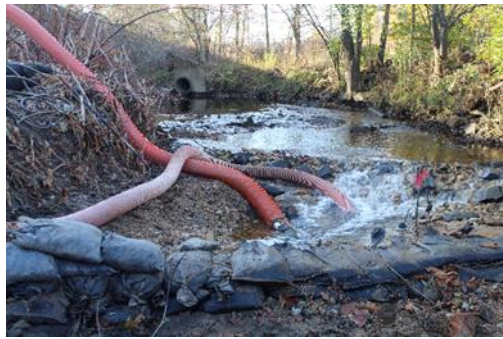
Photo 17a Upstream Cofferdam
