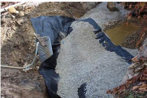
Photo 27 Placement of Combined Filter
