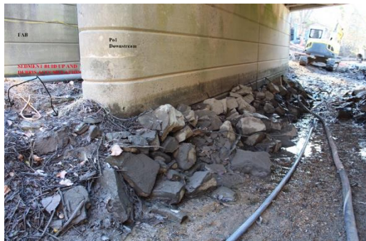
Photo 22 Preconstruction Condition of Span 1
