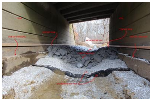
Photo 28 Placement of R6 Rocks on Top of Combined Filter
