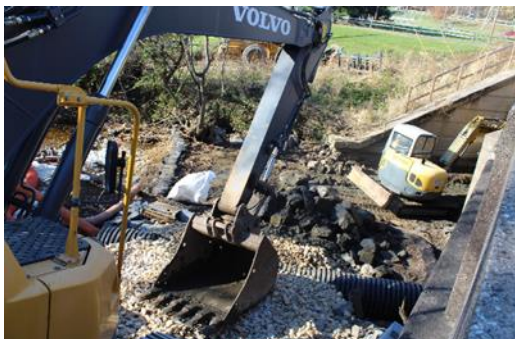
Photo 23 Large and Mini Track Excavators
