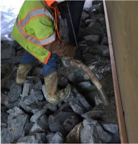
Photo 31 Grout Placement at Interface
