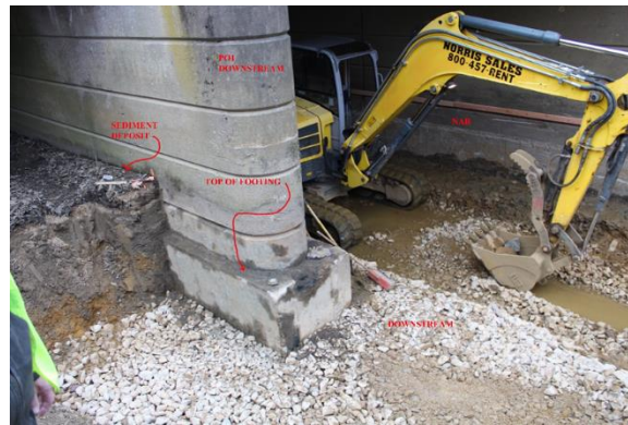
Photo 50 Cross-Section of the Streambed in Span 2
