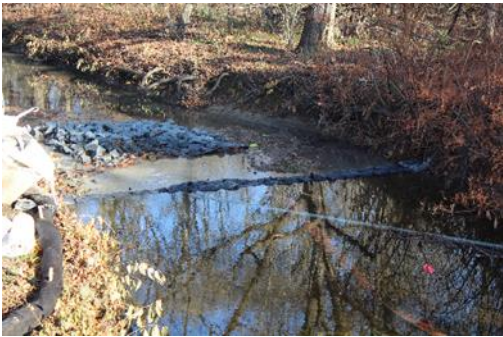
Photo 17b Downstream Cofferdam
