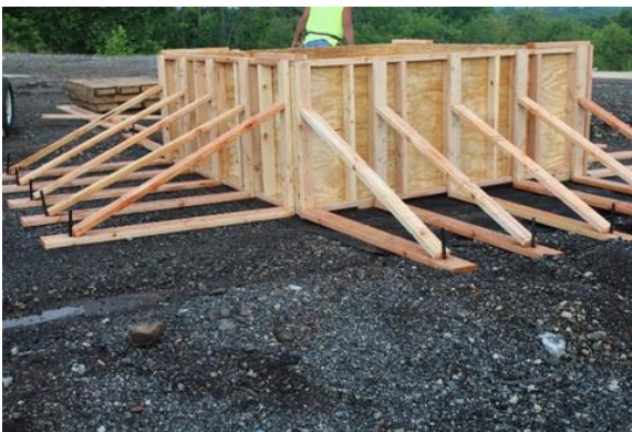
Photo 5 Test-Pit Form with Exterior Support
