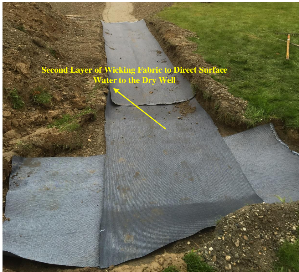
Figure 3.11 Second layer of H2Ri wicking fabric
