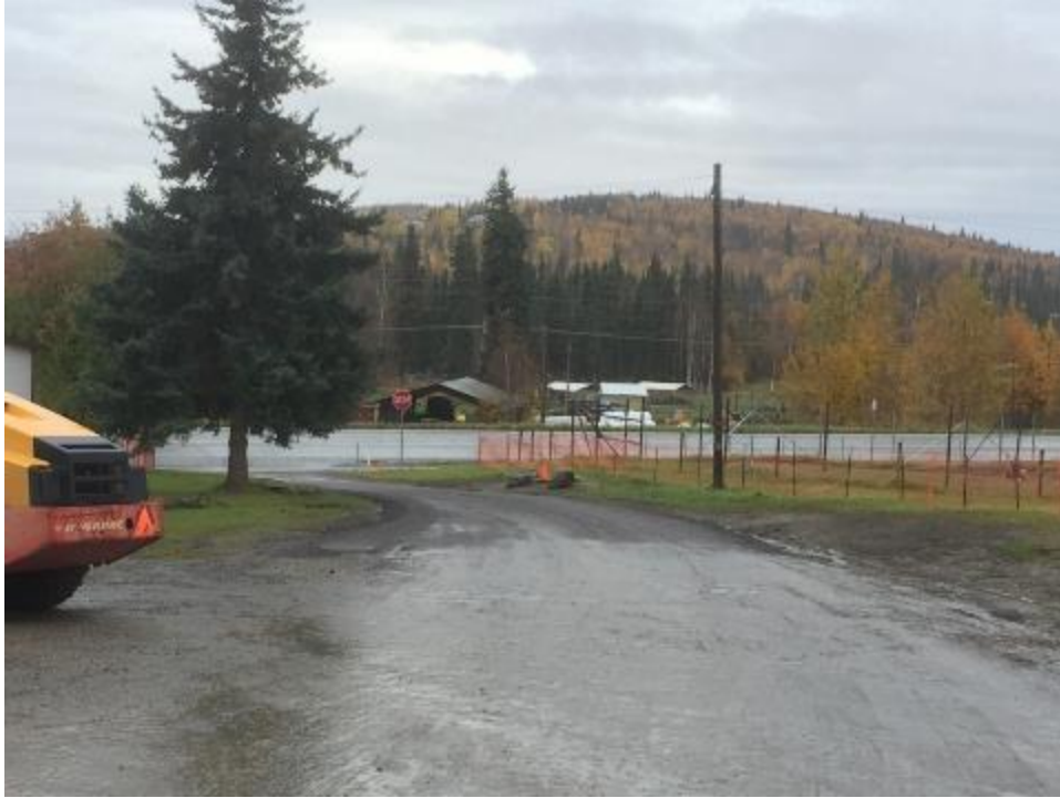
Figure 3.13 Road condition after rehabilitation
