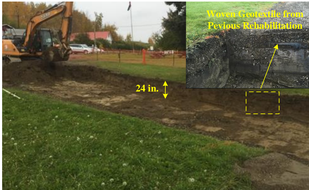
Figure 3.6 Excavation of the test section on the west side
