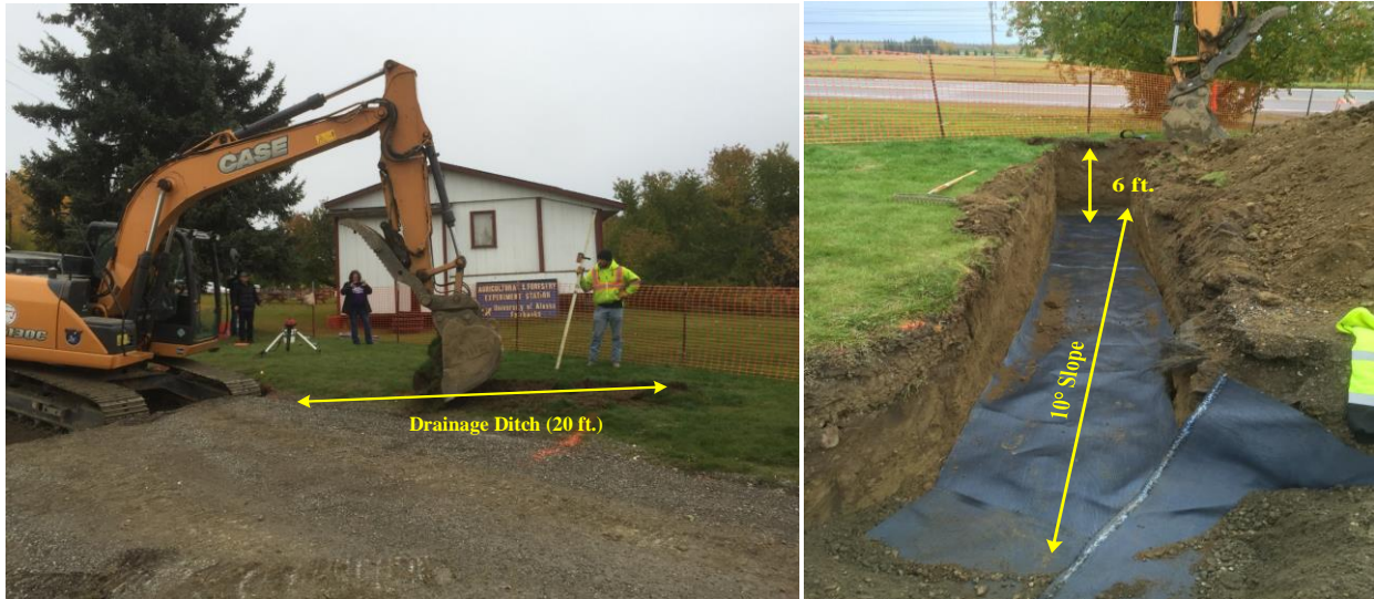
Figure 3.10 Excavation of drainage ditch
