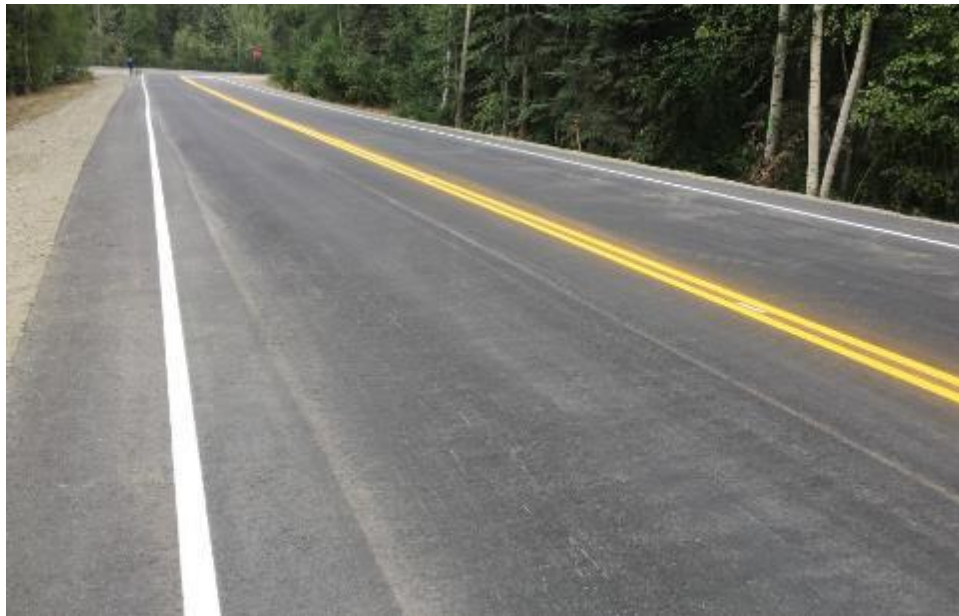
Figure 3.25 Road condition after rehabilitation
