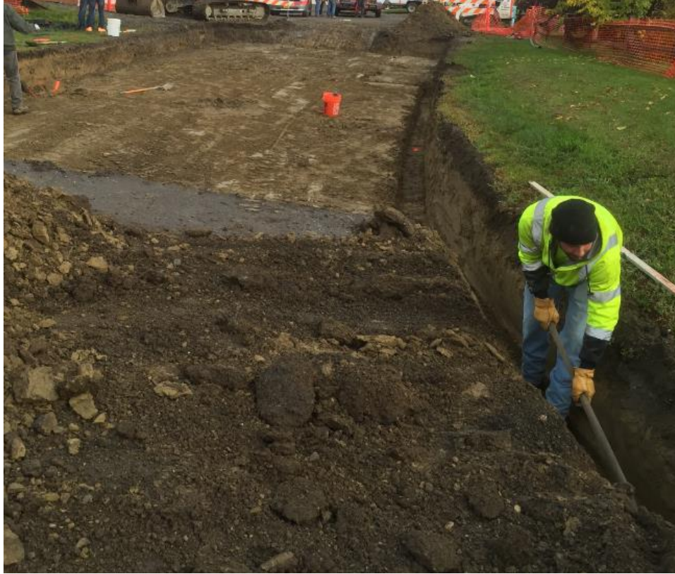
Figure 3.14 Excavation of drainage trench
