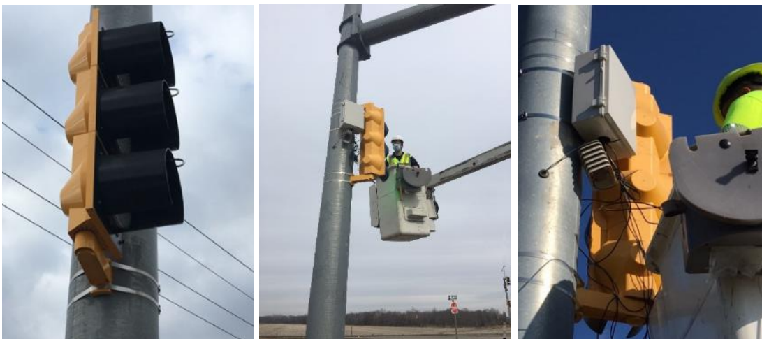
The installed new signals with a plastic weatherproof box for mounting the field monitoring system inside
