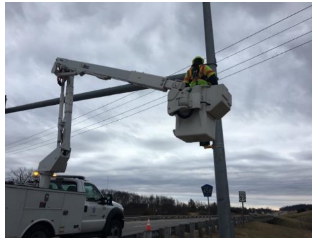
Remove the existing LED signals
