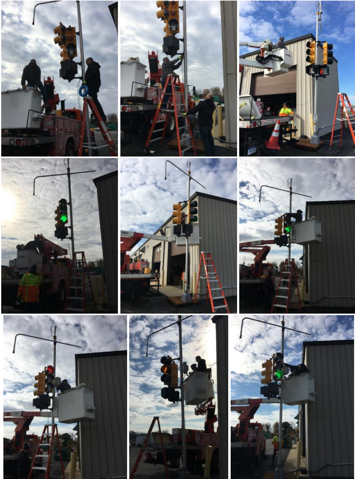
Figure 29: Field installation and setup of the onsite testing at the test site of Michigan in front of the signal shop, with the aid of the signal crew of Michigan DOT. A tunnel visor was installed with hook for mounting the cable camera on each signal module. The signals are facing north.
