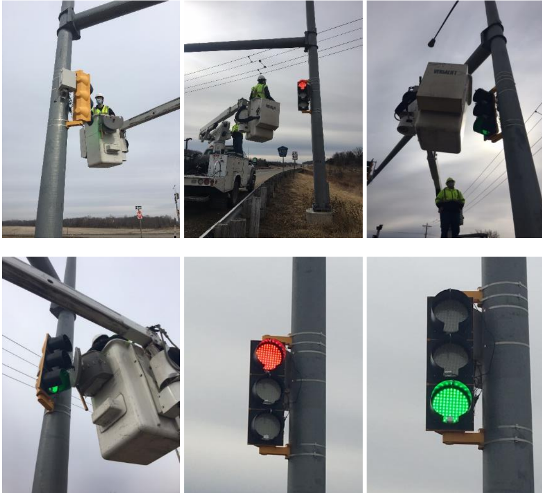
Figure 22: We stopped at the Lawrence field test site on Feb 25 th , 2021, with the Lawrence signal crew, to fix two problems related to the data collection and performance remote monitoring system (not part of the self-de-icing signal lights). We replaced the problematic cable cameras which failed after being exposed to the environment in the past two years, also fixed the loose mounting of the temperature sensors.
