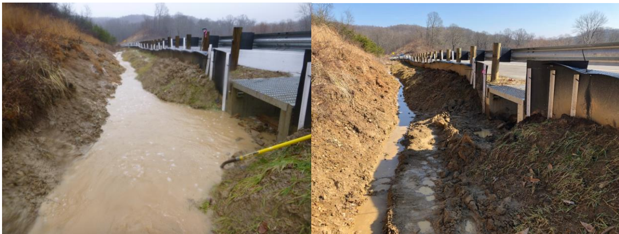
Figure A9-16. Flooding of ecopassage 3 in spring 2019 (left) and ecopassage 3 after an earthen dam was constructed to prevent further flooding (right) (ecopassages are labeled in Figure A9-2).
