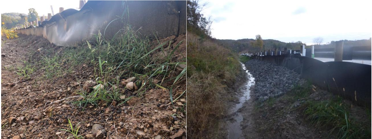
Figure A9-14. Area of erosion along fence before (left) and after (right) a rock bank was installed to reduce erosion.
