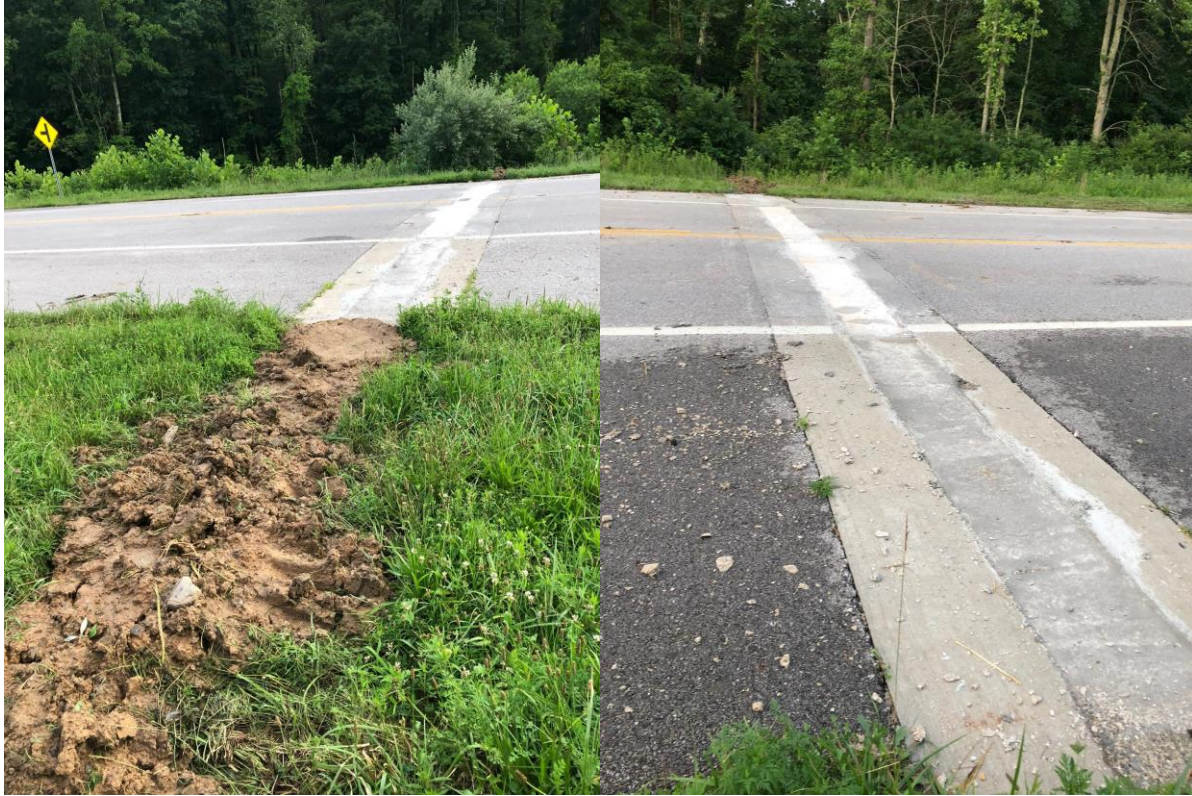
Figure A7-6. The 2013 ecopassages in place along State Route 78 near Nelsonville in Athens County, Ohio after they were filled in with concrete on June 27, 2019.
