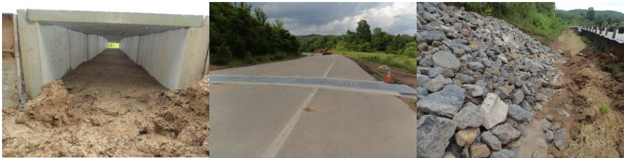
Figure A9-10. Ecopassage with layer of soil on the bottom (left), ecopassage with grated top in place (center), and rock bank and hay on biodegradable mesh used to prevent erosion (right).
