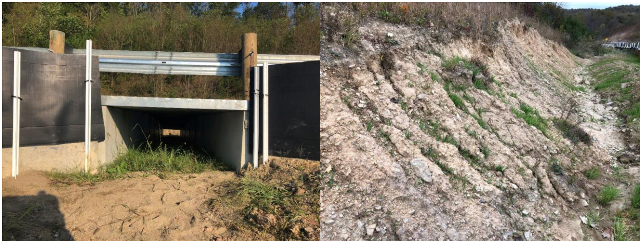
Figure A9-13. Barrier fencing attached to ecopassage headwalls (left) and grasses growing after the seeding of bare soils to reduce erosion (right).
