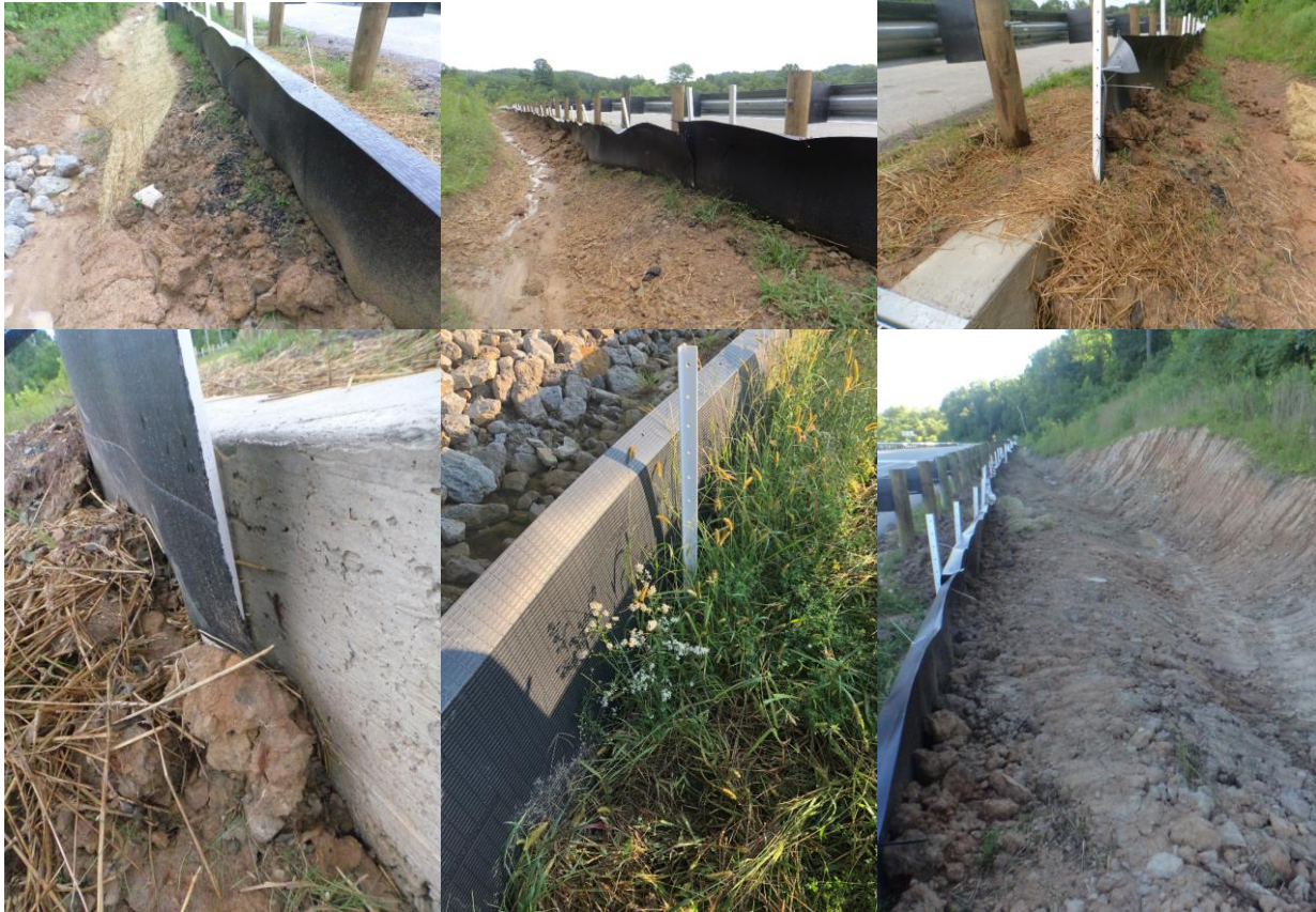
Figure A9-12. Ecopassage barrier fencing not buried in the ground (top left), barrier fencing top lip not folded properly (top center), barrier fencing not properly interfacing with the ecopassage headwall to prevent animal trespass (top right), bare headwall being climbed by a Red-spotted Newt (bottom left), barrier fencing not properly attached to fence post (bottom center), and steep ditch with no erosion control measures (bottom right).
