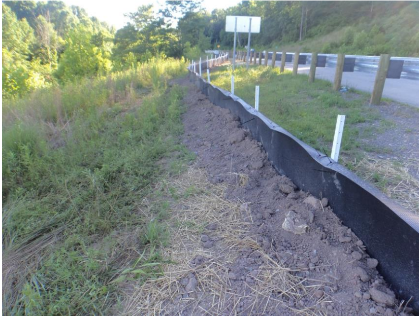
Figure A10-1. The 2018 barrier fencing angled toward ecopassages from the center on the east side of State Route 78 near Nelsonville in Athens County, Ohio.
