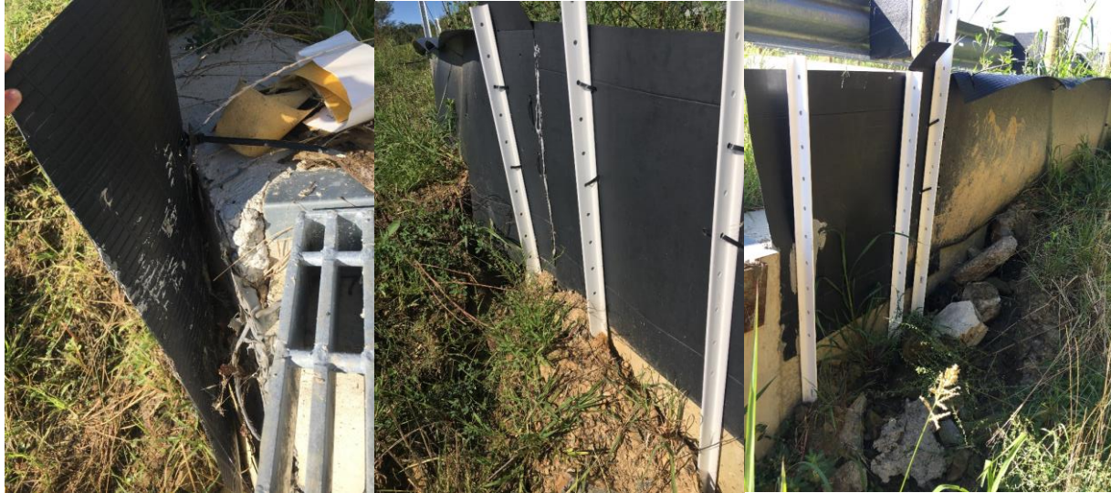
Figure A9-19. Area where fencing had separated from the headwall (left), area along a headwall where two pieces of fence had separated (center), and a persistent eroded area along the southwest headwall of ecopassage 5 (right) (ecopassages are labeled in Figure A9-2).
