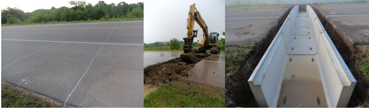
Figure A9-9. Roadway that has been painted and sawed through (left), excavated road cut (center), and concrete ecopassage placed into an excavated road cut (right).
