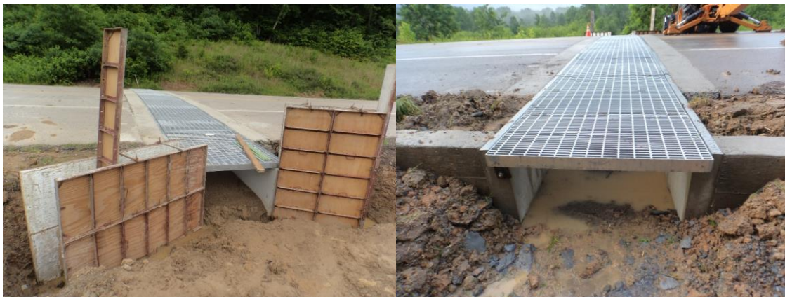
Figure A9-11. Ecopassage headwalls being created at an angle on the east side of the road (left) and completed headwalls that are straight on the west side of the road (right).
