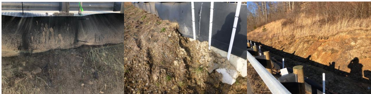
Figure A9-15. Area of erosion along barrier fence (left), area of erosion near an ecopassage headwall (center), and erosion on hillside (right) all after rains in spring 2019.
