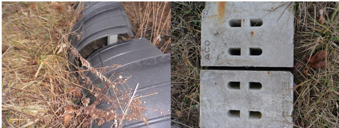
Figure A7-5. Maintenance concerns of the 2013 barrier-ecopassage system in place along State Route 78 near Nelsonville in Athens County, Ohio. Gaps and cracks in the plastic barrier fencing (left) and separation of concrete blocks that make up the ecopassages (right).
