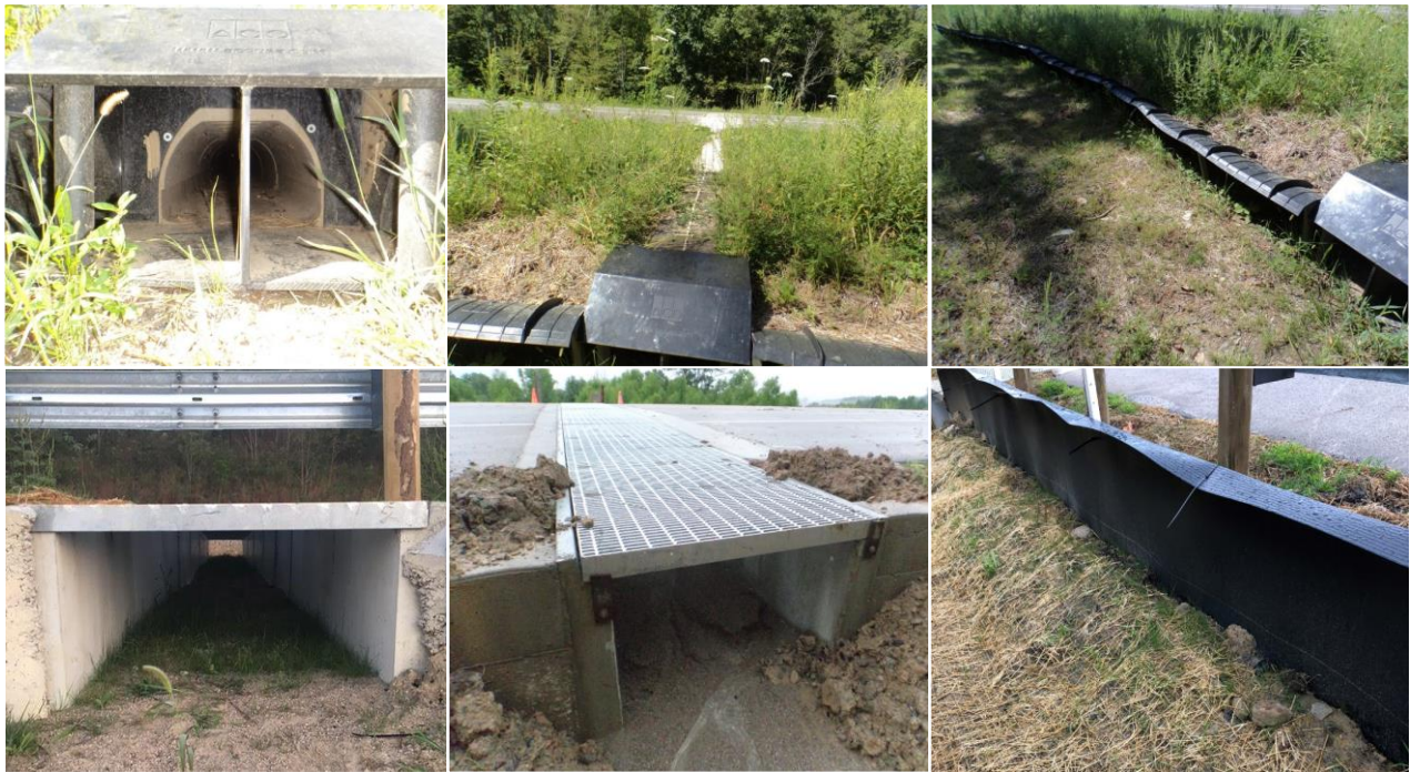
Figure 3. Images of the 2013 and 2018 barrier-ecopassage systems in place along State Route 78 near Nelsonville in Athens County, Ohio. Entrance view of a 2013 barrier-ecopassage system ecopassage (top left); 2013 ecopassage crossing the road (top center); 2013 barrier fence (top right). Entrance view of a 2018 barrier-ecopassage system ecopassage (bottom left); ecopassage crossing the road (bottom center); 2018 barrier fence (bottom right).
