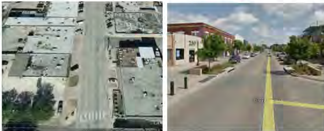
Figure 8 – Lower Greenville Avenue road diet – before left , after right
