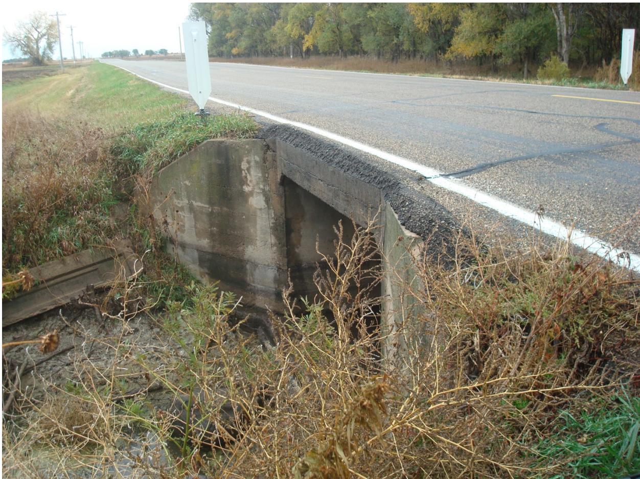
Figure 5.5 Culvert on 395 th Avenue three Miles North of SD Hwy 46
