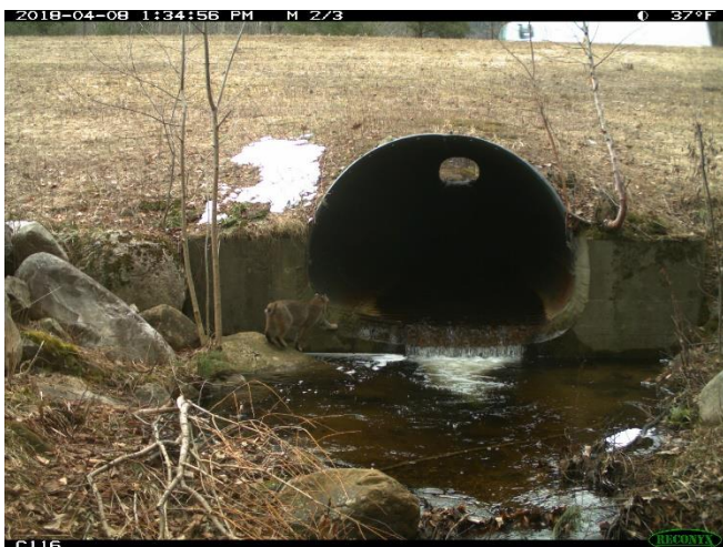
Bobcat at squash pipe 7-19-5, Sunderland
