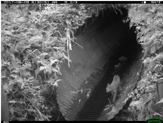
Bobcat moving through pipe culvert 16-13, Glover
