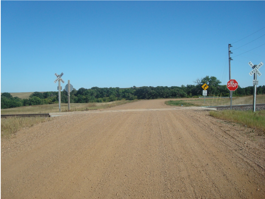
Figure 5.7 BIA 44 at Railroad Crossing (MP 9.4)
