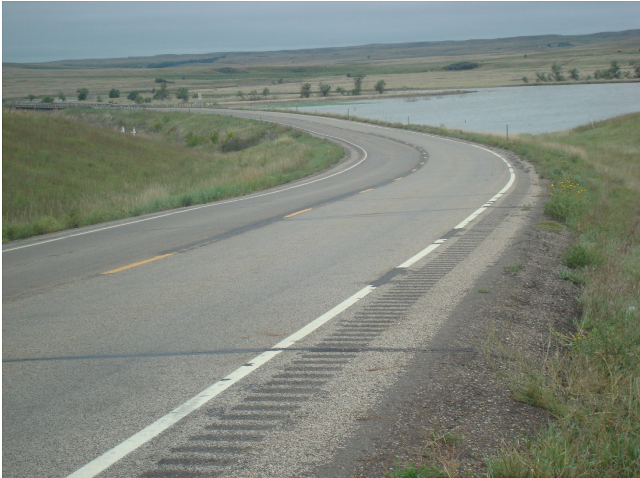
Figure 5.3 ND Highway 24 Curve at Bridge (MP 14 to MP 15)
