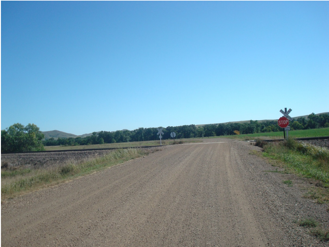
Figure 5.6 BIA 44 at Railroad Crossing (MP 2.5)
