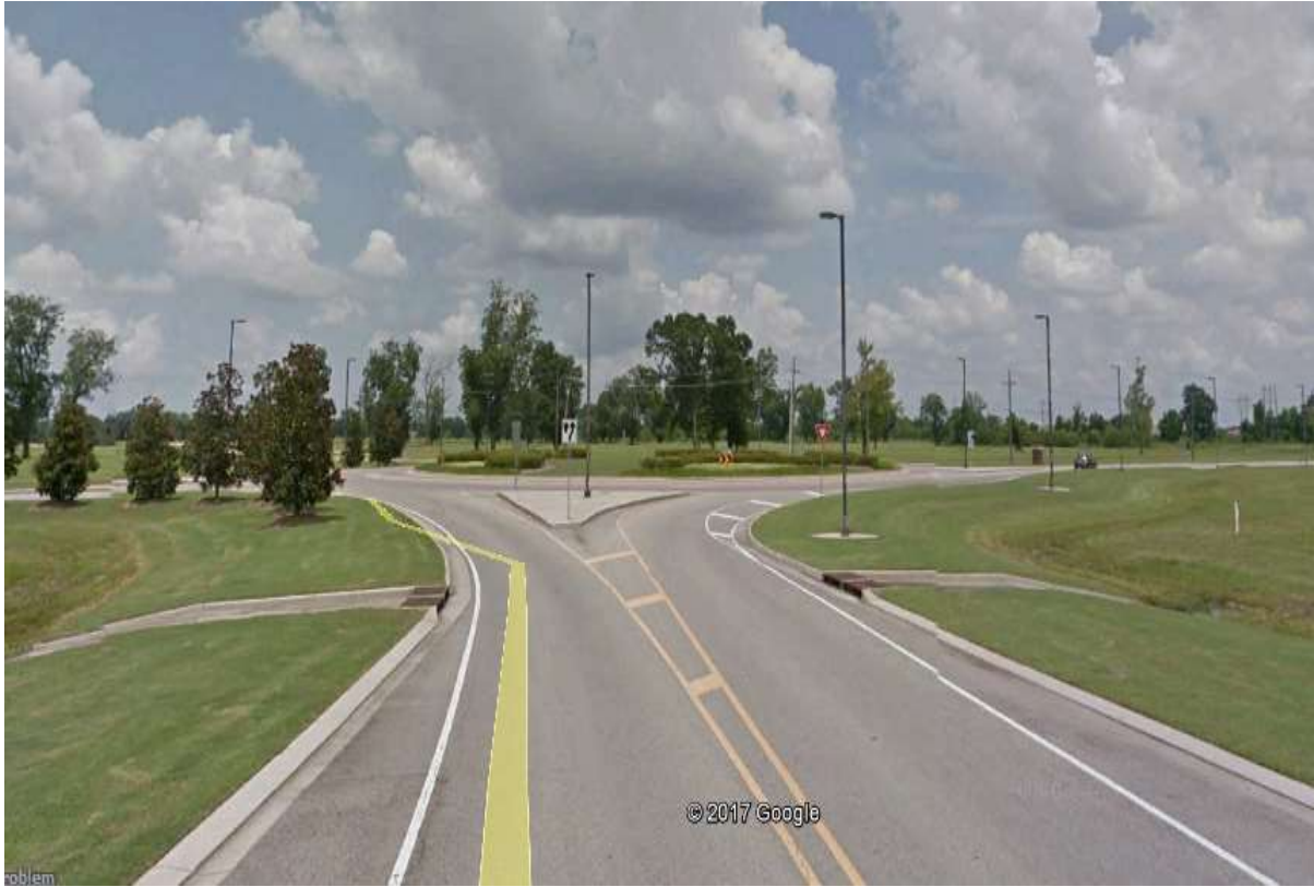
Figure E11.2 Traffic light condition in LA 327/ River Rd. at LA 327/ Gardere Rd. roundabout
