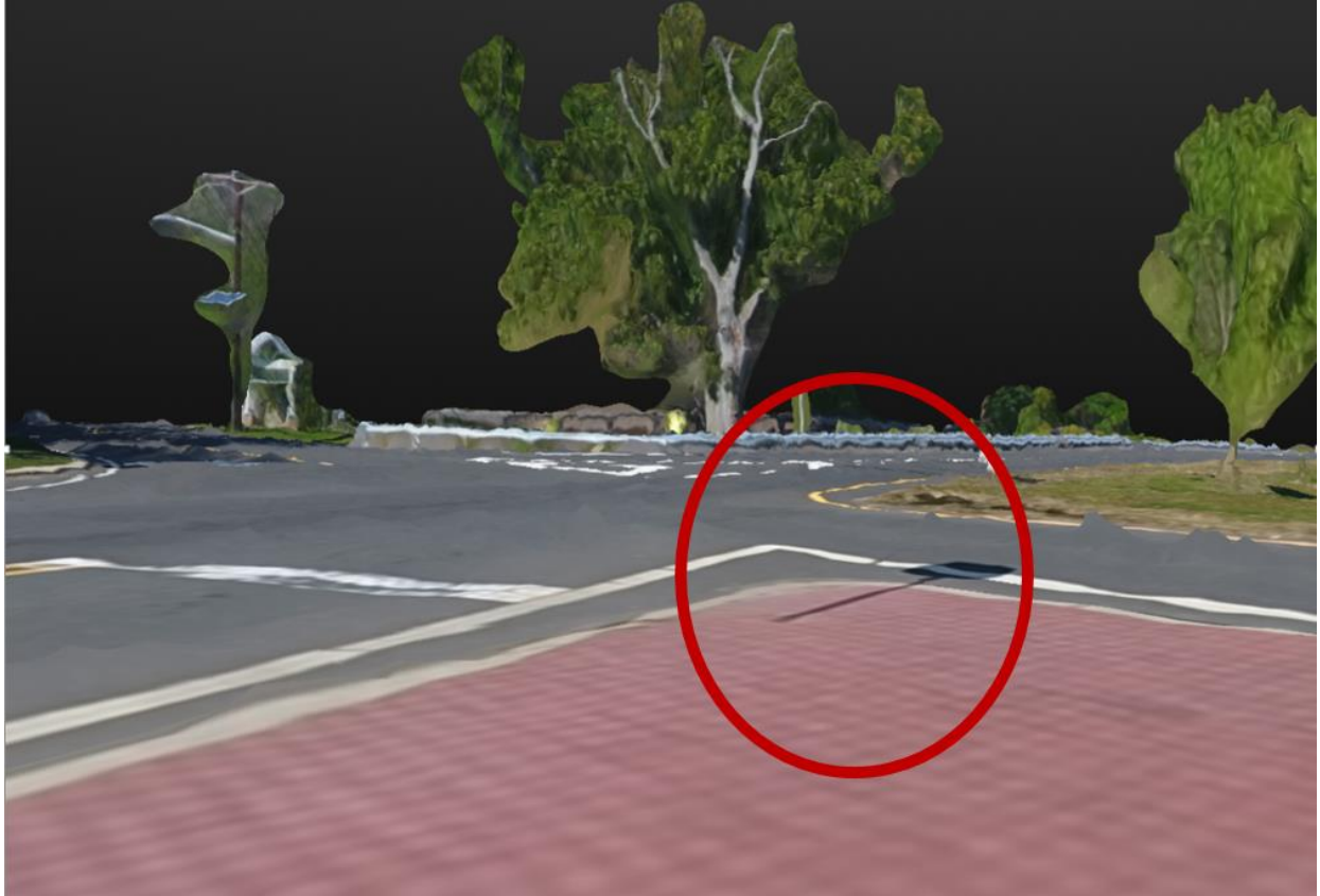
Figure 20: Missing Signage and Noise
