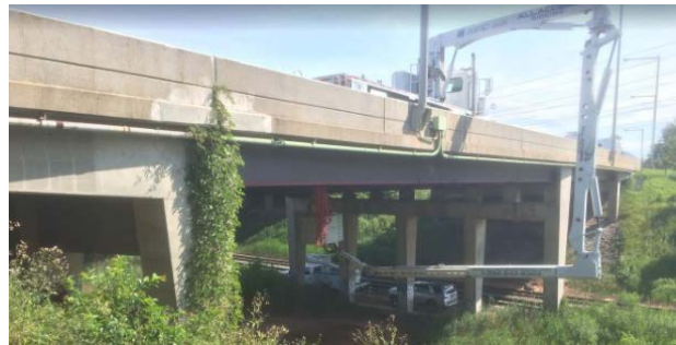
Figure 4: Elevation View During Underside Strain Gauge Installation
