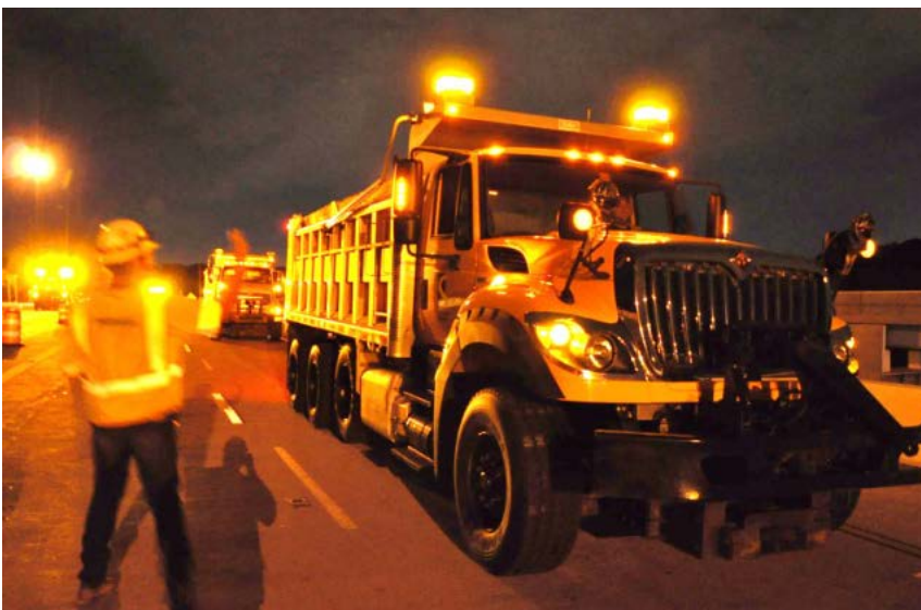
Figure 12: Truck staging during load test
