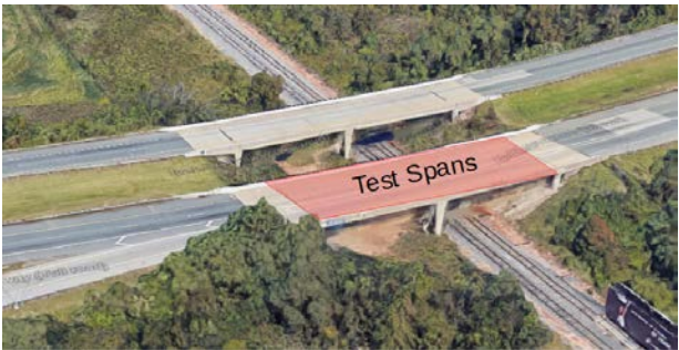
Figure 3: Overview of Selected Bridge
