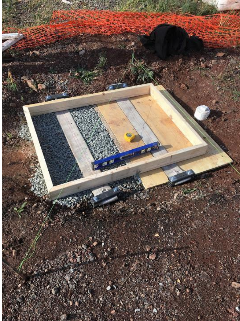
Figure 162: Layout of slab molds prior to geo-textile fabric
