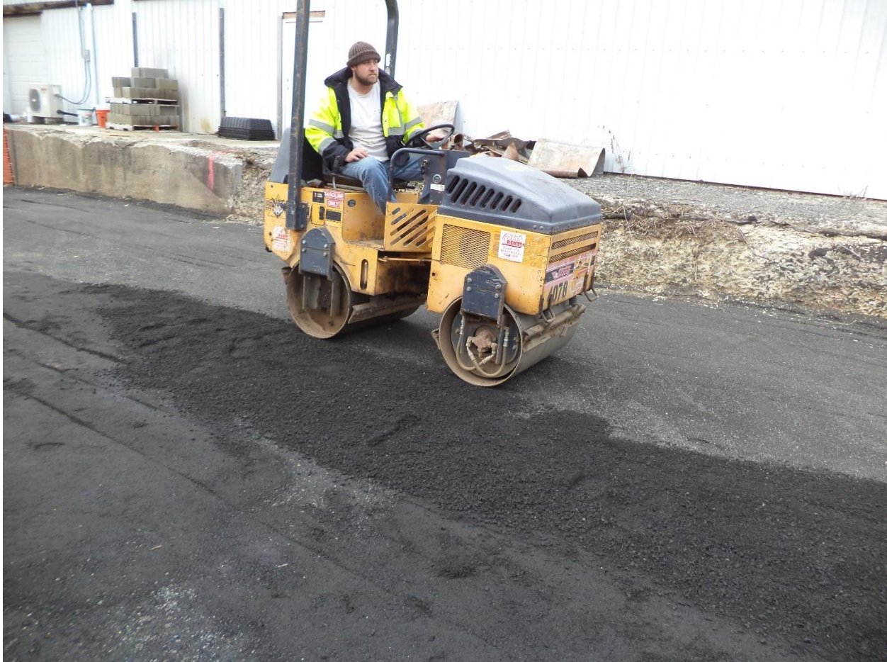
Figure 7: Rolling the base surface to ensure a stable surface to place the test specimens
