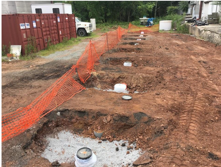
Figure 154: Prepared subgrades for drainage with footing tubes exposed
