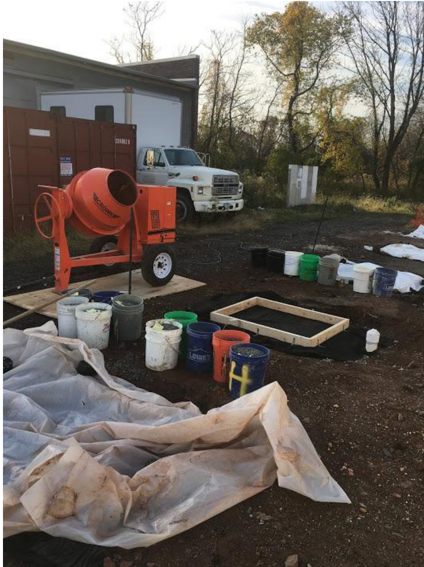
Figure 165: Aggregate, water, admixtures and tools prepared to mix concrete slabs
