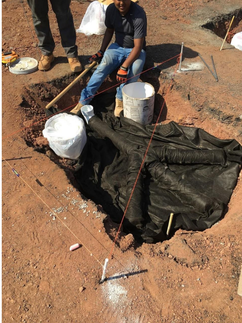
Figure 156: Non-woven geotextile fabric covering drainage pipe
