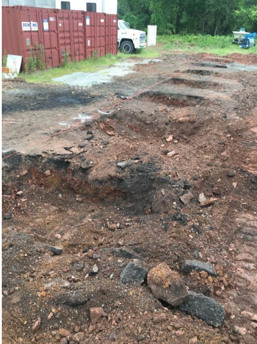
Figure 149: Rough foundations for pervious test samples, looking ESE
