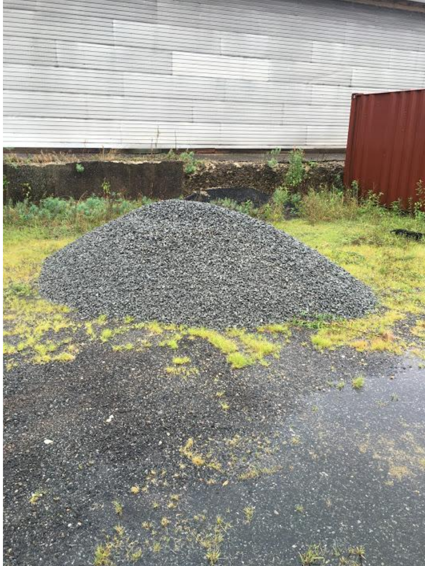
Figure 157: Stockpile of 3/4in (19mm) aggregate
