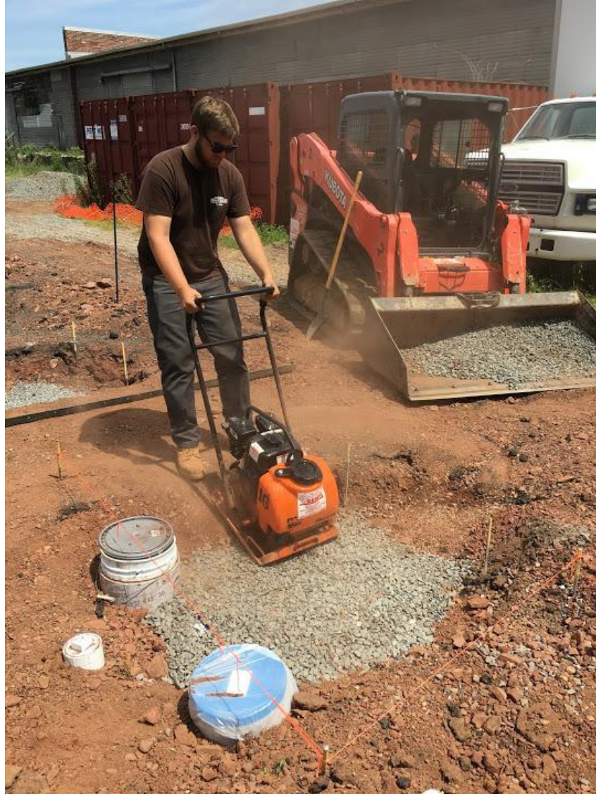
Figure 158: Placing and compacting base course aggregate
