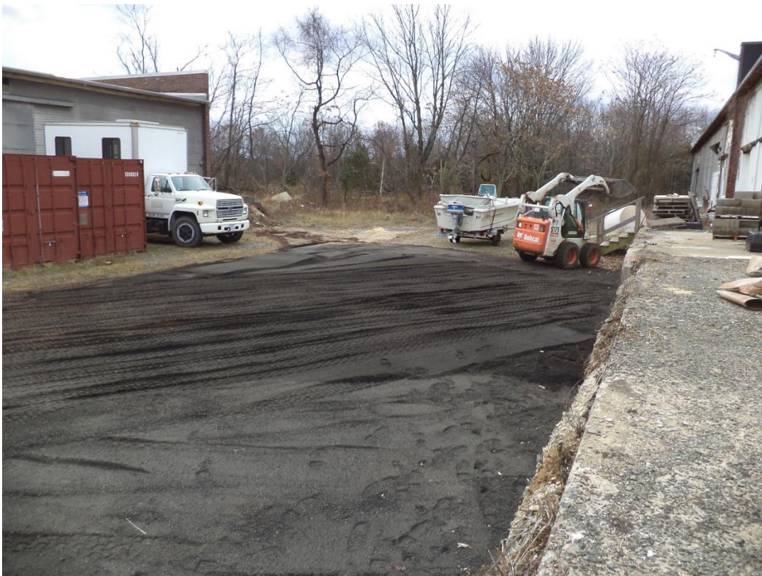
Figure 6: Back scraping the RAP base to prepare for rolling the surface with a vibratory drum roller
