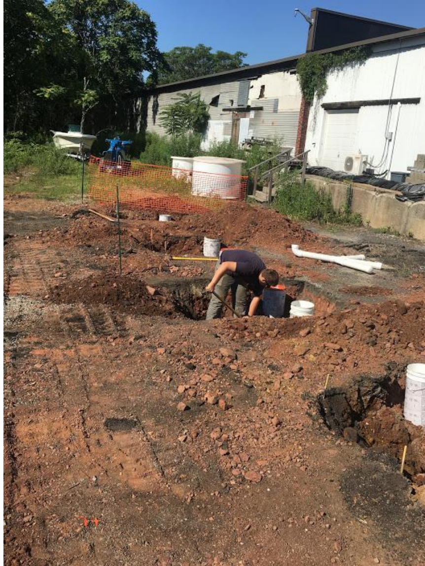
Figure 153: Footing tubes in place inside rough foundations
