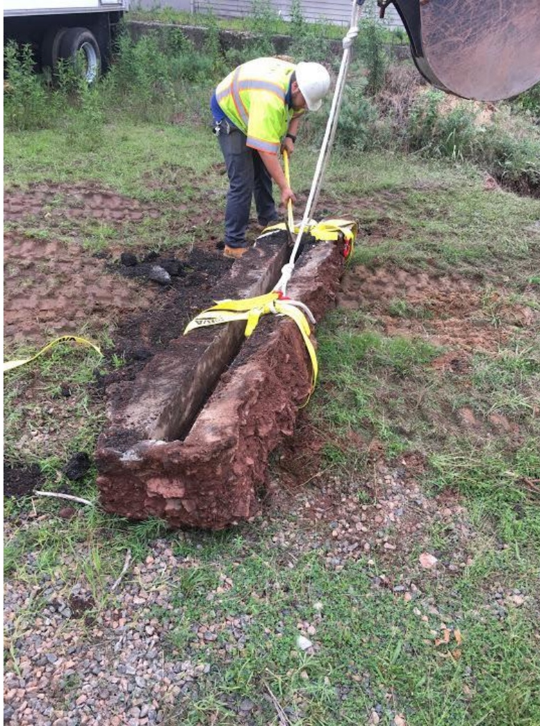
Figure 147: Preparing to move wall footing
