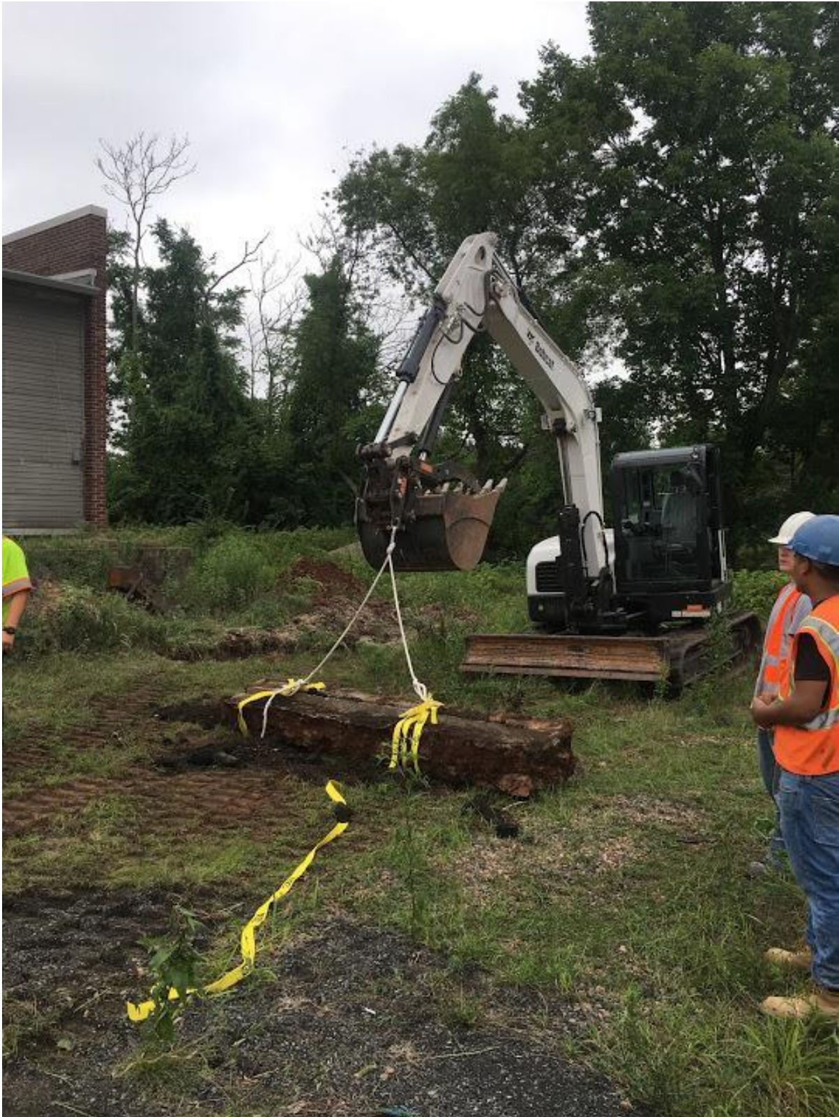
Figure 148: Moving the footing with the E85 Excavator
