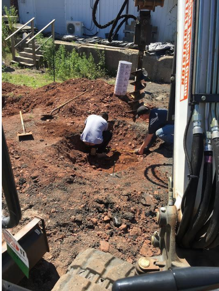
Figure 152: Auger attachment on Bobcat E50
