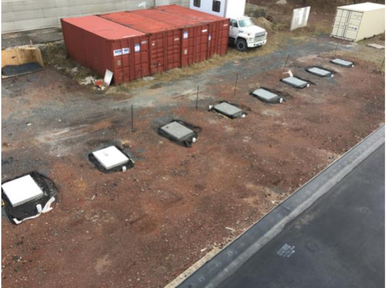
Figure 172: Final layout of field slabs after curing procedure and prior to backfilling
