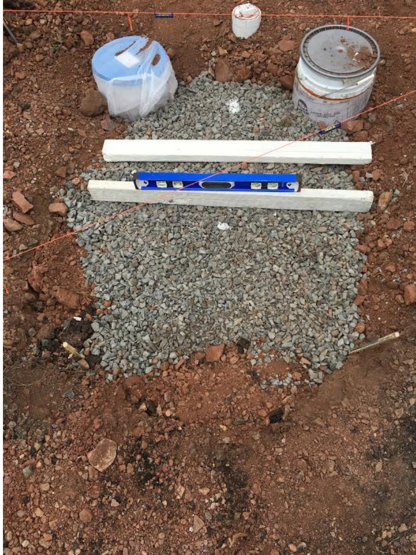
Figure 159: Leveling the base course
