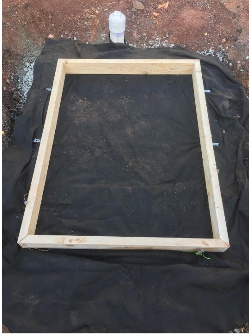
Figure 164: Final layout of concrete molds prior to pouring
