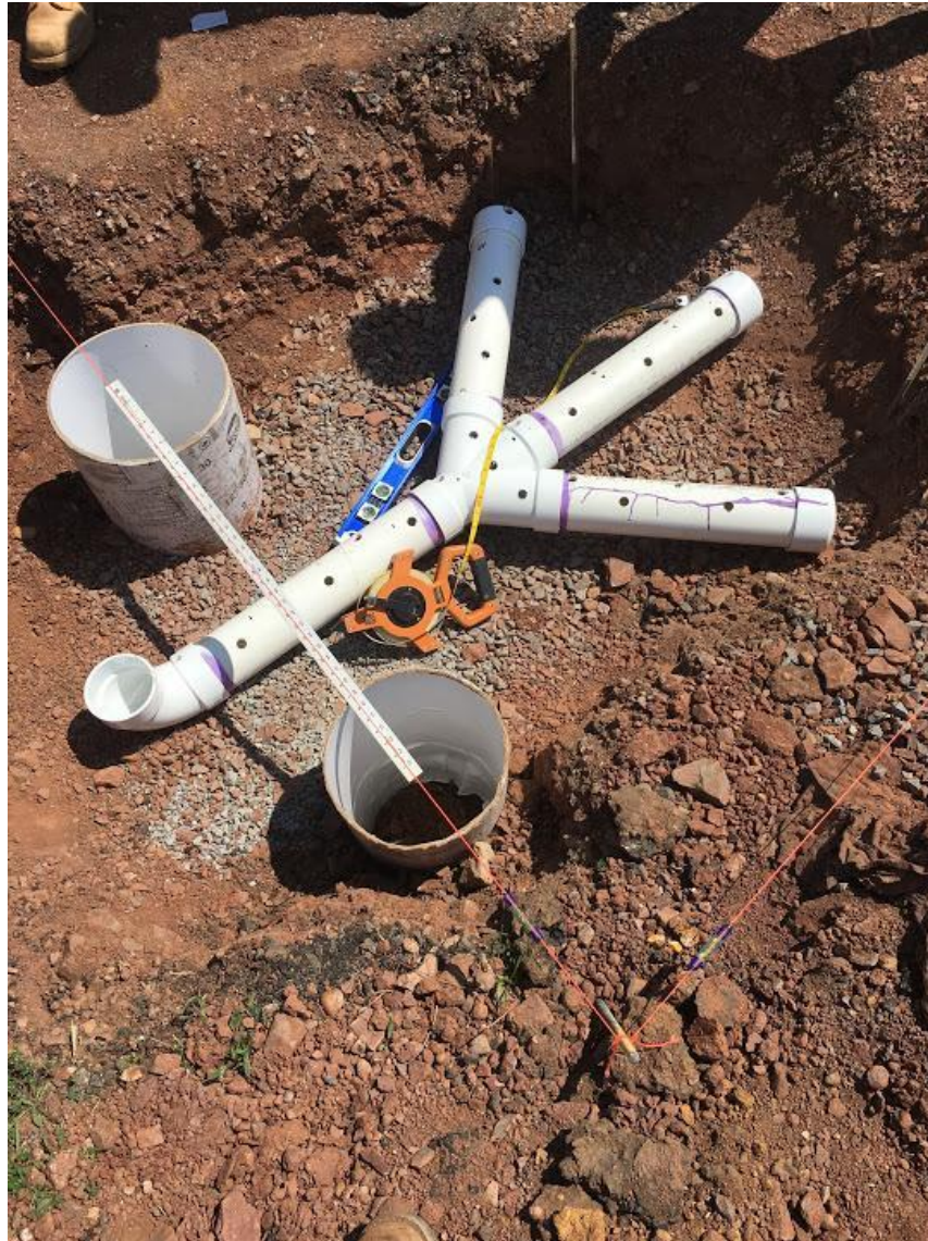
Figure 155: Drainage Pipe with Wyle 'Y'
