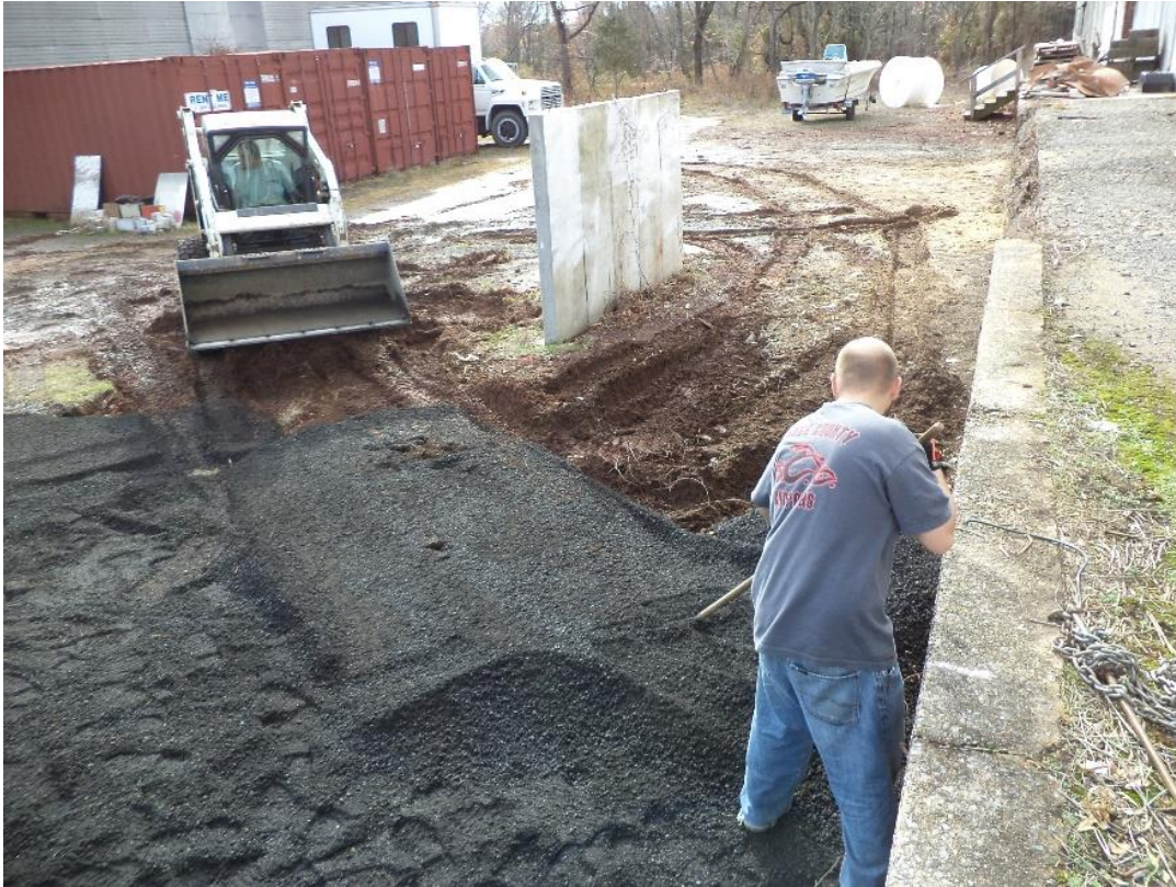
Figure 5: Preparing the testing surface by spreading Reclaimed Asphalt Pavement (RAP) to normalize the reflective surfaces
