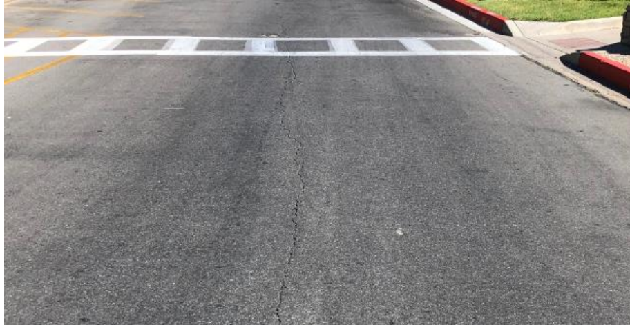
Figure 2-4. Longitudinal Crack
