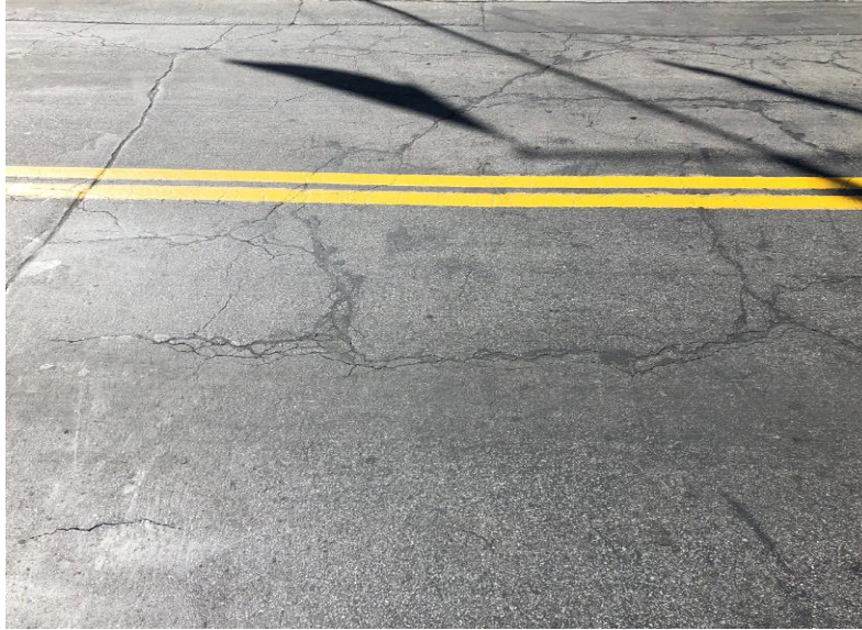
Figure 2-3. Block Crack
