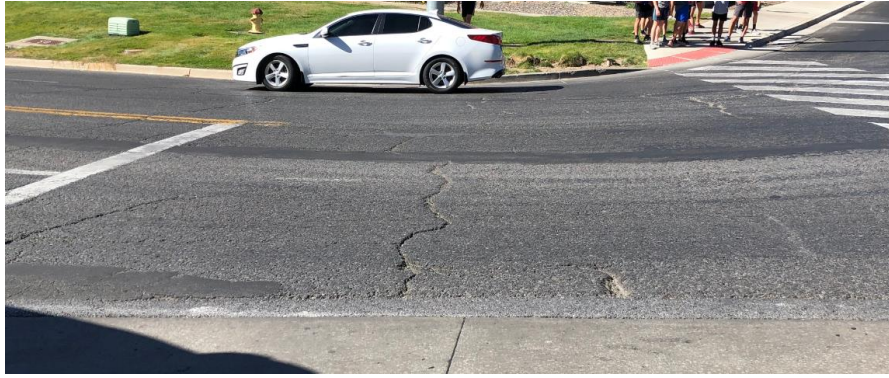
Figure 2-2. Transverse Crack
