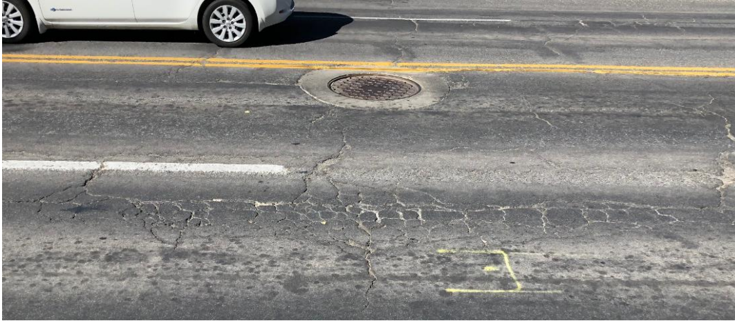
Figure 2-5. Wheel-Path Crack
