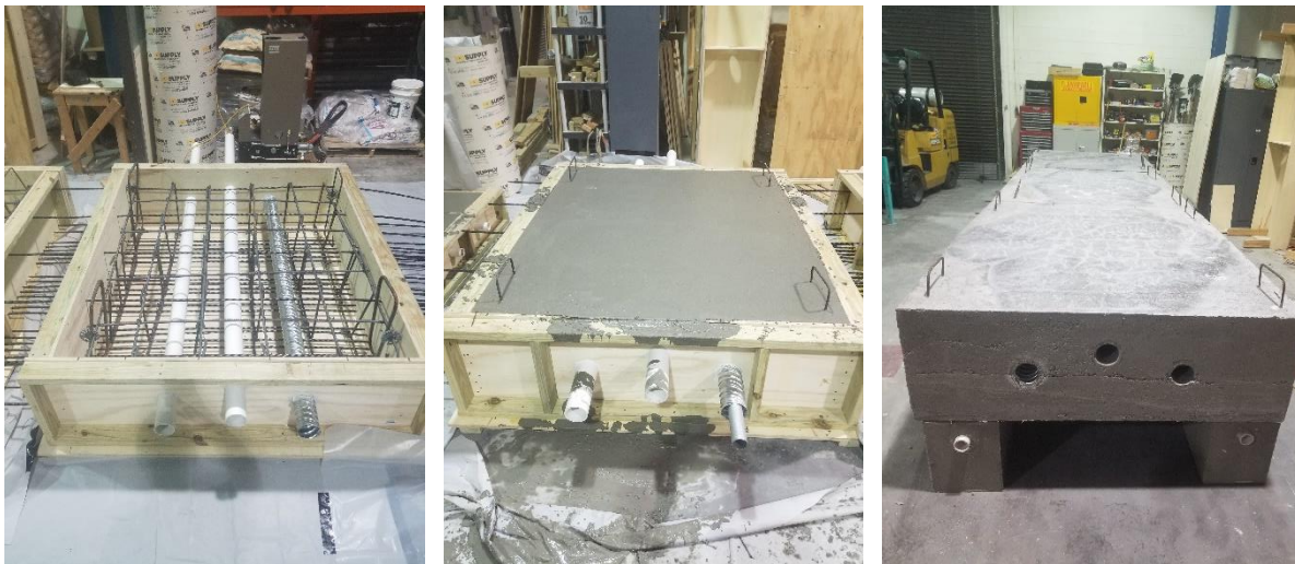
Figure 4-28: Construction of specimen.
