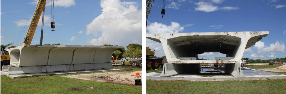
Figure A-7: Decommissioned box girder segments at FIU.
