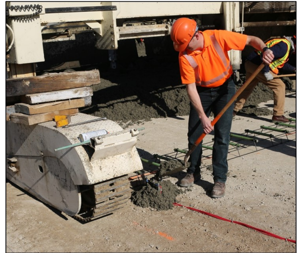
Placing concrete around sensors
