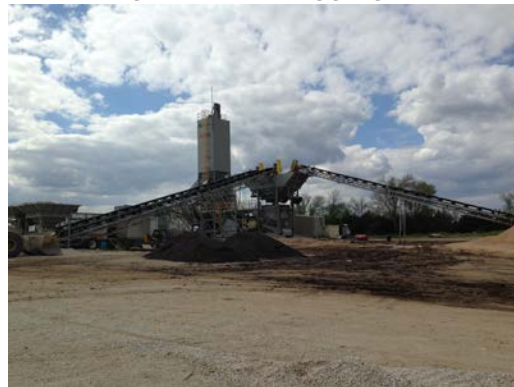
Figure 6: Light Weight Aggregate Stockpile
