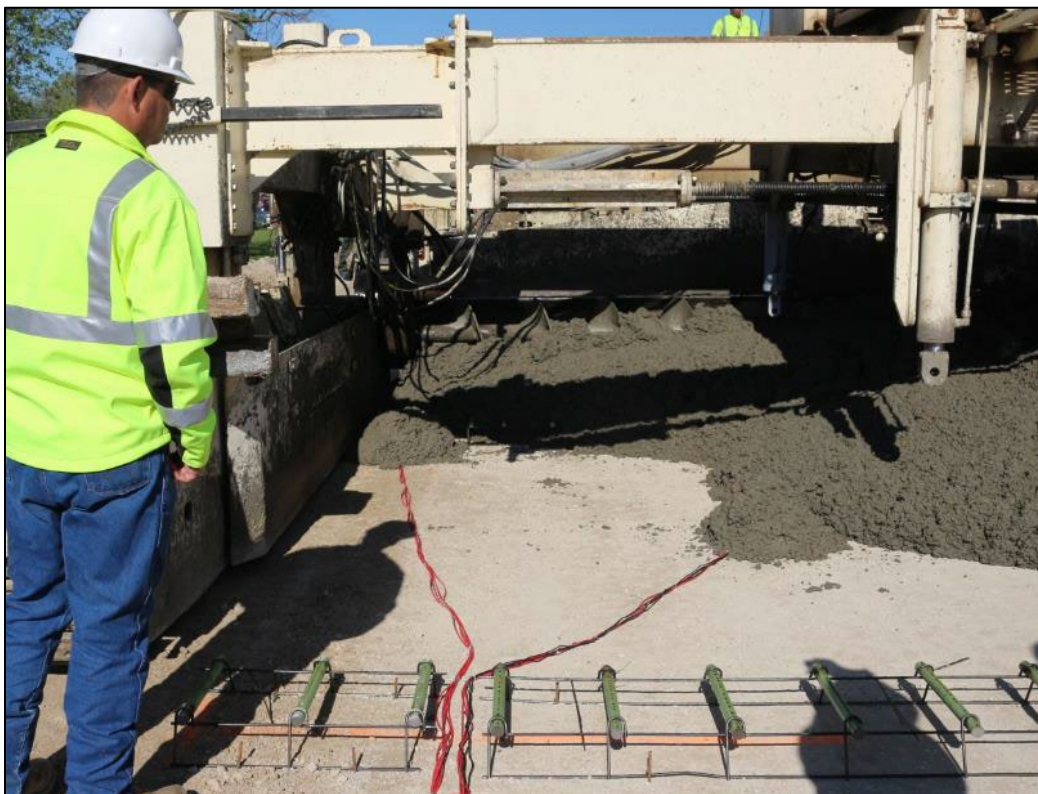
Figure 3.9: Concrete Laydown Machine Approaching Sensors
