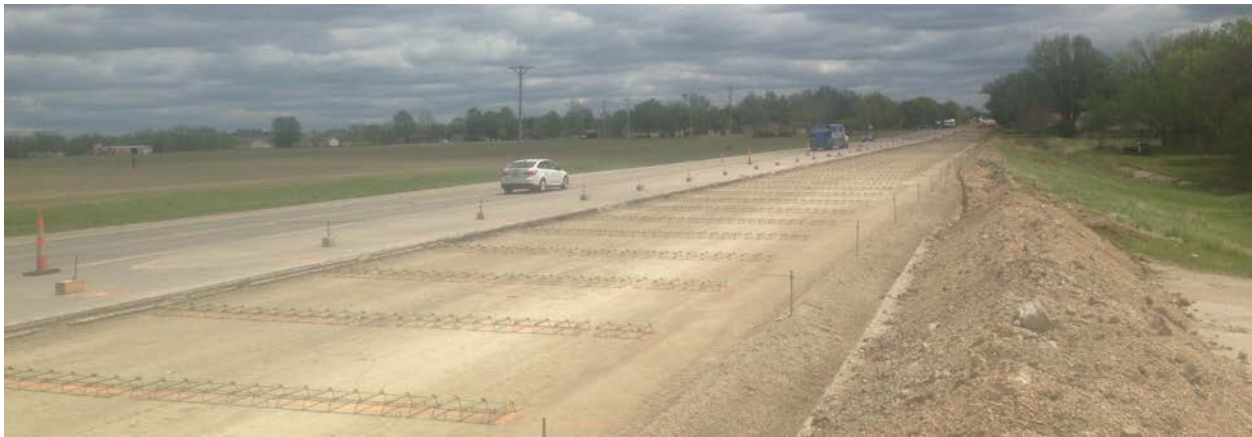
Figure 1: A view of the US-54 Reconstruction Section
