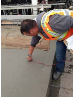
Figure 23: Maturity meter Instrumented in the Pavement
