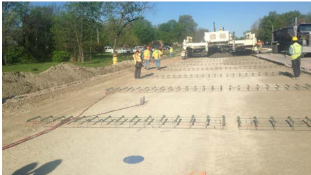
Figure 40: Metal Target placed on top of the base
