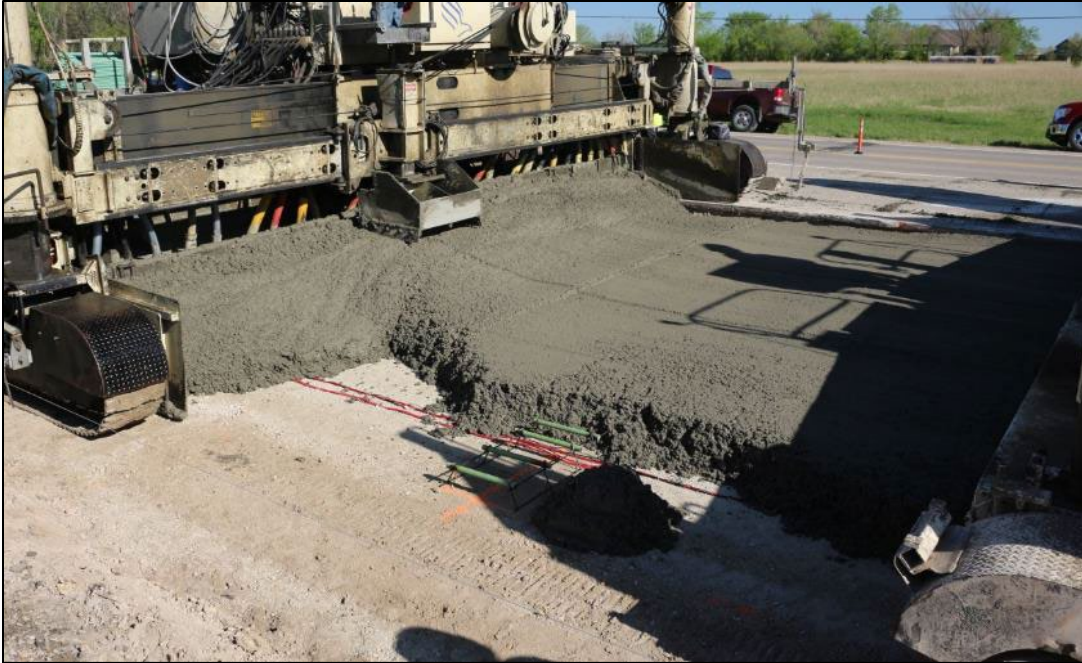
Figure 3.10: Sensors Between Laydown Machine and Finish Paver
