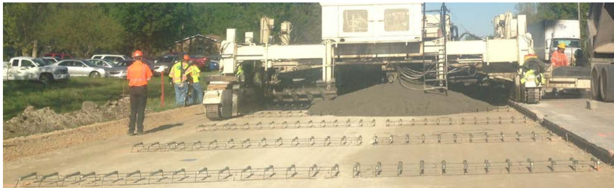
Figure 34: Dowels placed using Dowel Baskets
