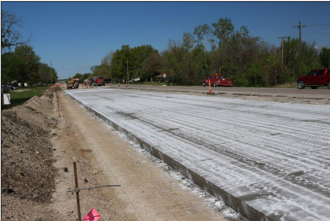
Figure 3.11: Initial Application of White Pigmented Curing Compound
