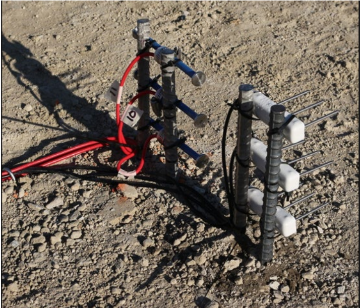
Figure 3.4: Moisture Sensors and Strain Gages in Center of Panel
