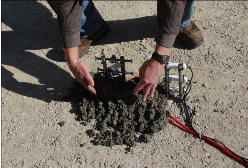
Figure 3.8: Packing Concrete Around Sensors to Ensure Proper Compaction
