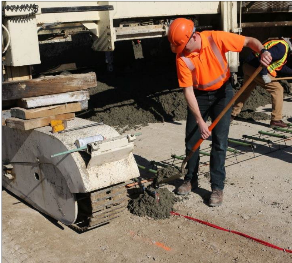
Figure 3.7: Placing Concrete Around Sensors
