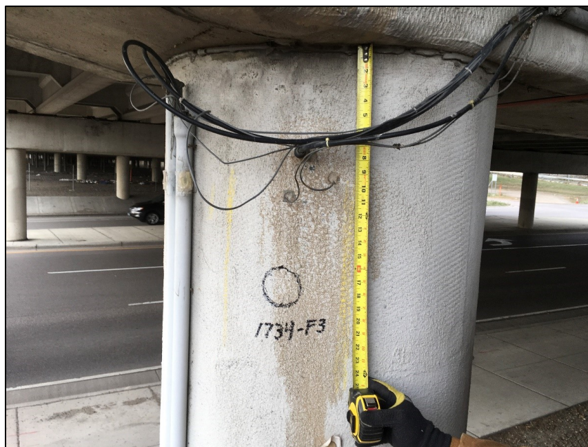
Figure 2.20 View of the instrumentation installed at Column 34F-3.
