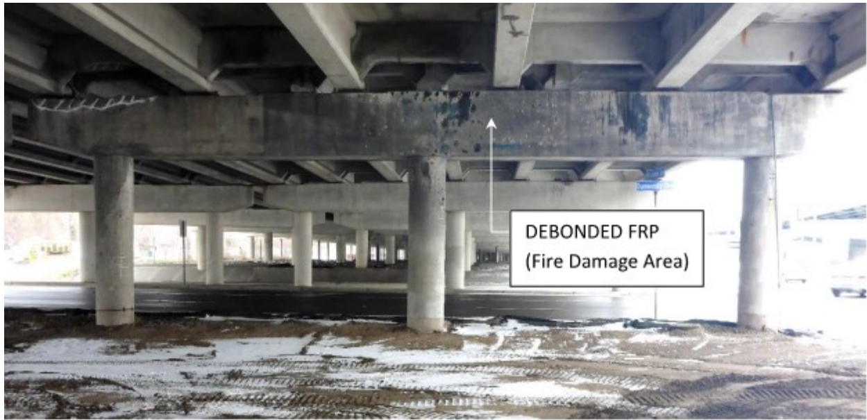
Figure 3.4 Pier 34WB - East Face
