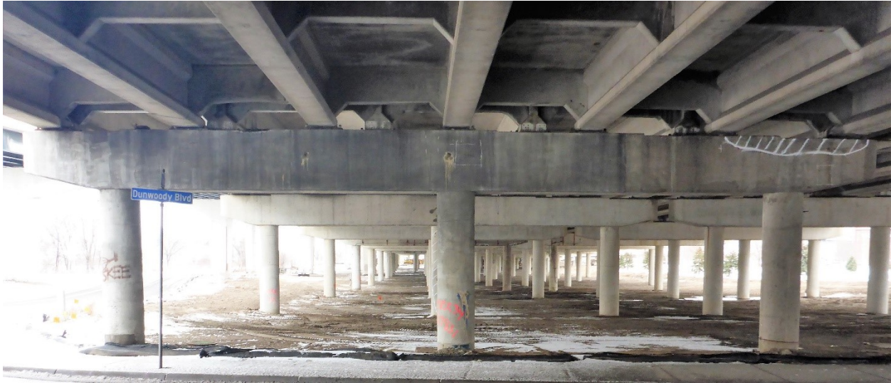
Figure 3.2 Pier 34WB - West Face
