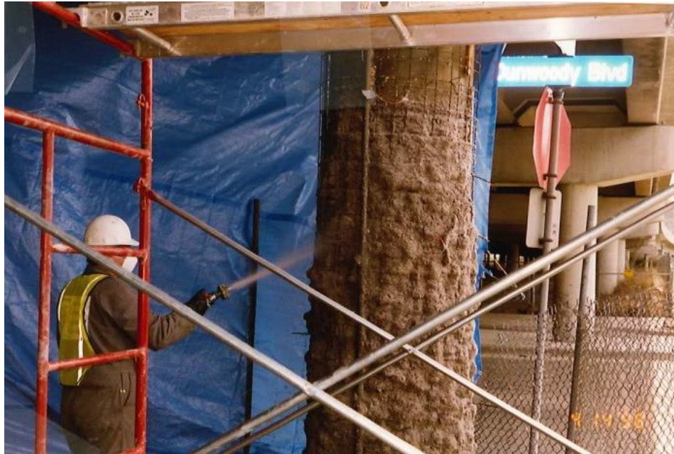
Figure 2.14 Pier 34WB - ECE installation in progress, during application of cellulose fiber
