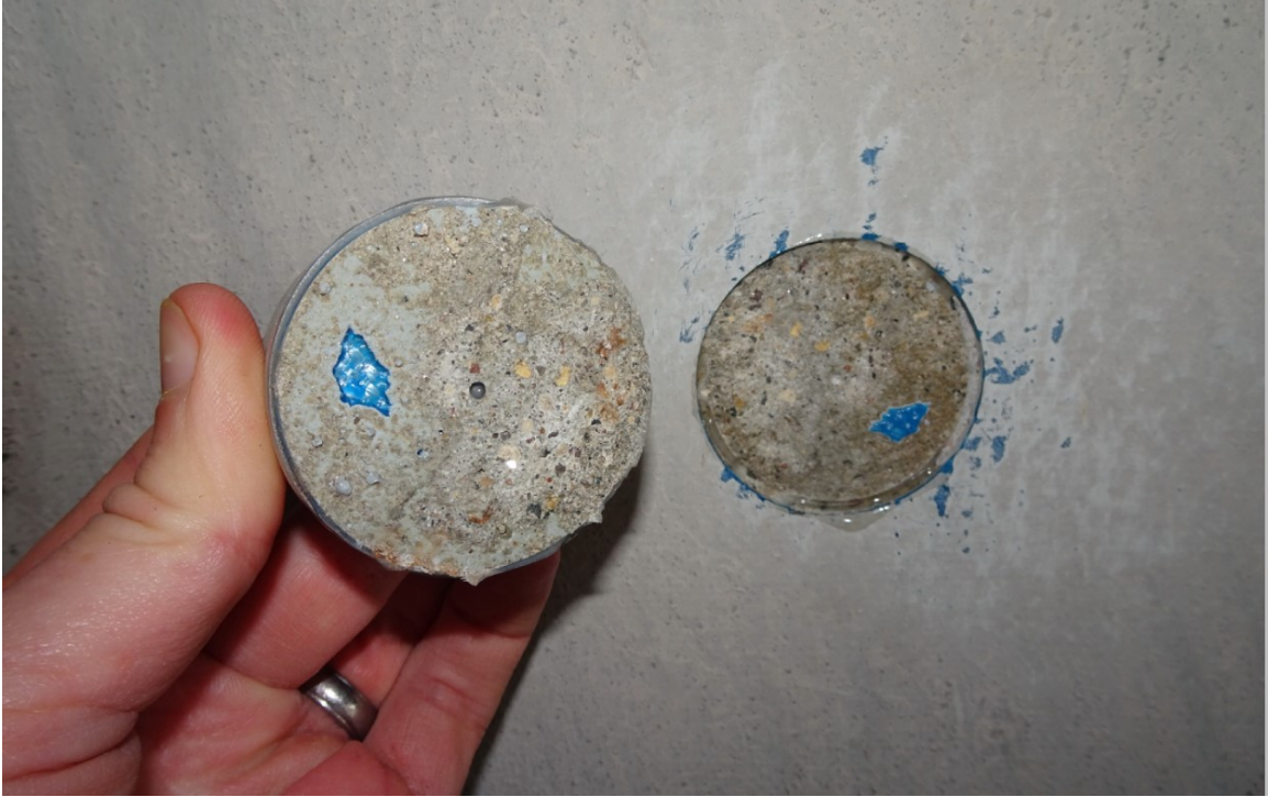
Figure 3.33 Pull-off testing of FRP wrap - cohesive failure in the concrete substrate
