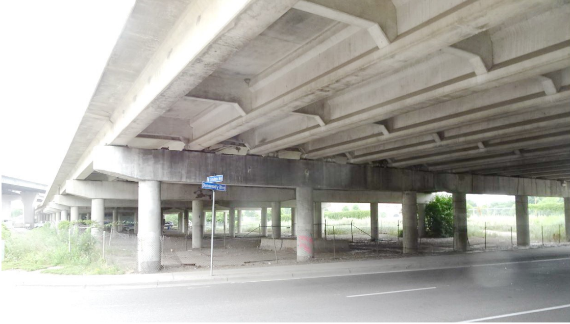
Figure 2.2 Bridge 27831 substructure, looking east at Pier 34WB and Pier 34EB
