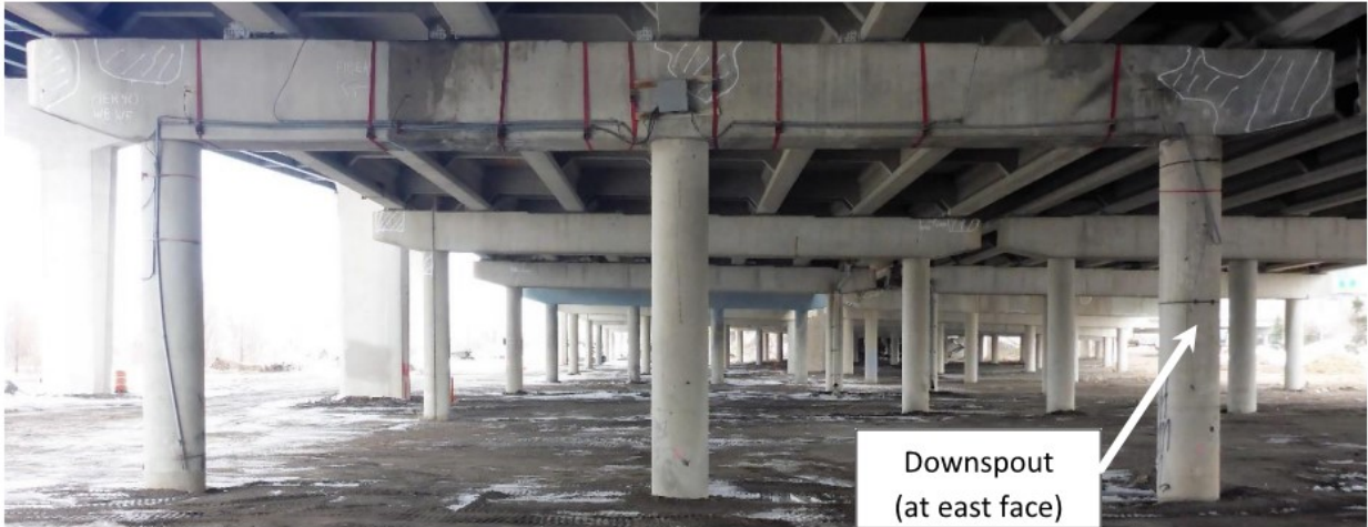
Figure 3.18 Pier 40WB - West Face
