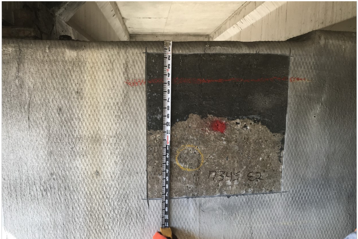
Figure 3.34 Pier 34EB - Example CFRP removal to facilitate locating of core sample
