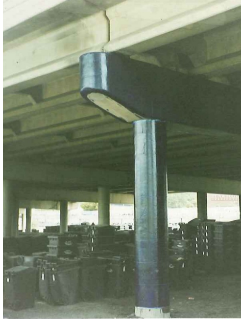
Figure 1.5 Typical FRP wrap installation on a bridge column
