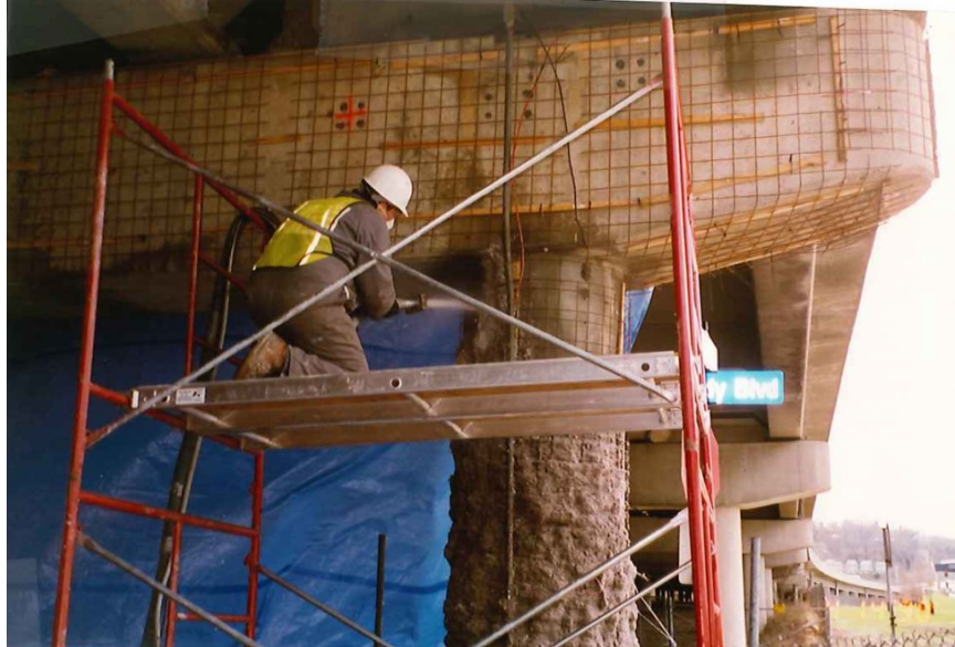
Figure 1.3 In-progress installation of ECE system
