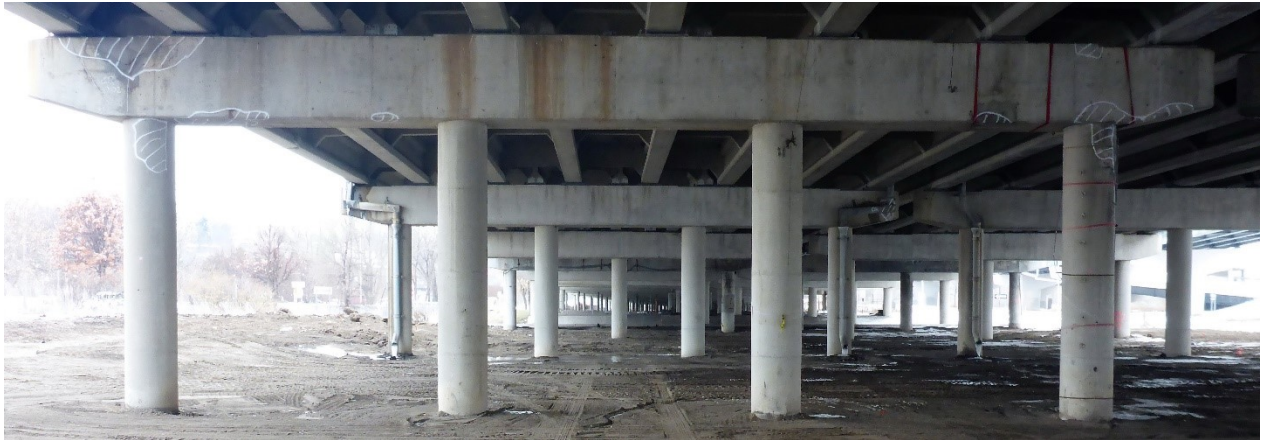
Figure 3.16 Pier 37EB - East Face
