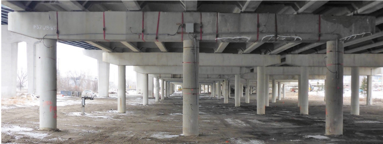
Figure 3.10 Pier 37WB - West Face
