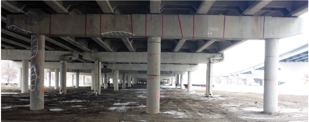
Figure 3.12 Pier 37WB - East Face
