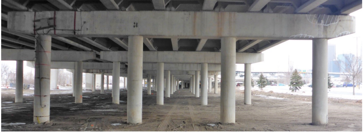
Figure 3.14 Pier 37EB - West Face
