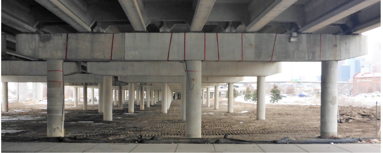
Figure 3.6 Pier 34EB - West Face
