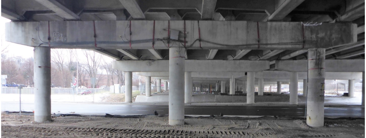
Figure 3.8 Pier 34EB - East Face
