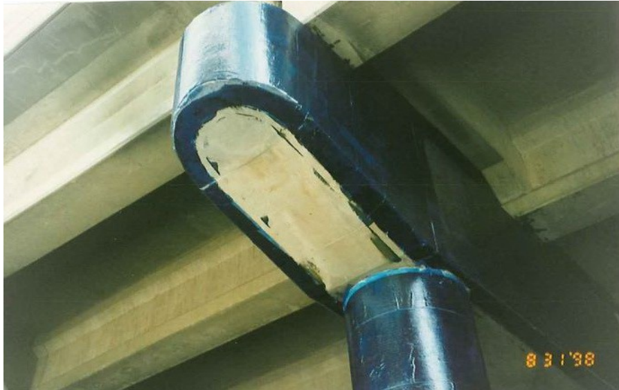
Figure 2.15 Pier 37WB - MBrace CFRP installation before application of UV coating.
