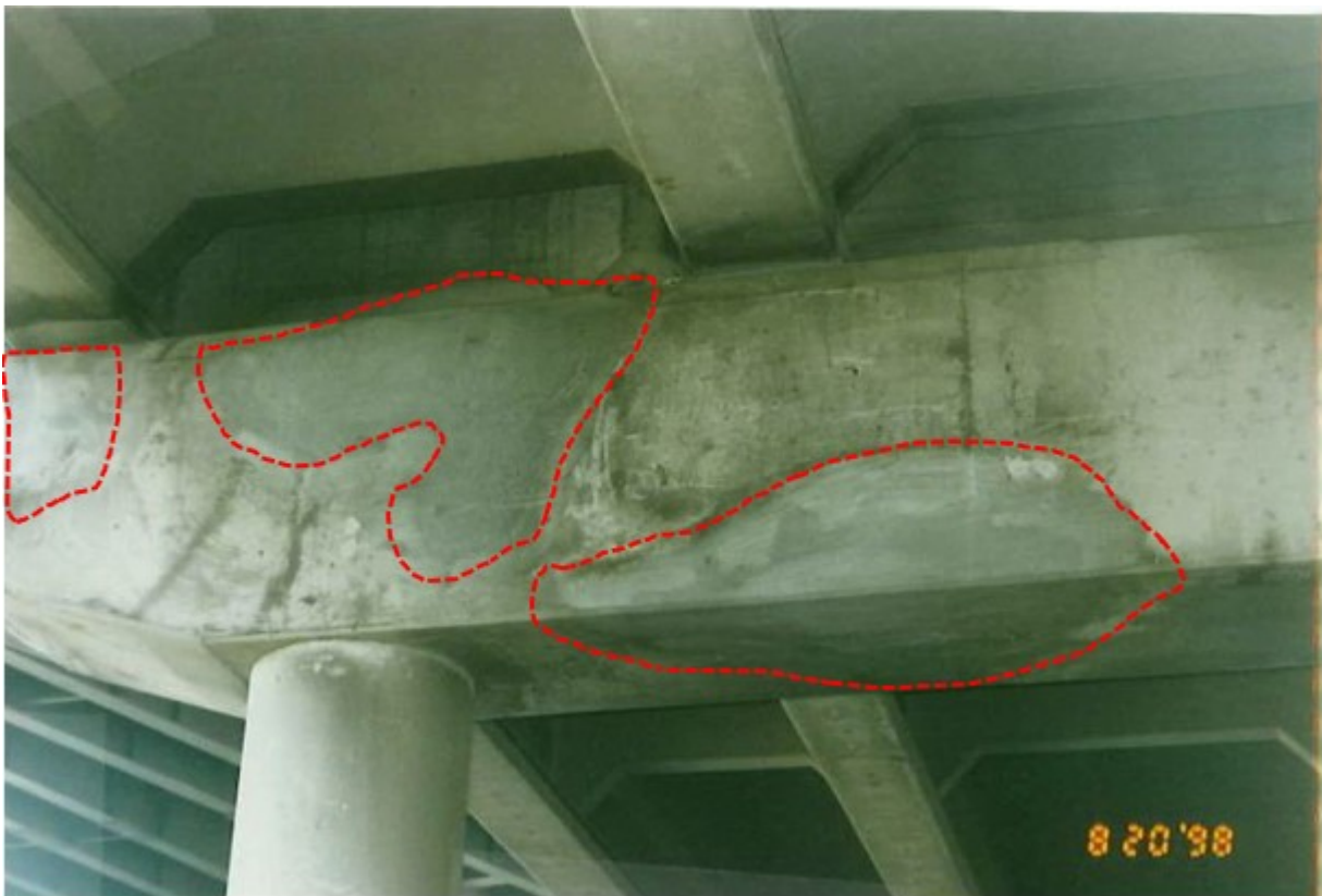
Figure 2.5 Example concrete repairs performed in 1997 (west face of Pier 40WB shown)
