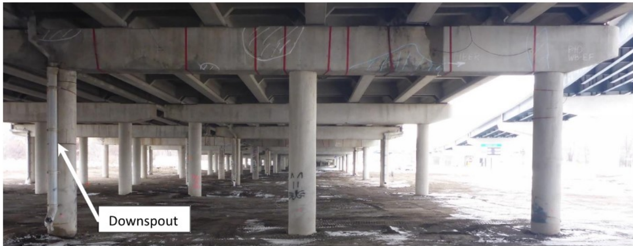
Figure 3.20 Pier 40WB - East Face
