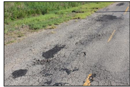
Figure 1.4: Ineffective patching.
