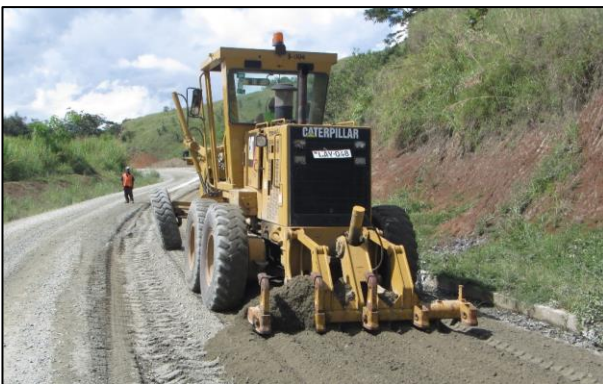
Figure 5.2: Grader ripper bar used to breakdown and mix materials.
