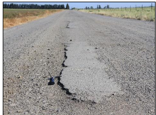
Figure 4.3: Strip of asphalt surfacing left after conversion.
