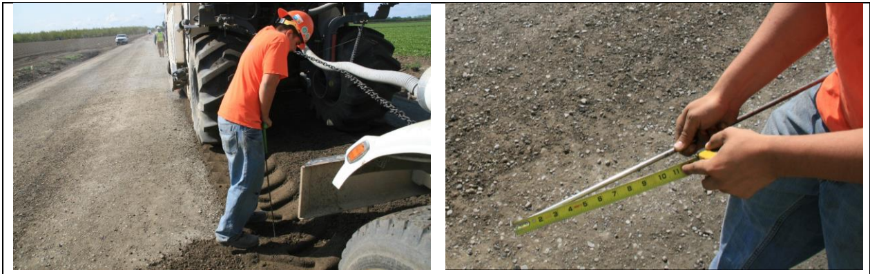
Figure 5.7: Depth control measurements with a T-bar.
