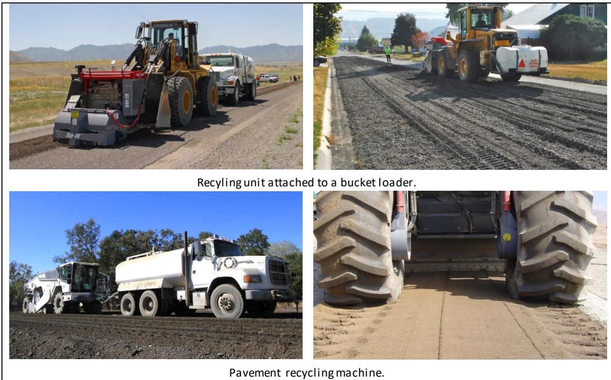
Figure 5.1: Examples of recycling machines and milled/mixed materials.
