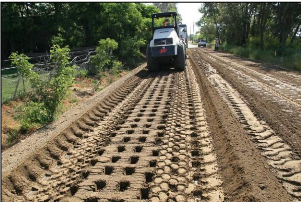
Figure 5.11: First and final pass of a padfoot roller.
