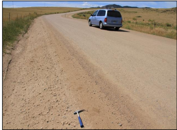
After (Unpaved Road)
