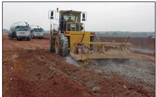
Figure 5.3: Disc plough used to mix materials after ripping with a grader.
