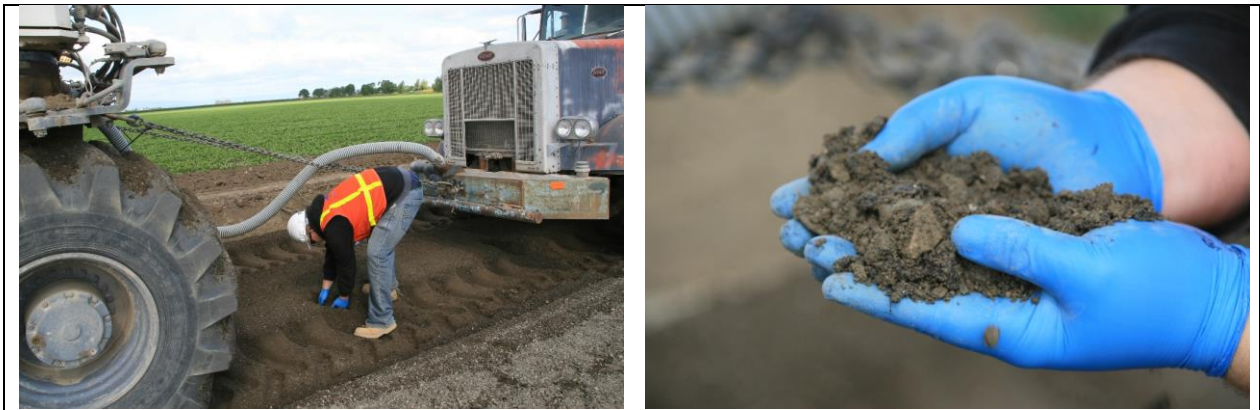
Figure 5.8: Checking material grading, mixing consistency, and moisture content behind the recycler.
