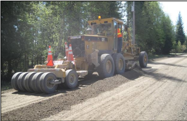
Figure 5.14: Roller attached to grader.
