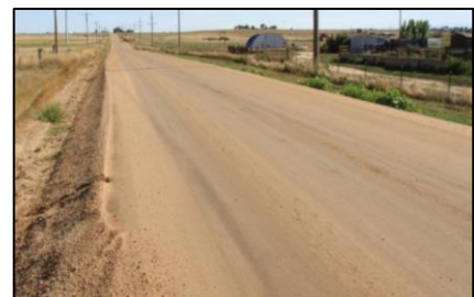
Figure 1.2: Engineered unpaved road
