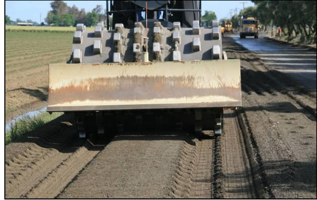
Figure 5.10: First roller pass.
