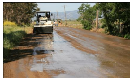
Figure 5.12: Final compaction.
