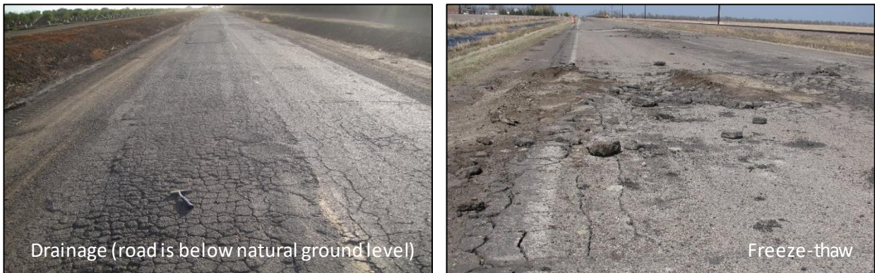
Figure 3.12: Examples of age plus environment-related distresses.
