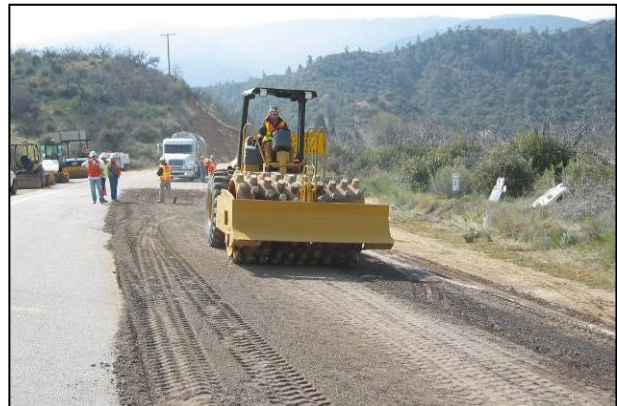
Figure 5.11: First and final pass of a padfoot roller.
