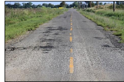
Figure 3.3: Frequent patching.
