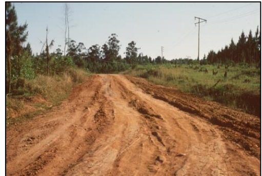
Figure 4.2: Converted road with high plasticity materials.
