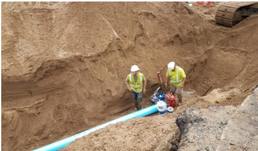
Figure 3.1 Construction crew installing a water line, Chaska, Minnesota [Photo Credit: Bolton & Menk, Inc.]
