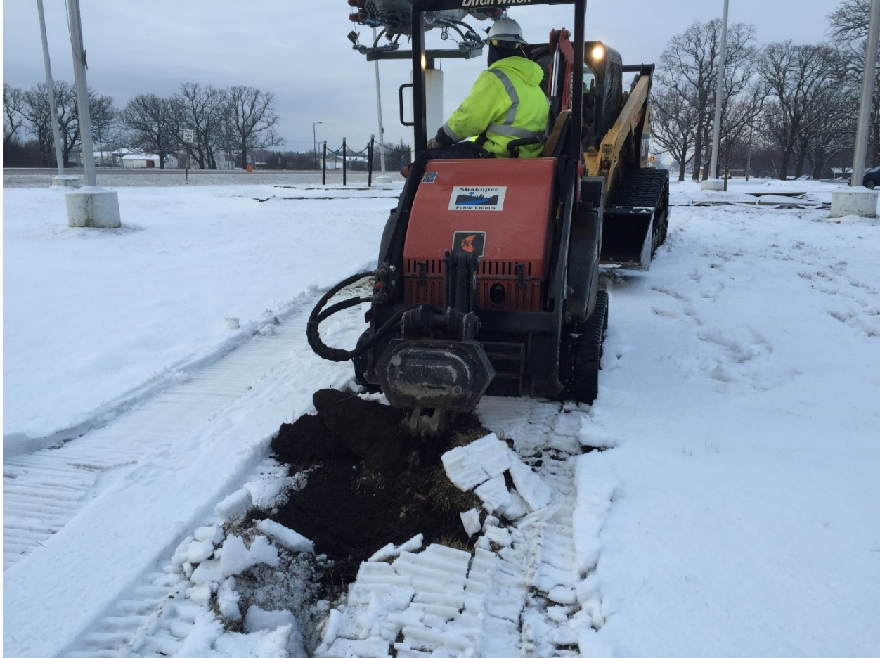
Figure 4.1 Winter utility installation using a ditch witch, Shakopee, Minnesota [Photo Credit: Bolton & Menk, Inc.]
