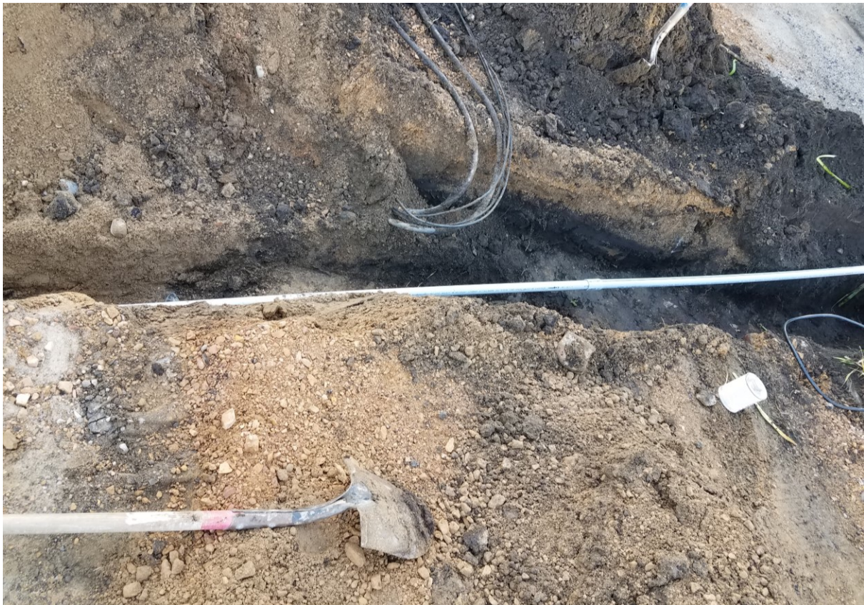
Figure 5.1 New conduit installation (center) and abandoned lines (top), Chaska, Minnesota [Photo Credit: Bolton & Menk, Inc.]
