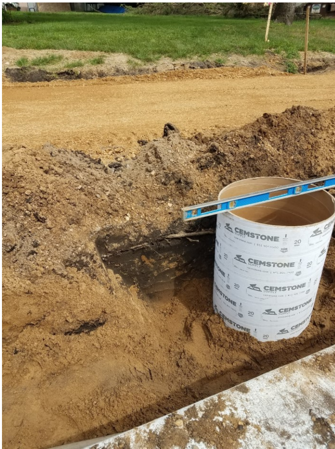
Figure 5.4 New light pole base installation, Chaska, Minnesota [Photo Credit: Bolton & Menk, Inc.]
