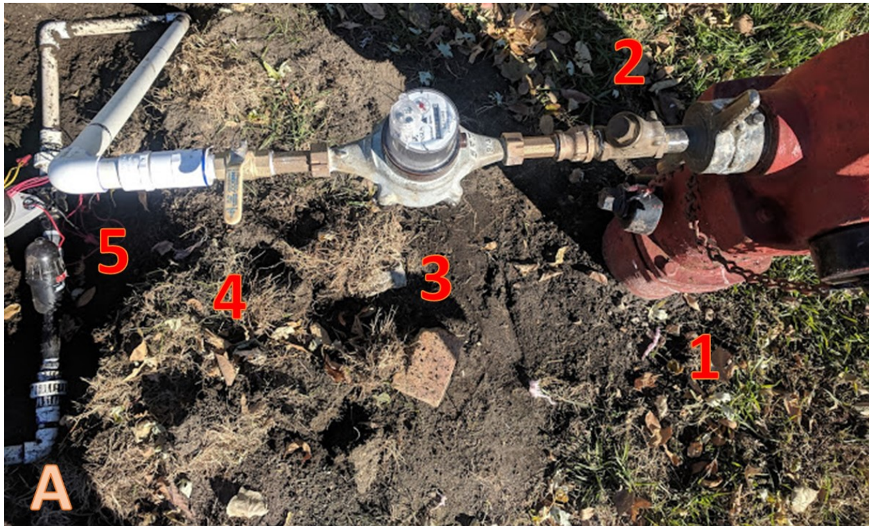
Figure 3.2 Hydrant meter assembly.
