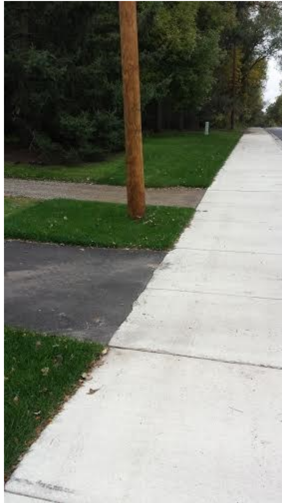
Figure 2.9 New roadside project shows breaks in turf where irrigation would have to move over a driveway.
