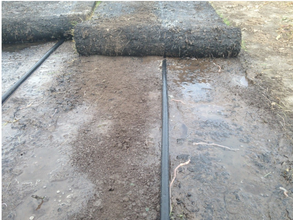
Figure 2.2 Below sod drip irrigation system on 18-inch (45.7-cm) row spacing with a flow rate of 0.45 gph (1.7 liters per hour).
