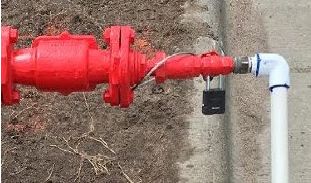
Figure 4.8 Mainline point of connection.
