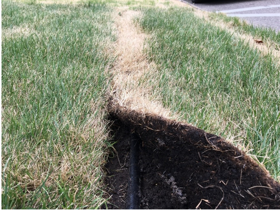
Figure 4.13 Sod not rooting directly above drip irrigation lines.
