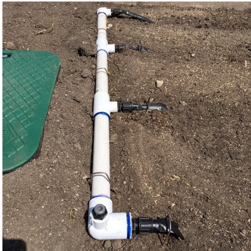
Figure 4.11 Drip footer with air relief valve.
