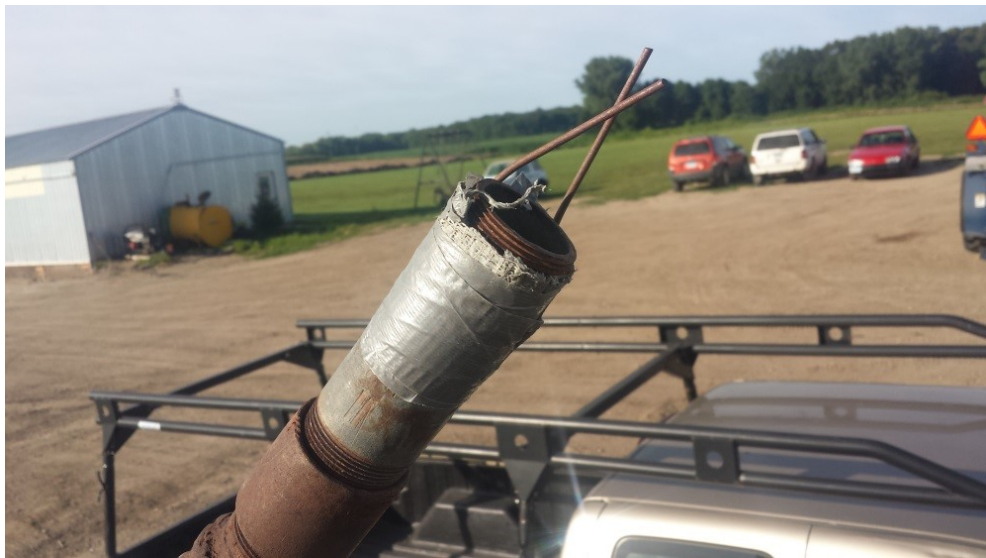
Figure 2.4 Sod staple taped to an open pipe for distribution of water. This is an example of a poor existing setup.
