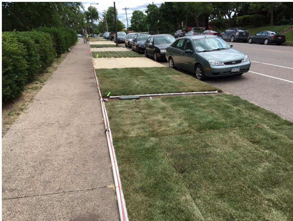
Figure 4.3 Como Avenue site following installation.
