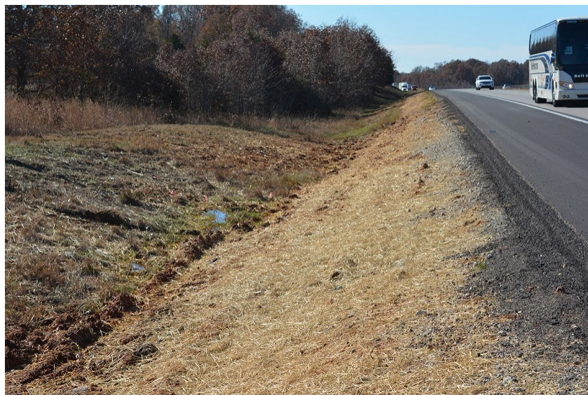
Figure 2.15 The final configuration of the test site
