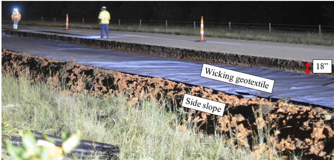
Figure 2.9 Horizontal placement of wicking geotextile in test section 2
