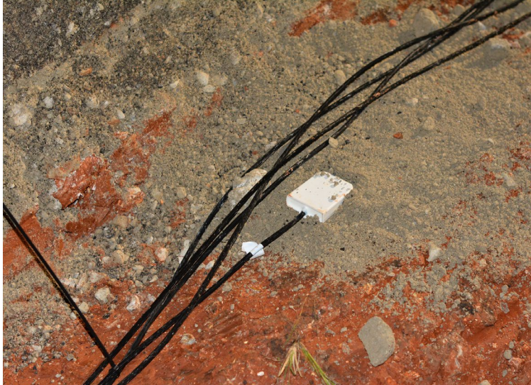
Figure 2.7 Sensor installation in the subgrade soil
