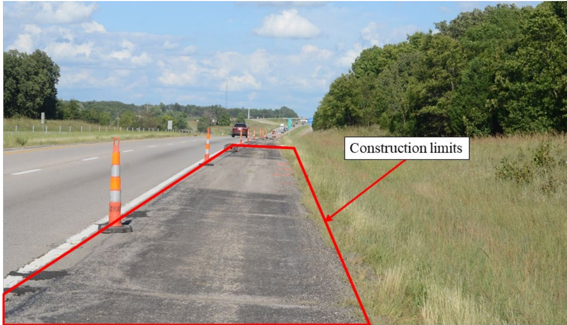
Figure 2.4 View of the site before construction
