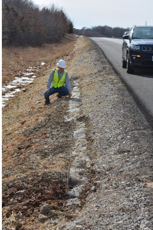
Figure 2.16 Exposing the outer end of the wicking geotextile on February 9, 2019
