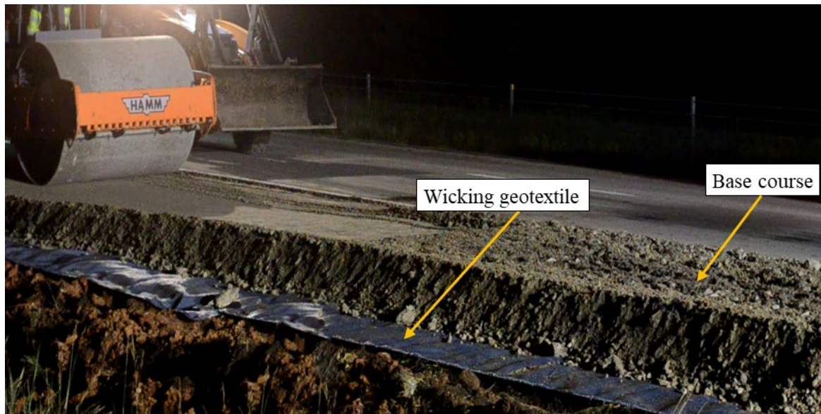
Figure 2.11 Compaction of the base course
