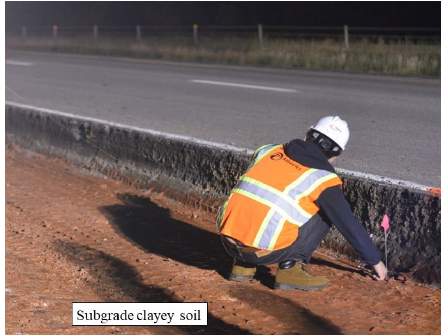
Figure 2.6 View of the shoulder after excavation
