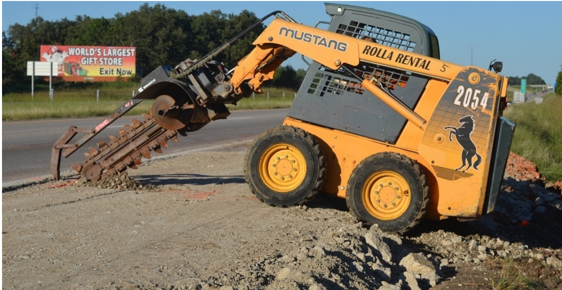
Figure 2.12 Preparing a trench for sensor installation using a trench-digger
