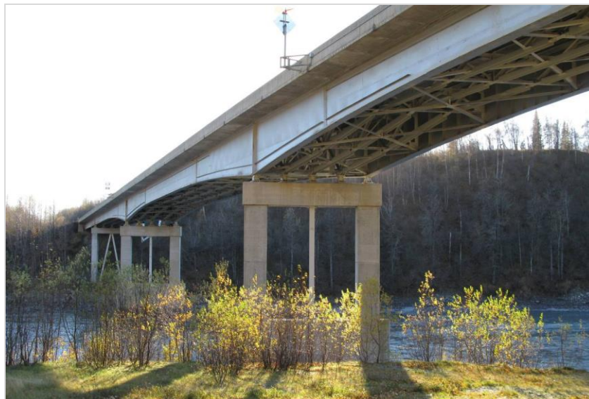
Figure 1.1 Chulitna River Bridge, after 1993 upgrades
