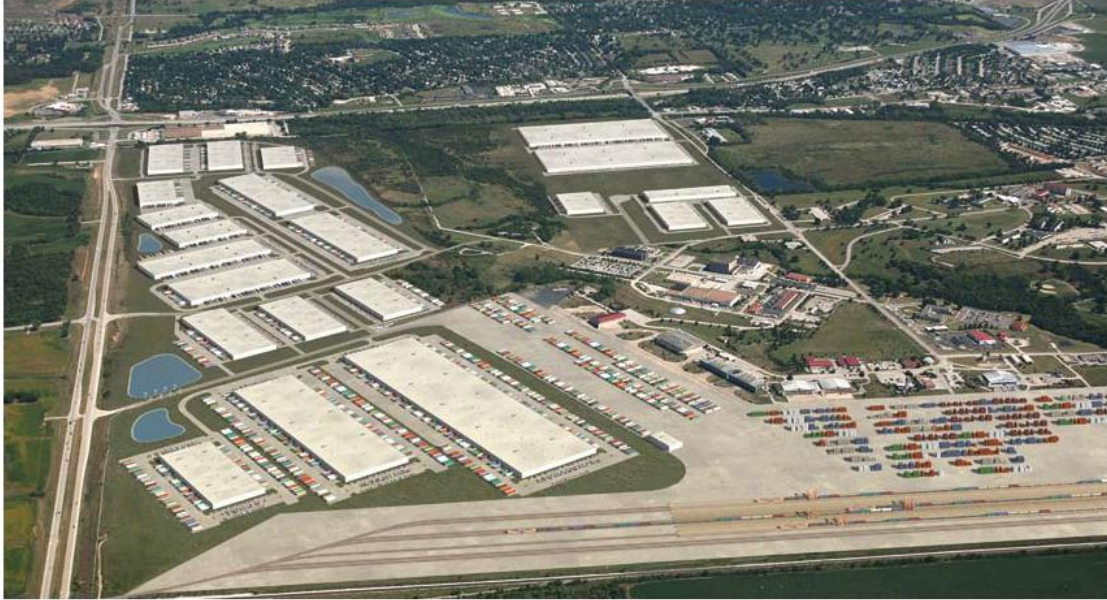
CenterPoint Intermodal Center, Kansas City
