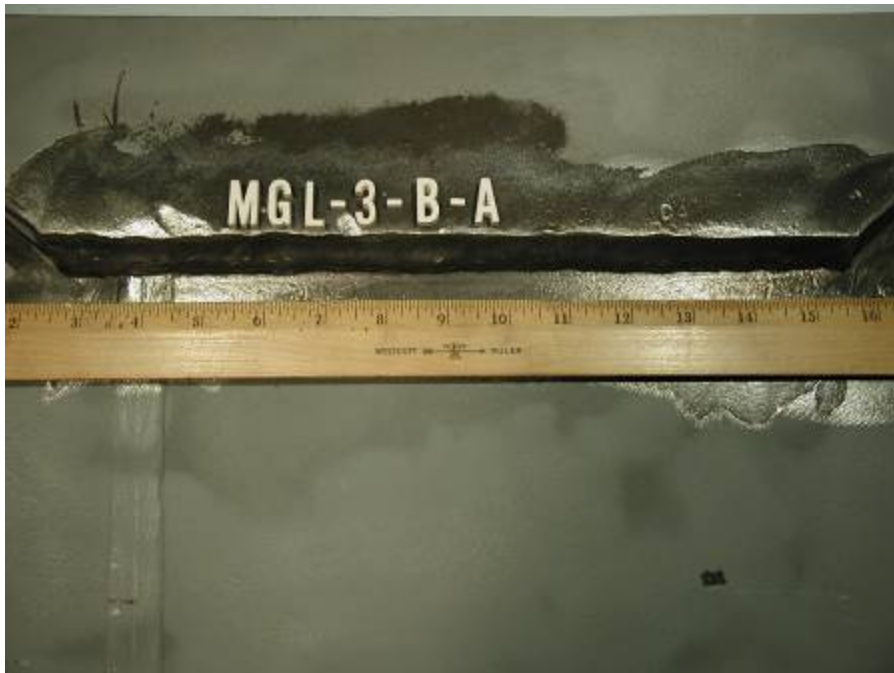
Figure 24. Tank Car Fillet Weld Master Gage with Fatigue Cracks at Weld Terminations
