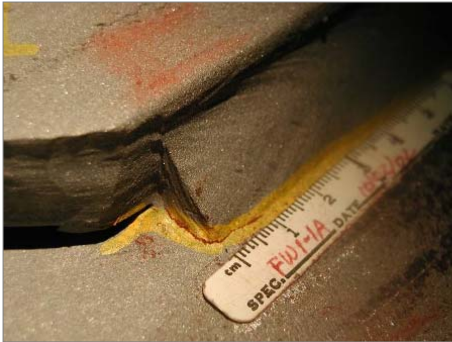
Figure 19. Magnetic Particle Indication Showing an Artificially Induced Fatigue Crack at the Termination of a Tank Car Fillet Weld
