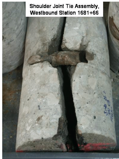
Figure 5. Shoulder Tie Assembly, Westbound Station 1681+66
