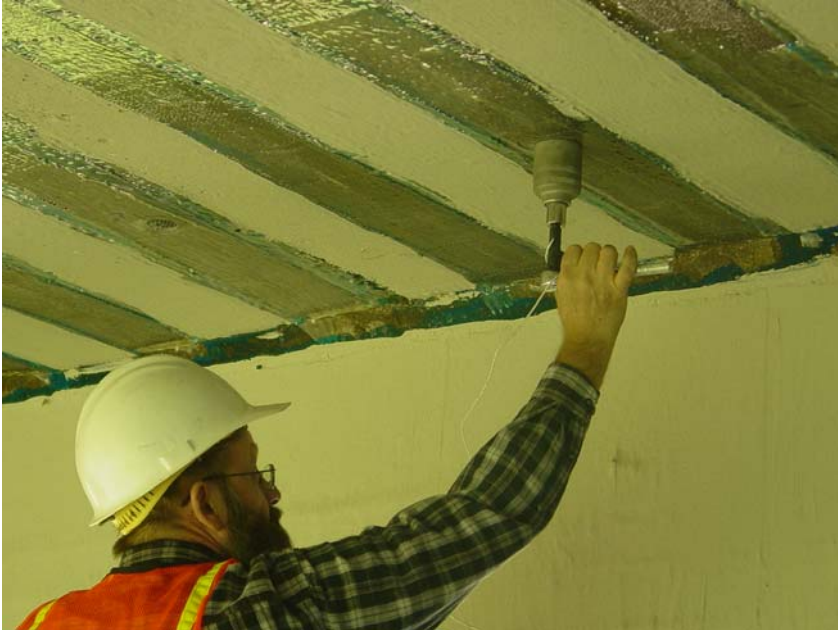
Figure 4.5: Pull-off test on the deck plugs.
