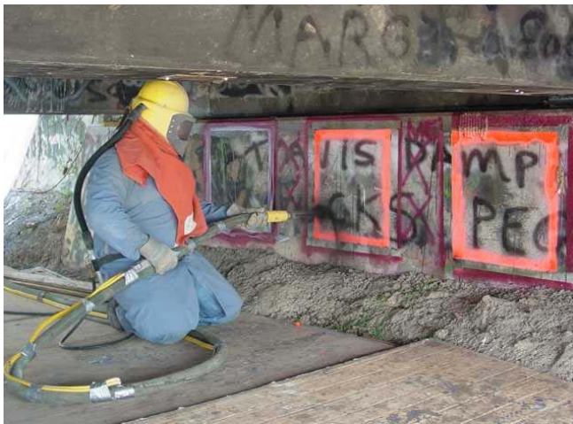
Figure 1.5: Sandblasting for the test panels on the abutment (left) and one of the bents (right).
