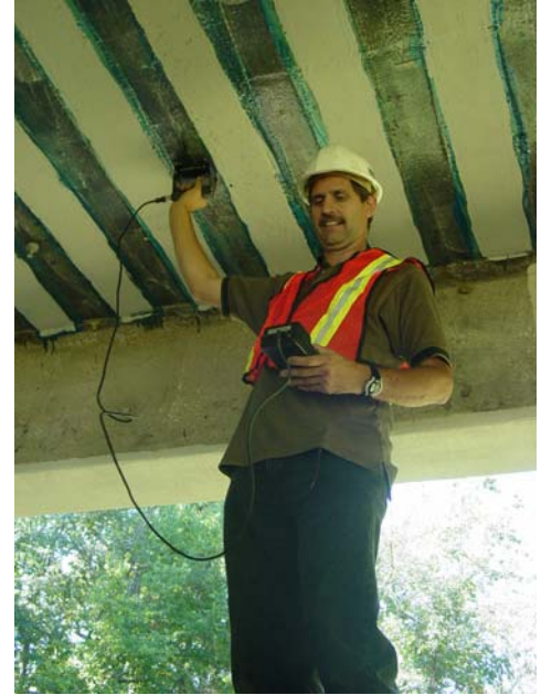
Figure 4.6: Impact echo test on the deck failed plug location.
