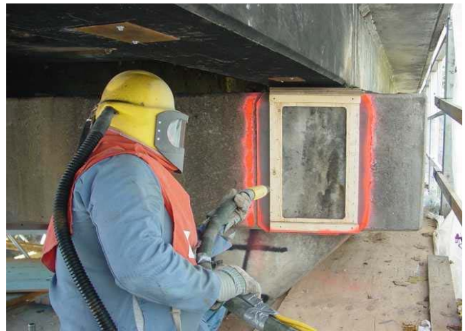
Figure 1.5: Sandblasting for the test panels on the abutment (left) and one of the bents (right).
