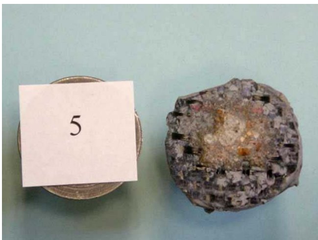
Figure 4.11: Example of composite separation, starting at the top coat of epoxy and extending into the concrete.
