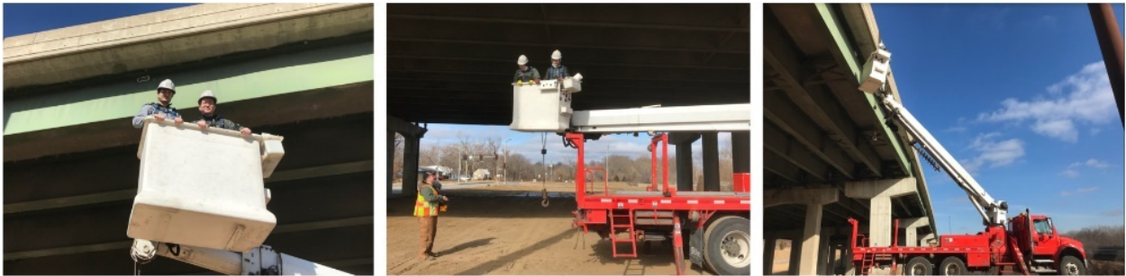
Figure 6.14: Field Deployment of the Monitoring System on a Steel Bridge
