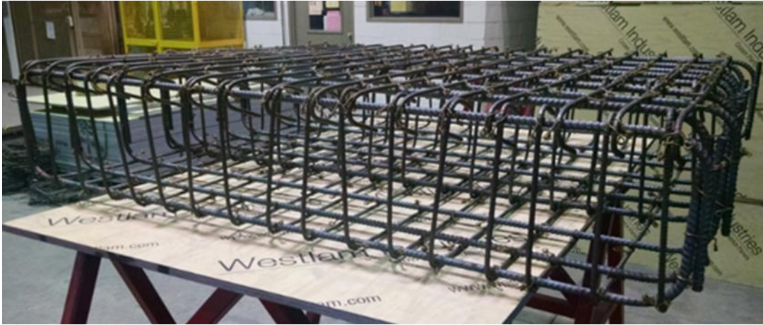
Figure 2.5 As-built wall footing reinforcement
