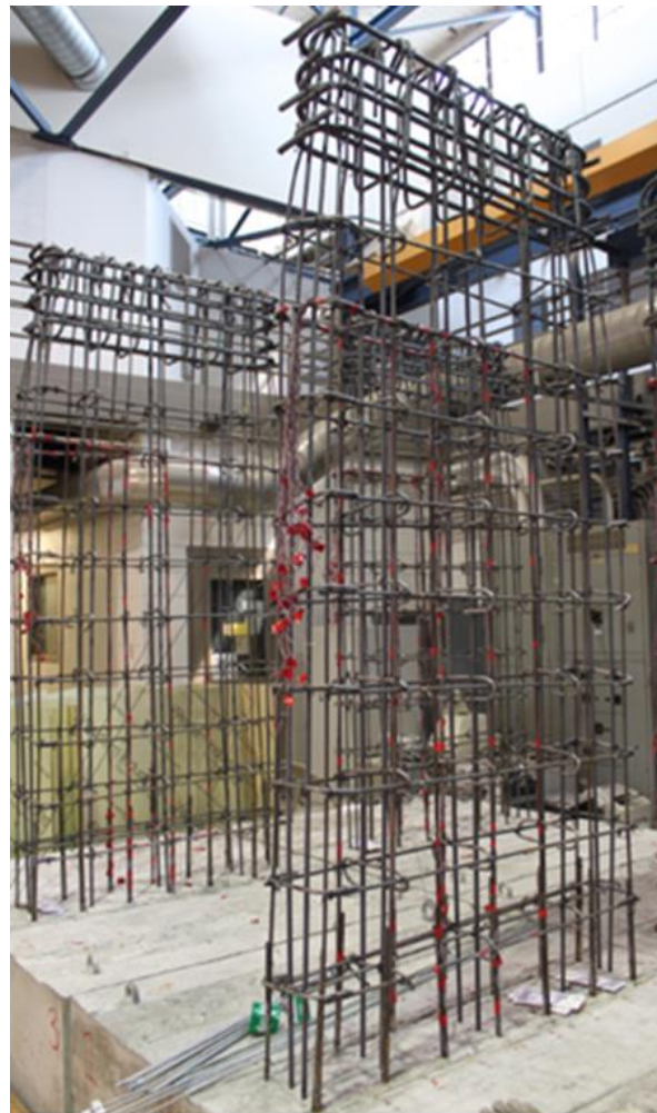
Figure 2.6 As-built wall pier reinforcement
