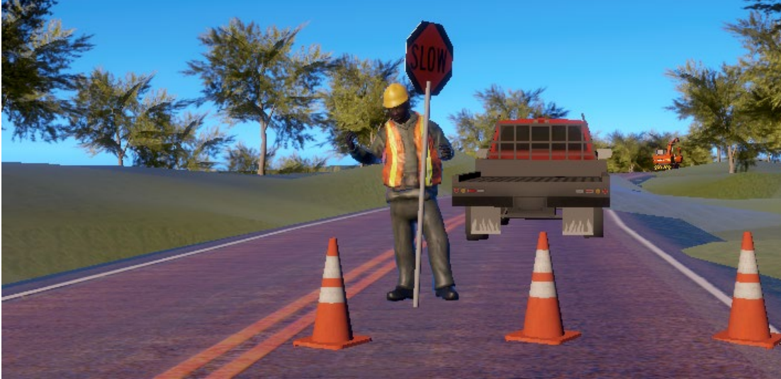
Flagger releasing traffic with slow sign
