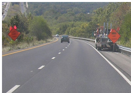
Damage and duct tape (MoDOT)
