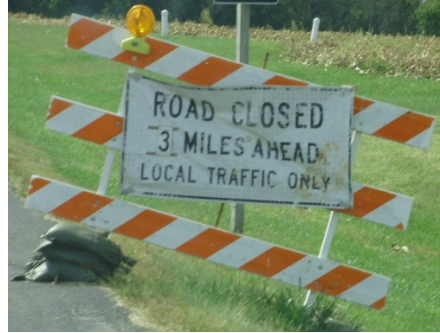
Damage and placed incorrectly (MoDOT)
