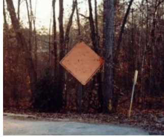
Damage (North Dakota)
