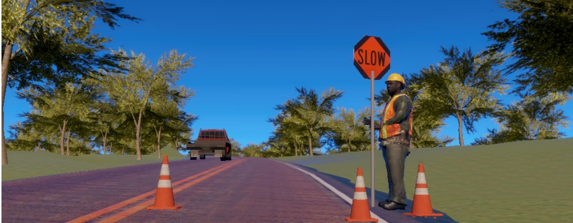
Flagger releasing traffic with slow sign
