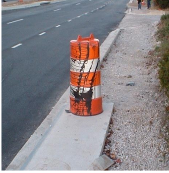
Damage (North Dakota)
