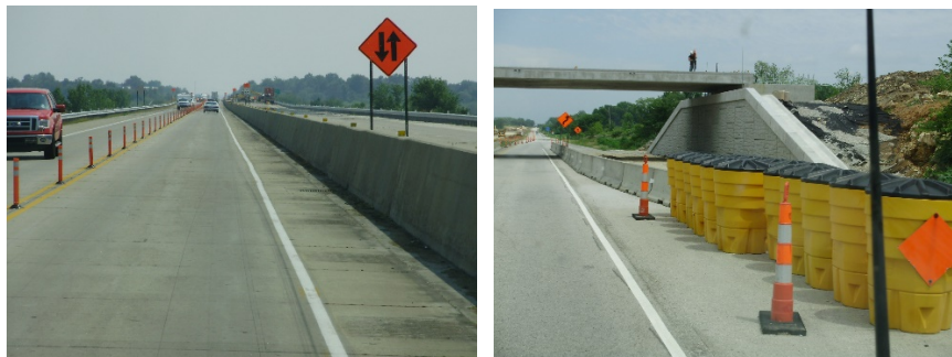
Figure 3.10 Example of temporary traffic barriers (MoDOT)
