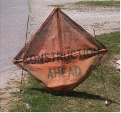
Damage and placed incorrectly (NDSC)
