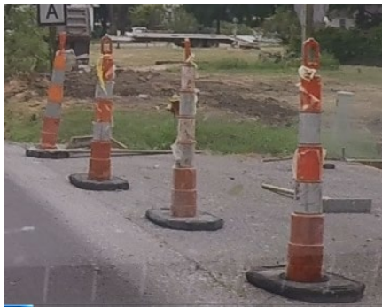
Damaged trim-line (MoDOT)
