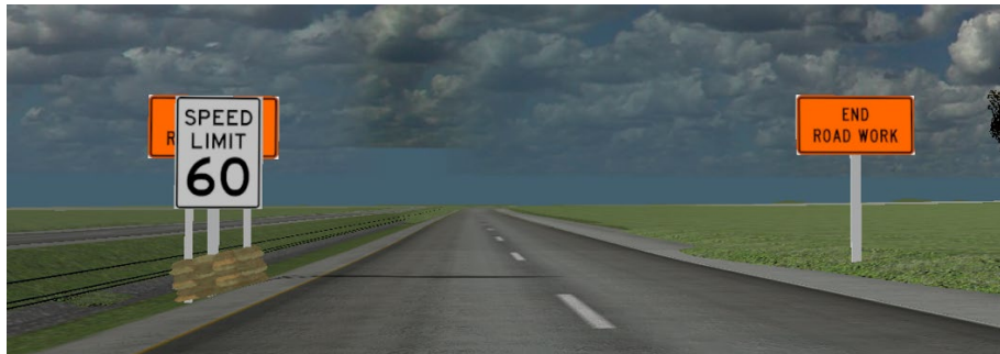
End road work sign covered by speed limit sign and large mound of sandbags
