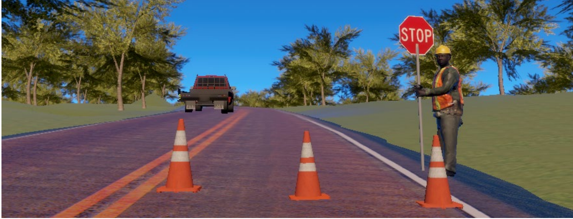
Flagger holding the stop sign
