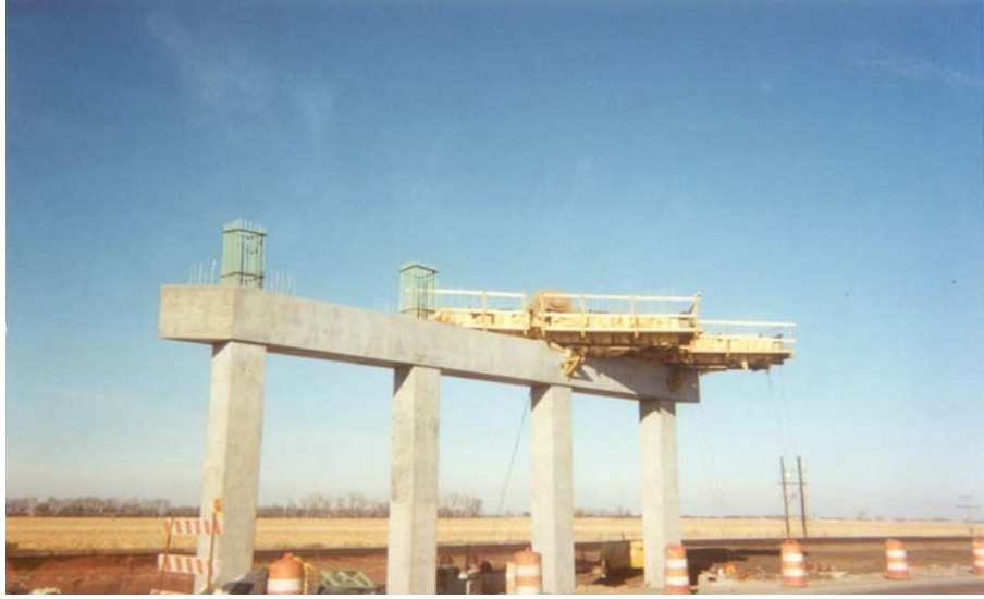
Figure 4.6 Pier Setup and Haunch Block Forming
