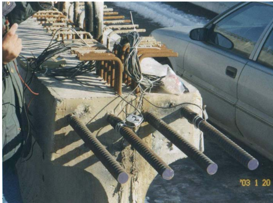
Figure 4.20 Strain Gauges Attached to Threaded Rods in the Precast Yard
