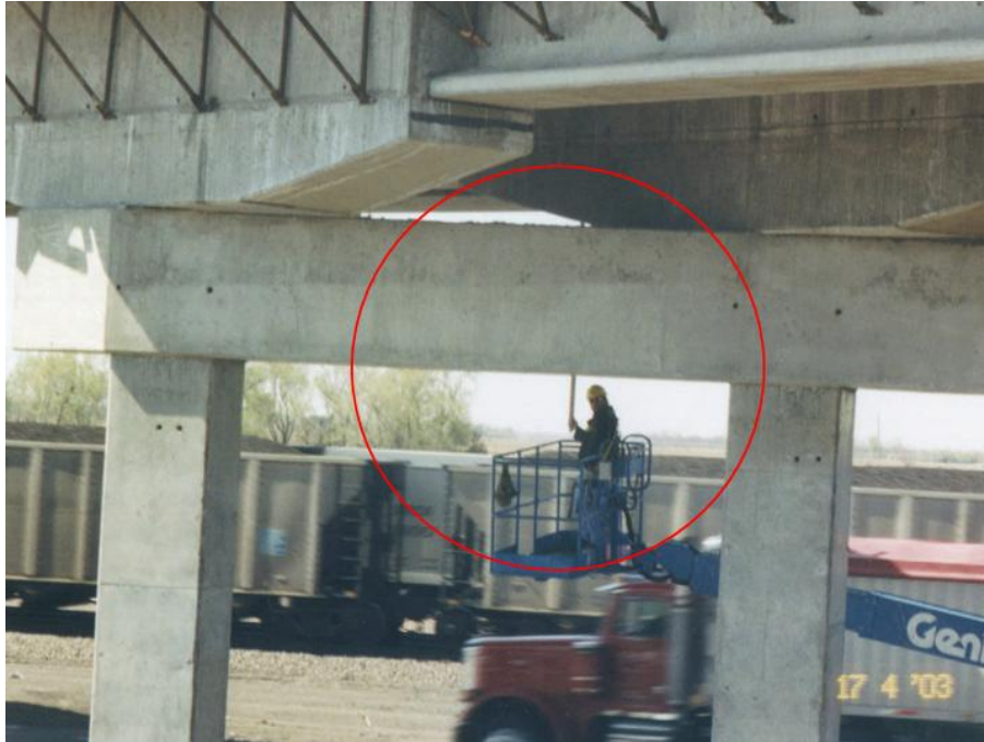
Figure 4.25 Determination of Girder Deflection
