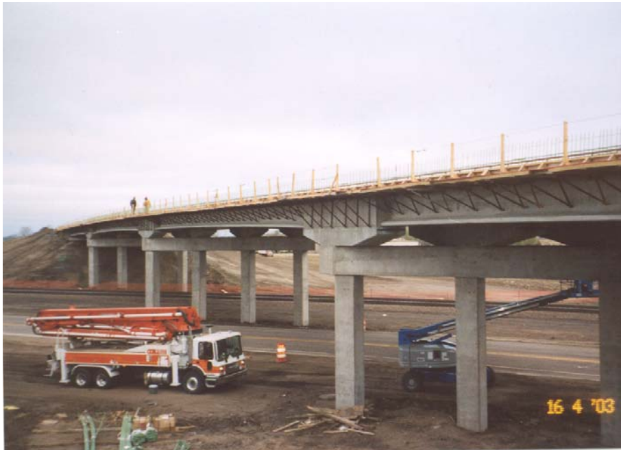
Figure 4.15 Side View of Deck Forming
