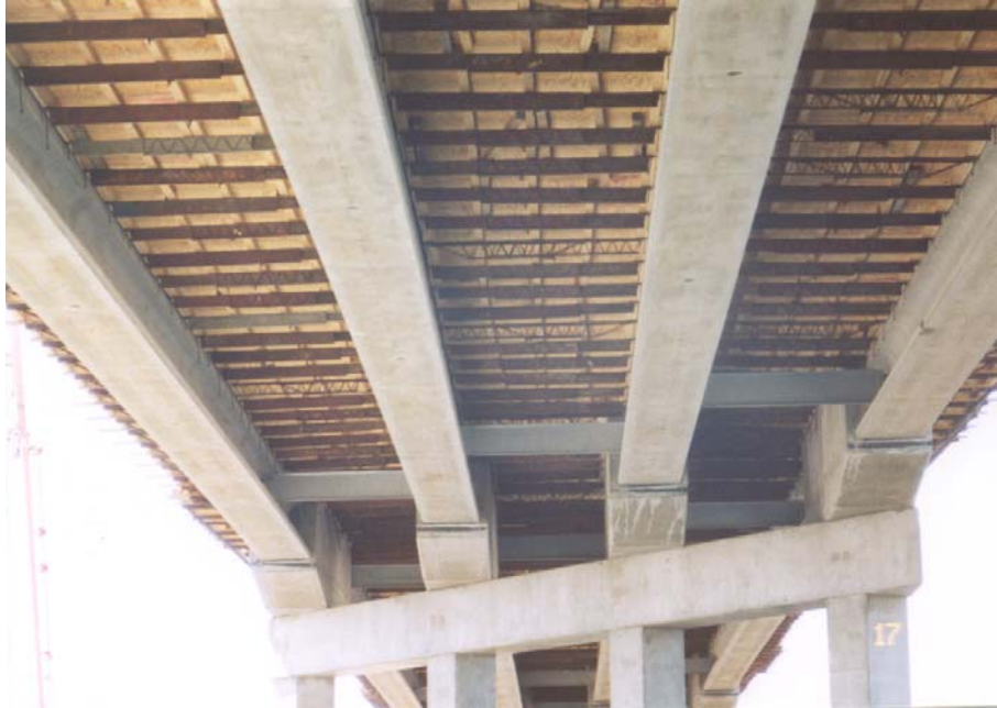
Figure 4.16 View of Deck Forming below the Bridge
