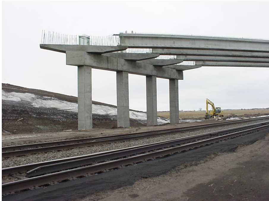
Figure 4.9 Precast Girders Placed on Pier Haunch
