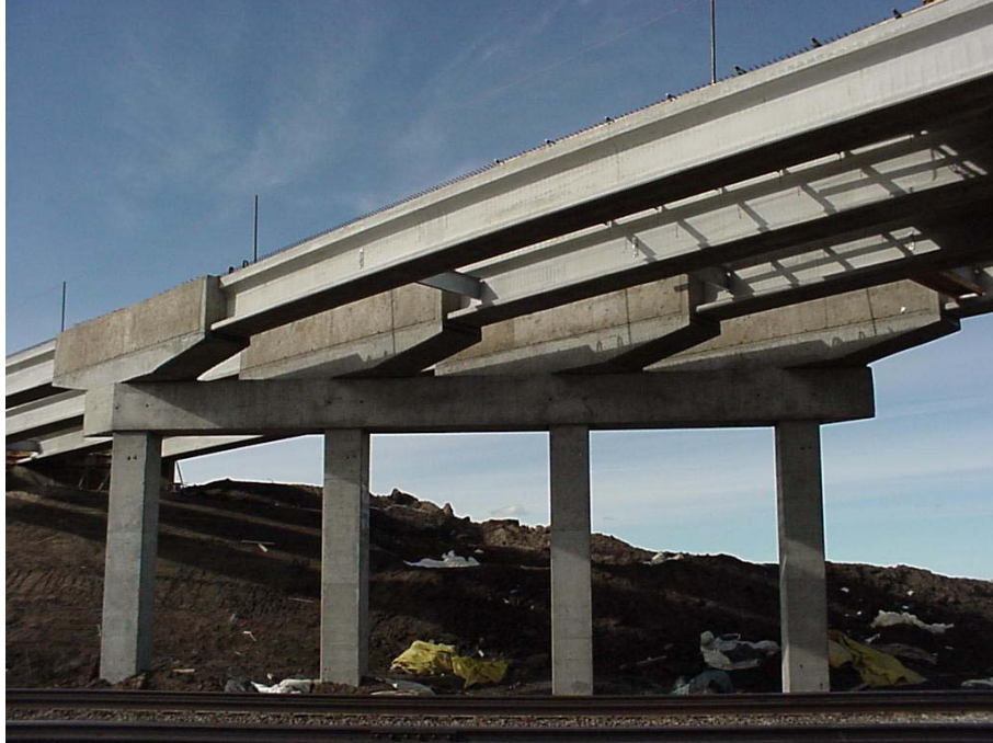
Figure 4.14 Concrete Placement of Continuity Block over Pier
