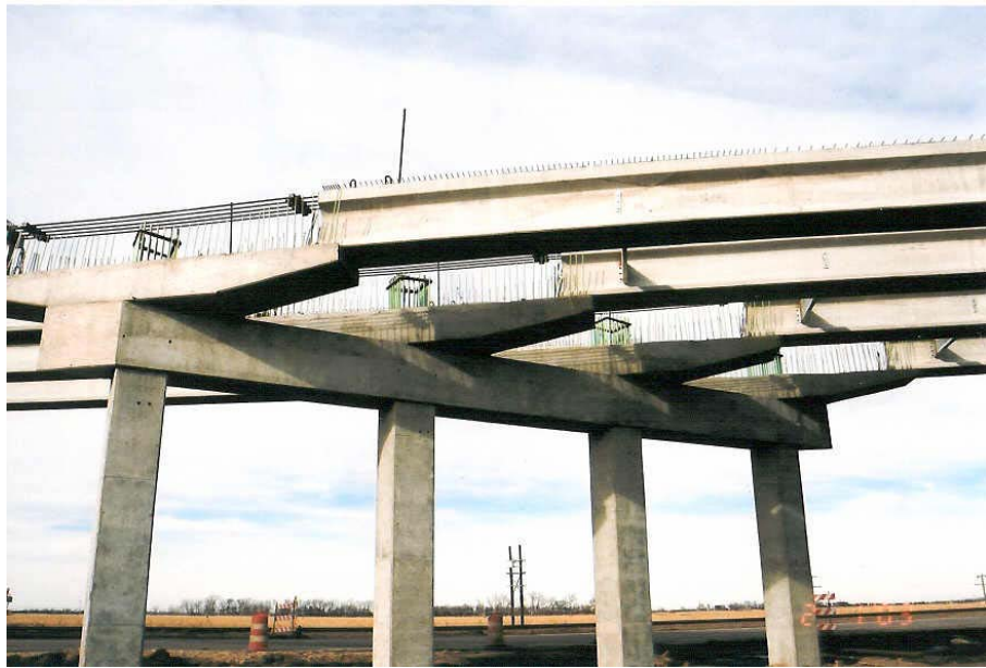
Figure 4.11 Precast Girder Coupled by Bolted Connection Detail
