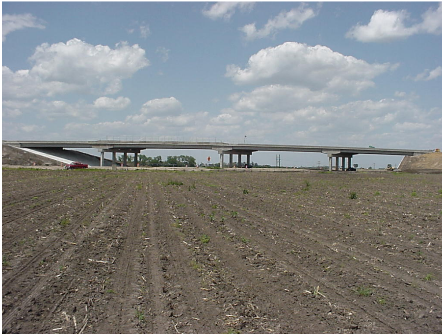
Figure 4.19 Completion of Bridge Construction
