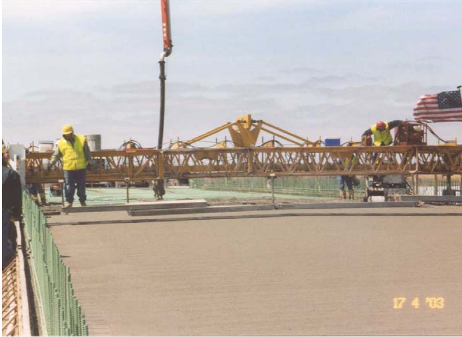
Figure 4.18 Casting the Bridge Deck
