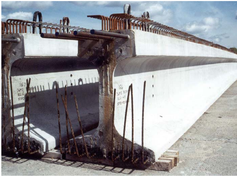
Figure 4.7 Modified NU 1100 I-section Girder in the Precast Yard
