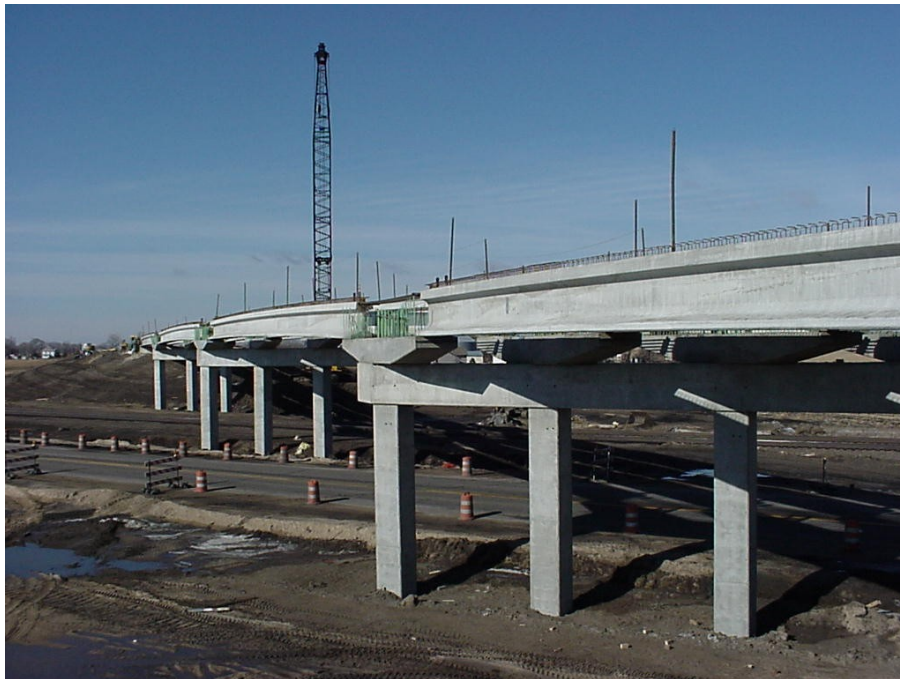
Figure 4.13 Girders Coupled by Threaded Rods before Continuity Block Placement
