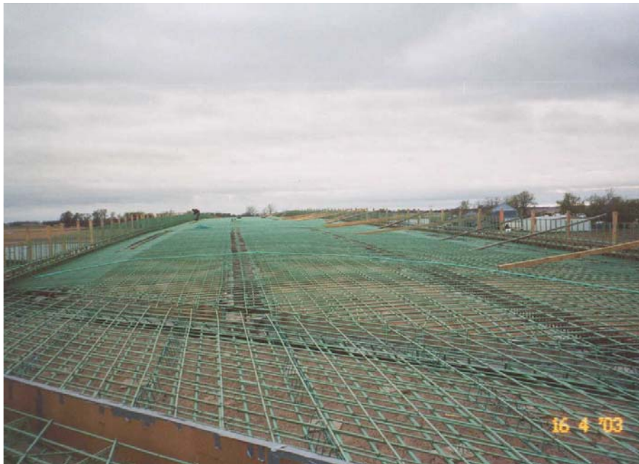
Figure 4.17 Deck Reinforcement Setup
