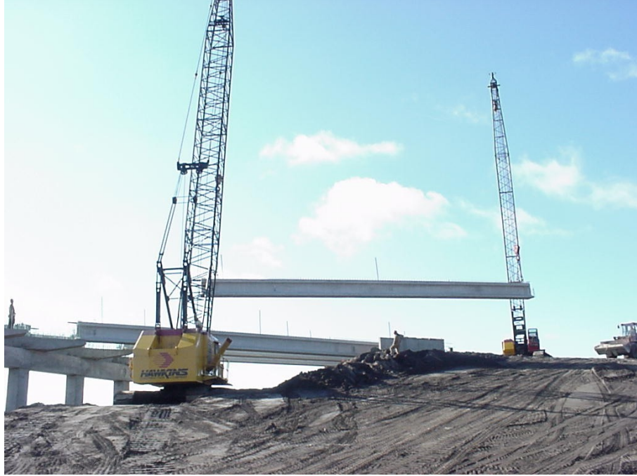
Figure 4.8 Precast Girders during Erection
