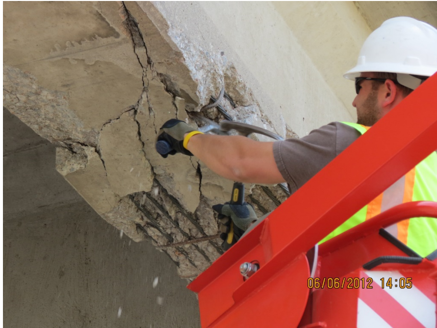
Figure 90: Removing all loose concrete immediately from the girder, York East Bridge, courtesy of NDOT
