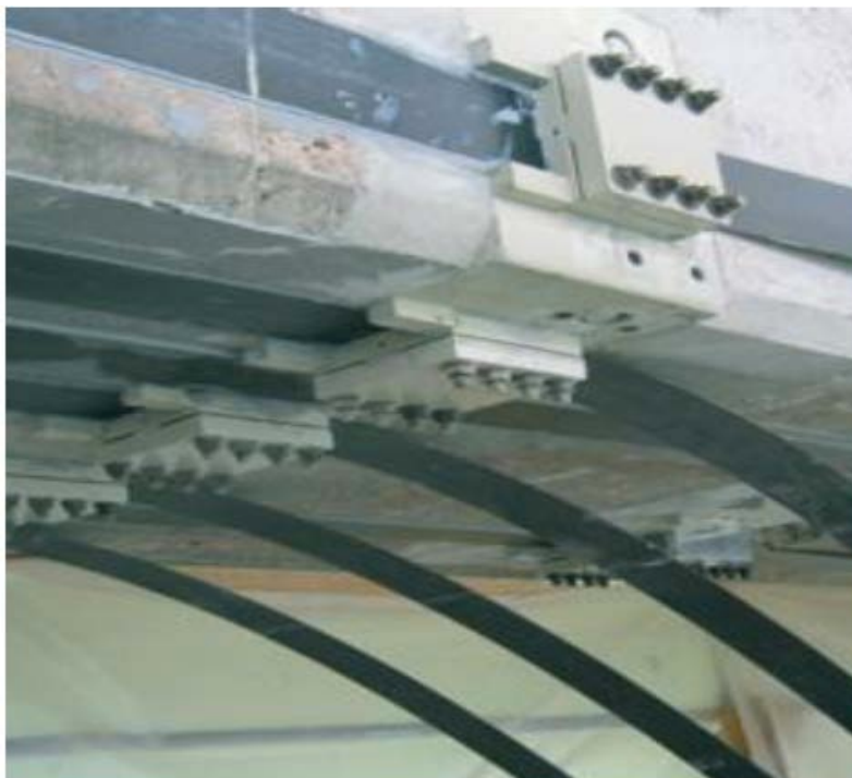
Figure 33: Sika carbostress system external CFRP post-tensioning, courtesy of Kasan, 2009
