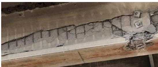
Figure 13: Severe III damage, several damaged strands, NDOT Schuyler Bridge
