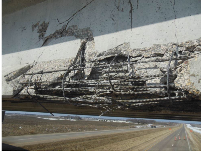
Figure 12: Heavy damage with web cracking and severed mild reinforcing and prestressing strands, courtesy of Iowa DOT, 2014
