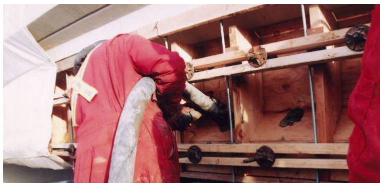
Figure 28: Pumping concrete into plywood formed section, courtesy of Alberta Infrastructure and Transportation, 2005
