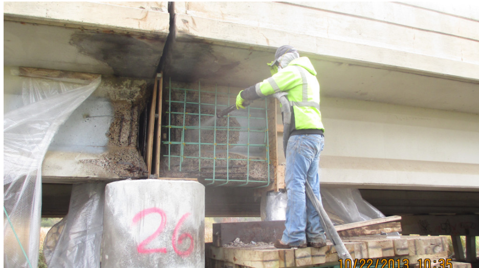
Figure 51: Shotcreting repair at girder end, MN/RC 2018-07 Report
