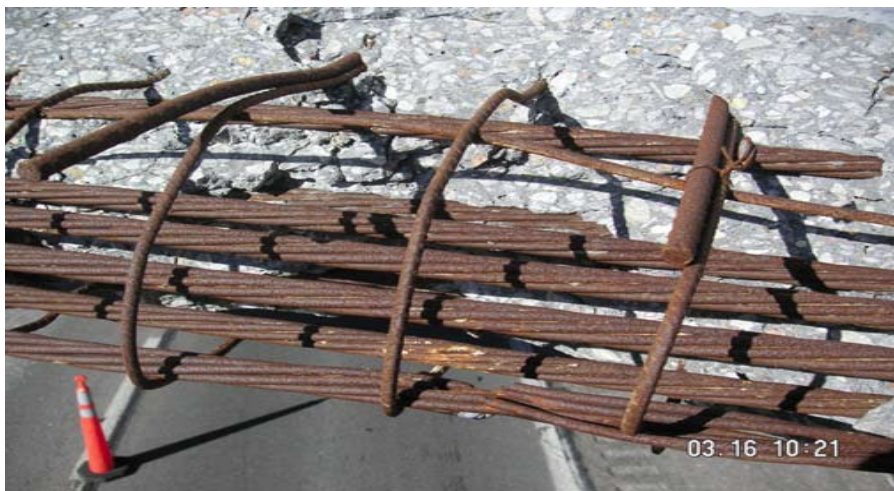
Figure 15: Severe I damage, one severed strand, NDOT Wood River Interchange Bridge Girder (A), courtesy of NDOT
