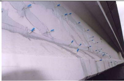
Figure 16: Epoxy injection ports, AIT, 2005
