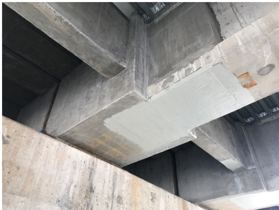
Figure 118: Girder end encasement and CFRP layers, visible crack at the diaphragm, Kearney South Platte River Bridge, courtesy of NDOT
