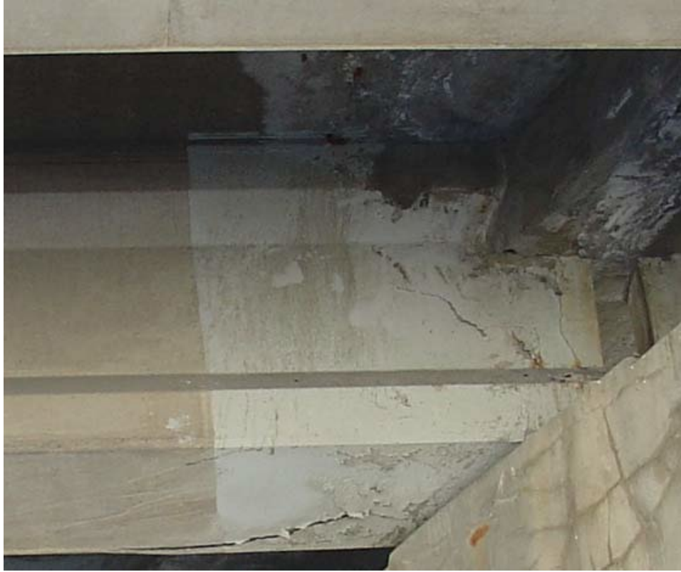
Figure 48: Severe class corrosion damage at girder end causing severe cracks, courtesy of Pantelides et al., 2010
