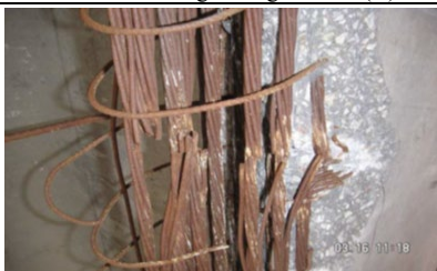
Figure 10: Severe II damage, five severed strands, NDOT Wood River Interchange Bridge Girder (E)
