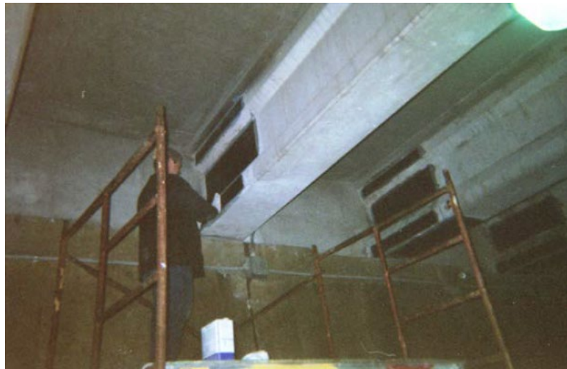
Figure 53: CFRP fabrics installation on I-65 expressway bridge girders, courtesy of Choo et al., 2013
