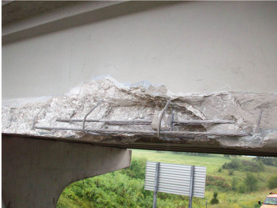
Figure 11: Bottom flange damage with mild reinforcing and prestressing strands intact, courtesy of Iowa DOT, 2014
