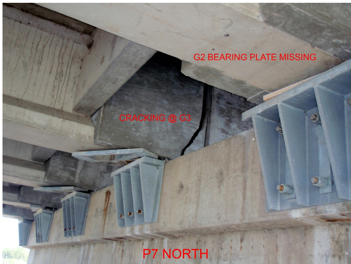
Figure 114: Damage at girder end, Kearney South Platte River Bridge, courtesy of NDOT
