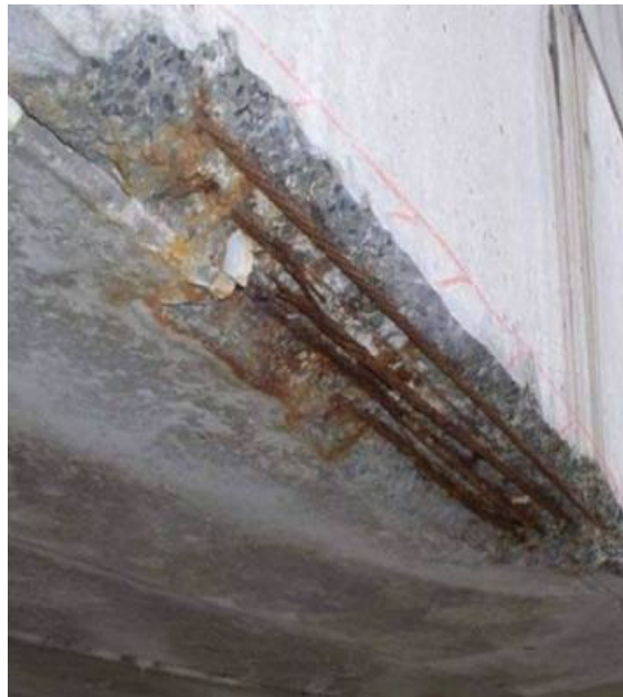
Figure 44: Condition State Poor, exposed strands on concrete bridge girder, courtesy of WisDOT, 2018
