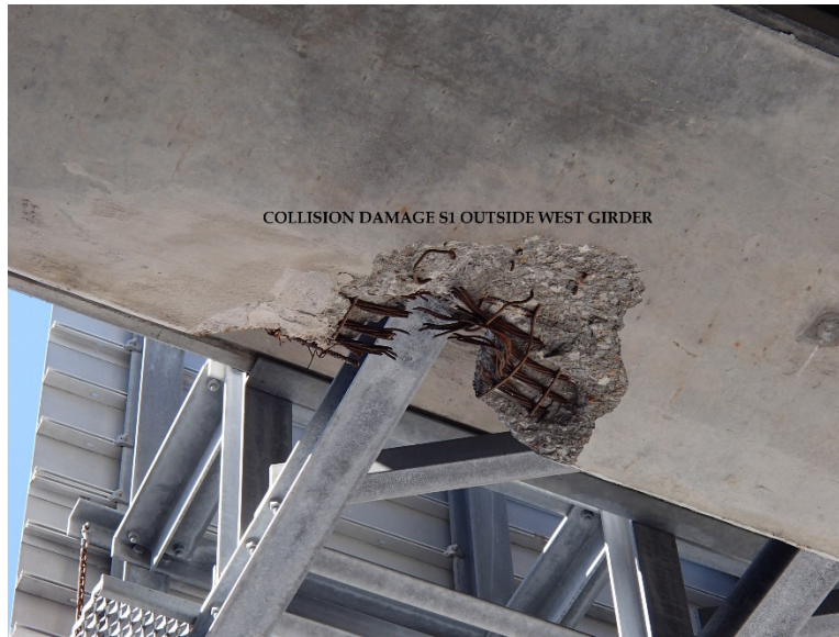
Figure 65: Level of damage, 168 th St. over West Dodge Road Bridge, courtesy of NDOT
