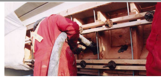
Figure 18: Pumping concrete into plywood formed section, AIT, 2005
