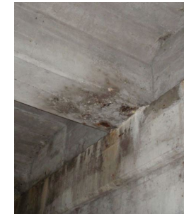
Figure 6: Extensive damage, water saturation, rust staining, and spalling on a cast-in-place concrete T-girder, MnDOT, 2019
