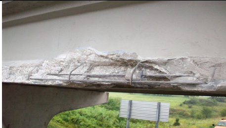
Figure 4: Moderate damage, exposed intact strands, Iowa DOT, 2014
