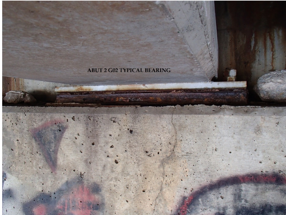
Figure 107: Corrosion damage at bearing assemble, Platte River Bridge East of Grand Island, courtesy of NDOT
