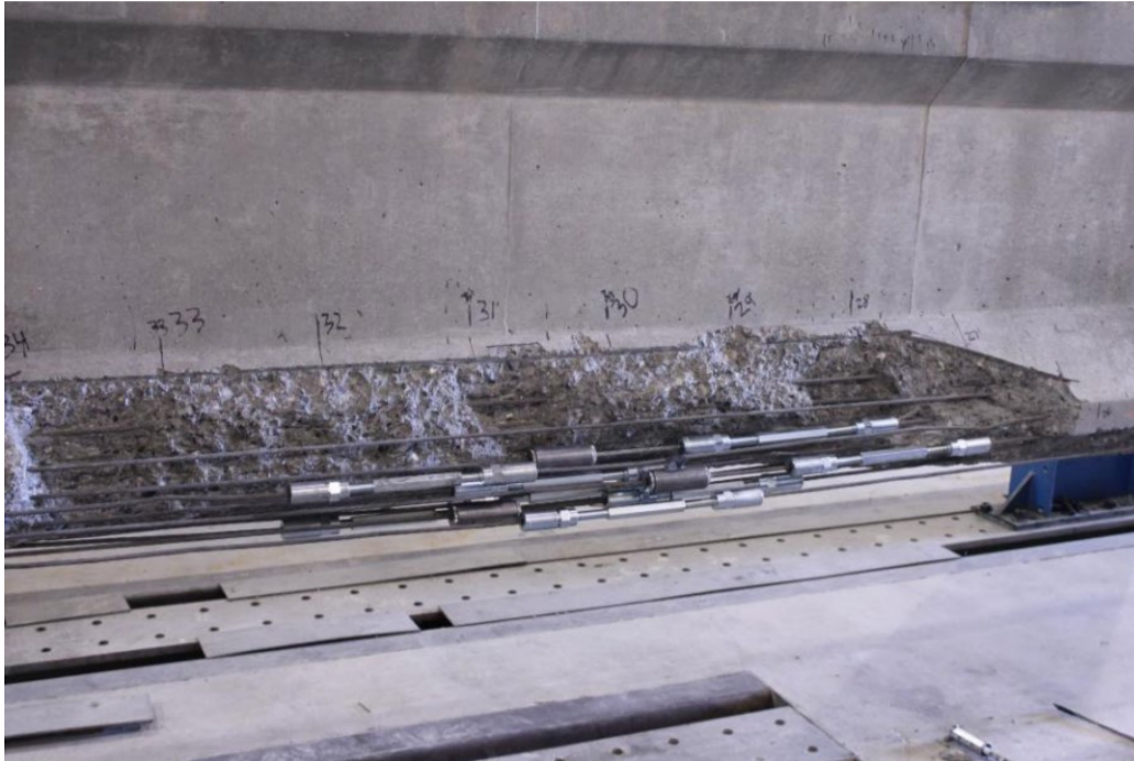
Figure 29: Strand splicing, courtesy of Jones, 2017
