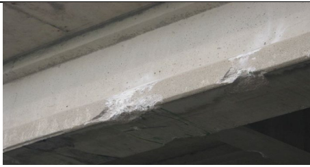
Figure 1: Minor damage, bottom flange spalling, Iowa DOT, 2014
