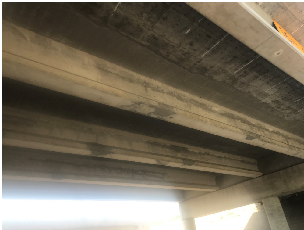
Figure 103: Replaced girder and girders with patching and epoxy injection works, I-680 over US-75 Bridge, courtesy of NDOT
