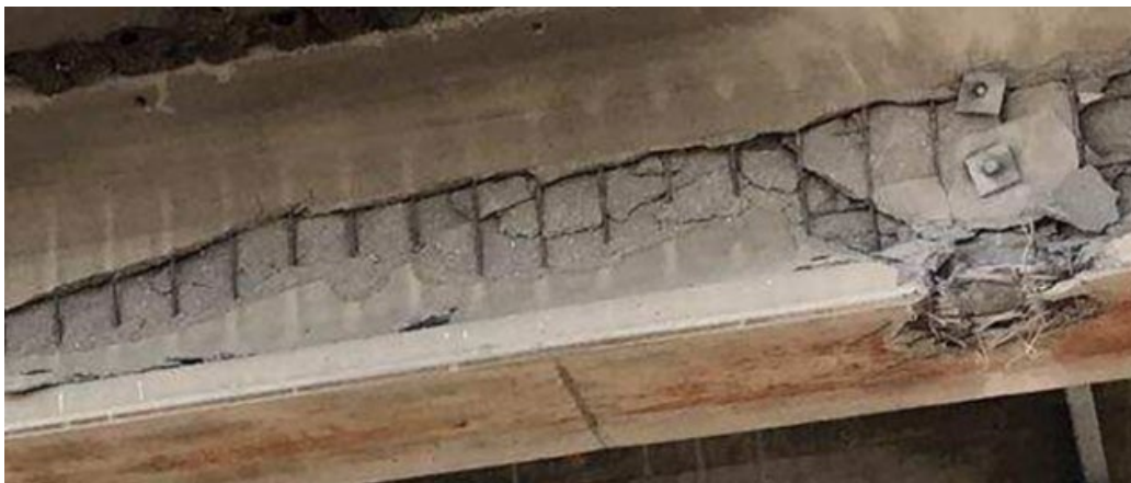
Figure 21: Severe III damage, several damaged strands, NDOT Schuyler Bridge, courtesy of NDOT
