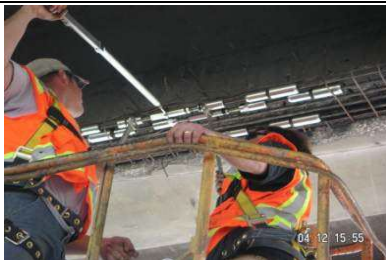
Figure 28: Strand splicing with a torque wrench, Enchayan, 2010
