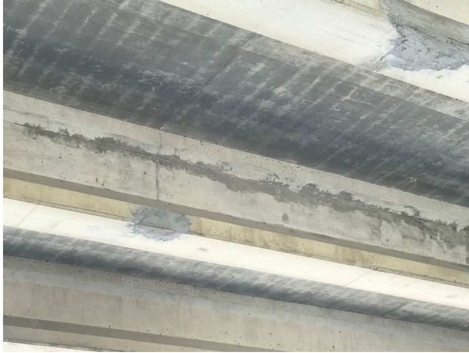
Figure 102: Girders with patching and epoxy injection works, I-680 over US-75 Bridge, courtesy of NDOT
