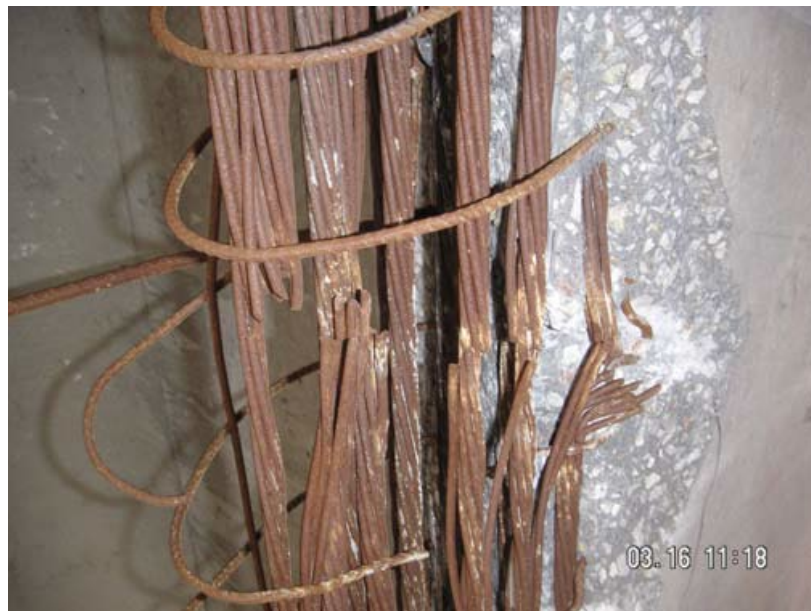
Figure 82: Girder (A) level of damage, Wood River Interchange Bridge, courtesy of NDOT
