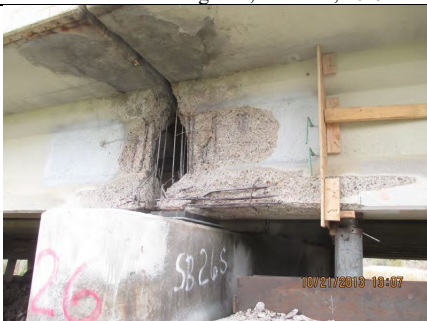
Figure 10: Severe damage, exposed strands > 15 %, MN/RC 2018-07 Report
