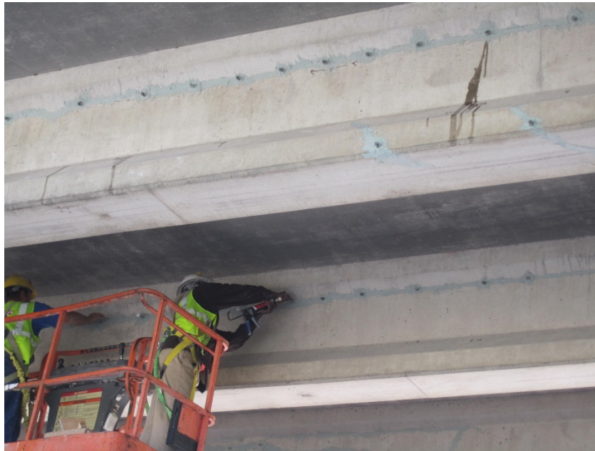
Figure 24: Epoxy injection process done in I-680 over US-75 Bridge, courtesy of NDOT
