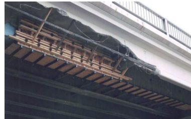
Figure 20: Patching plywood form to restore cross-section, AIT, 2005
