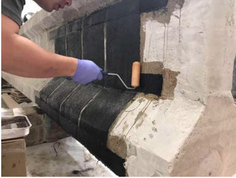
Figure 54: Applying shear CFRP to full-scale prestressed girder end, courtesy of Andrawes et al., 2018
