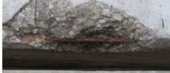
E: Corroded strand with heavy pitting
