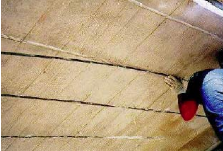
Figure 39: Use of near-surface mounted C-FRP in bridge decks, courtesy of Parretti et al 2004
