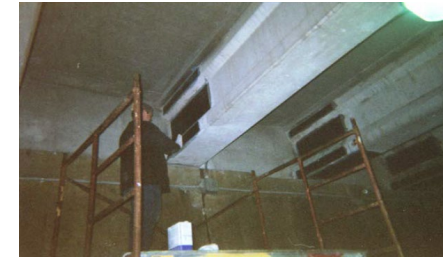
Figure 24: CFRP fabrics installation, Choo et al., 2013
