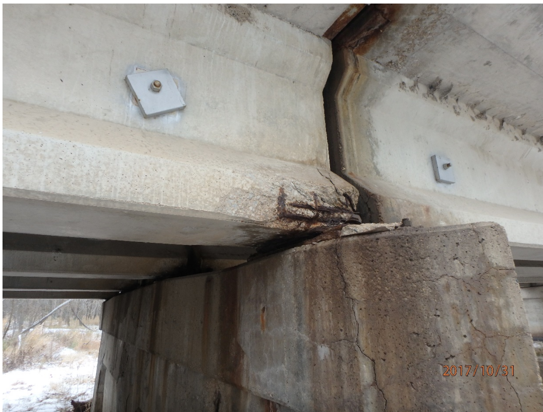
Figure 126: Damage at girder ends, Platte River South Bridge, courtesy of NDOT
