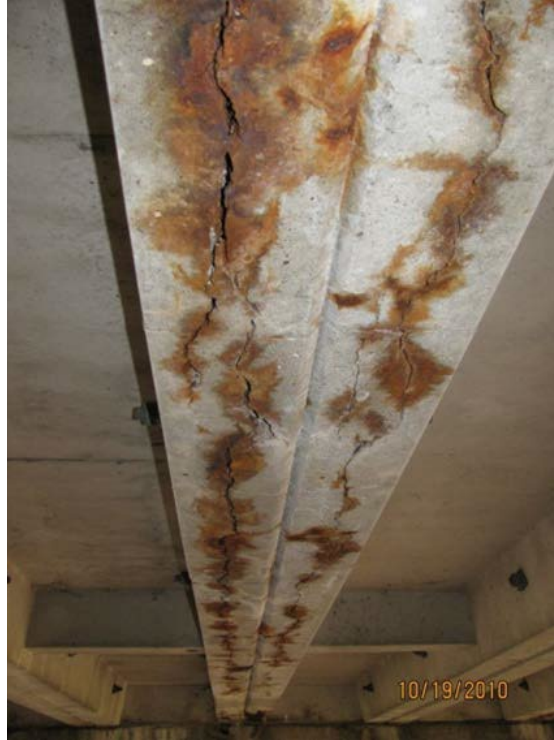
Figure 47: Condition State 3 cracking, delamination, and rust staining a precast concrete channel girder, courtesy of MnDOT, 2019
