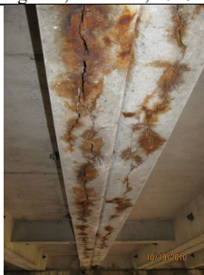
Figure 7: Extensive damage, delamination, and rust staining a precast concrete channel girder, MnDOT, 2019
