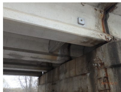
Figure 11: Severe damage, exposed strands, NDOT Platte River South Bridge
