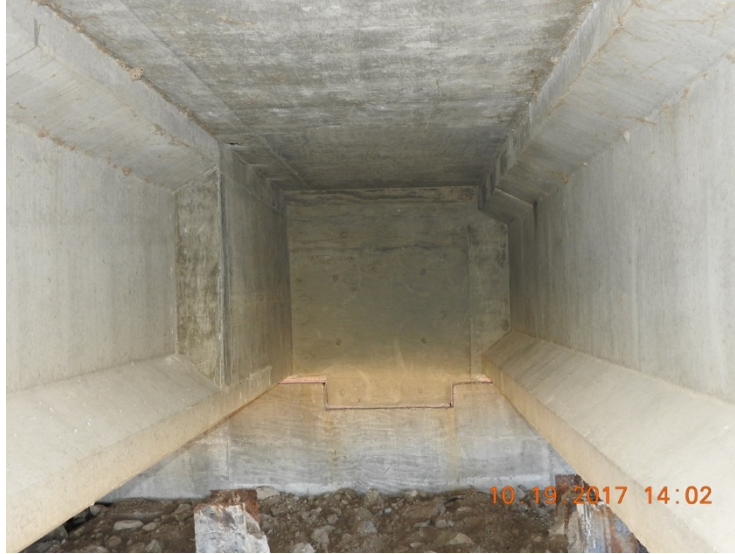
Figure 133: Repaired girder end with a concrete encasement, Alma South Bridge, courtesy of NDOT
