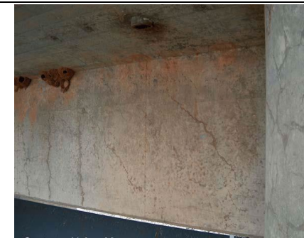
Figure 3: Moderate damage, hairline cracks, WisDOT, 2018
