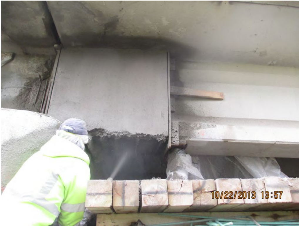
Figure 52: Shotcreting the bottom surface of the repair at girder end, MN/RC 2018-07 Report
