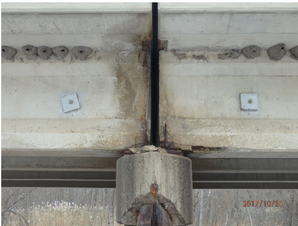
Figure 125: Damage at girder ends, Platte River South Bridge, courtesy of NDOT
