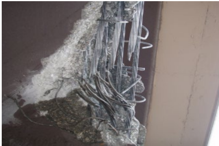
Figure 20: Severe II damage, three severed strands, NDOT Scottsbluff Gering Bypass Bridge, courtesy of NDOT
