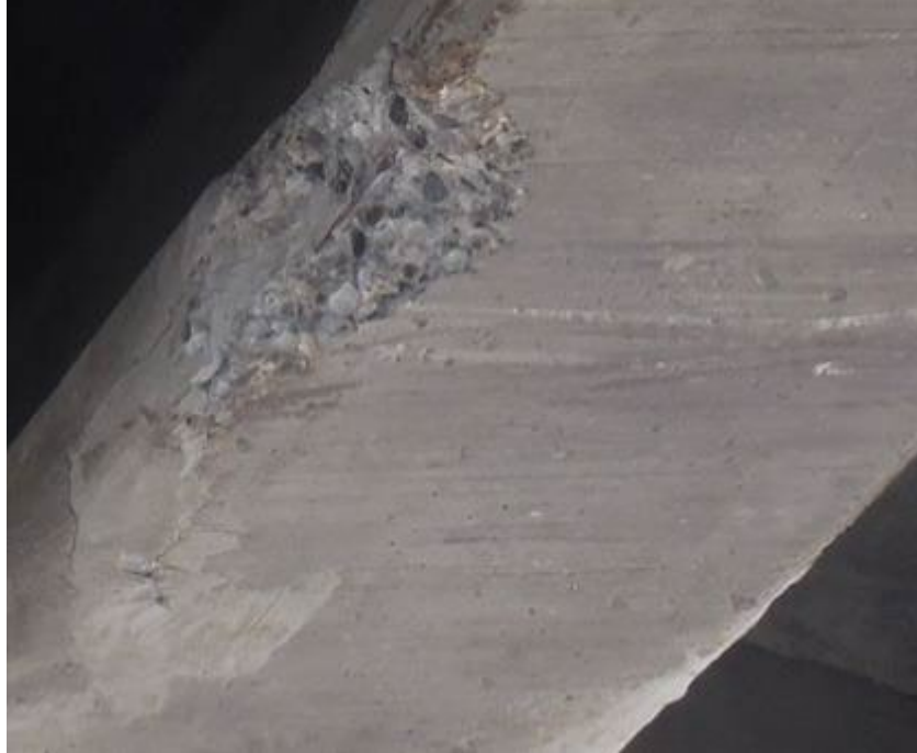
Figure 43: Condition State Fair, exposed strand on concrete bridge girder, courtesy of WisDOT, 2018
