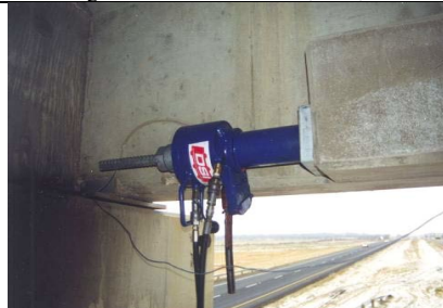
Figure 29: External post-tensioning end block, AIT, 2005
