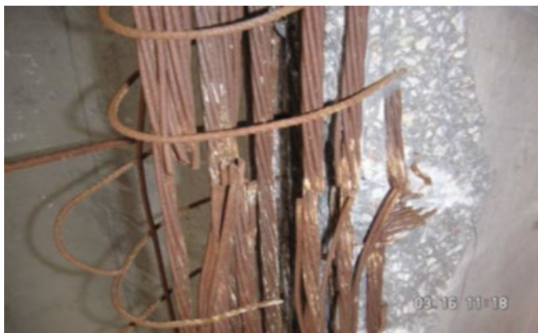
Figure 18: Severe II damage, five severed strands, NDOT Wood River Interchange Bridge Girder (E), courtesy of NDOT
