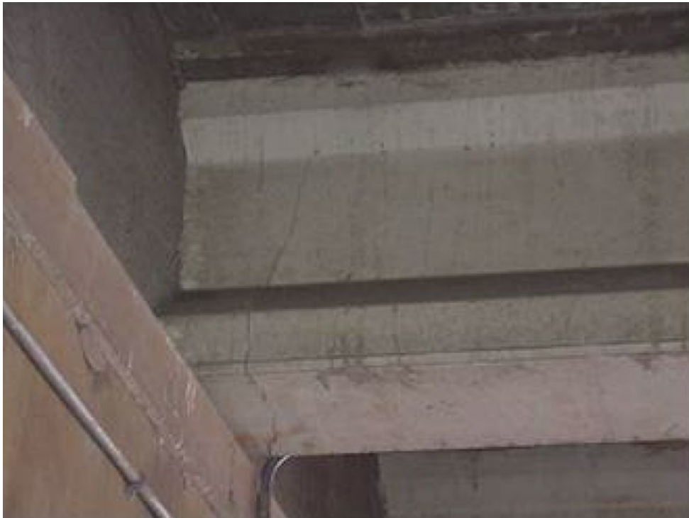
Figure 49: Severe class corrosion damage at girder end causing severe cracks, courtesy of Choo et al., 2013
