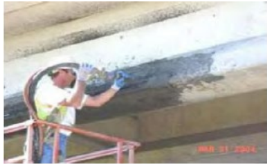
Figure 19: Shotcrete patch, Harries et al., 2012
