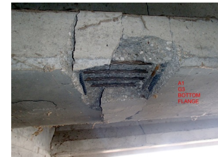
Figure 12: Severe damage, exposed strands, severe cracks or fractures, NDOT Alma South Bridge
