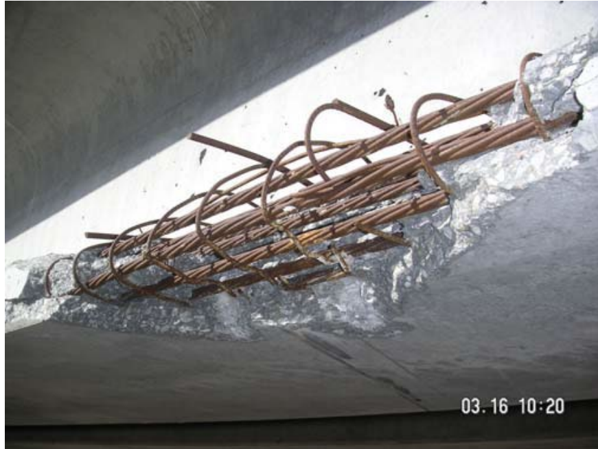
Figure 82: Girder (A) level of damage, Wood River Interchange Bridge, courtesy of NDOT
