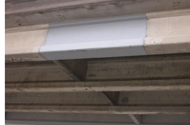
Figure 23: FRP Wrapped Repair, Iowa Dot, 2014
