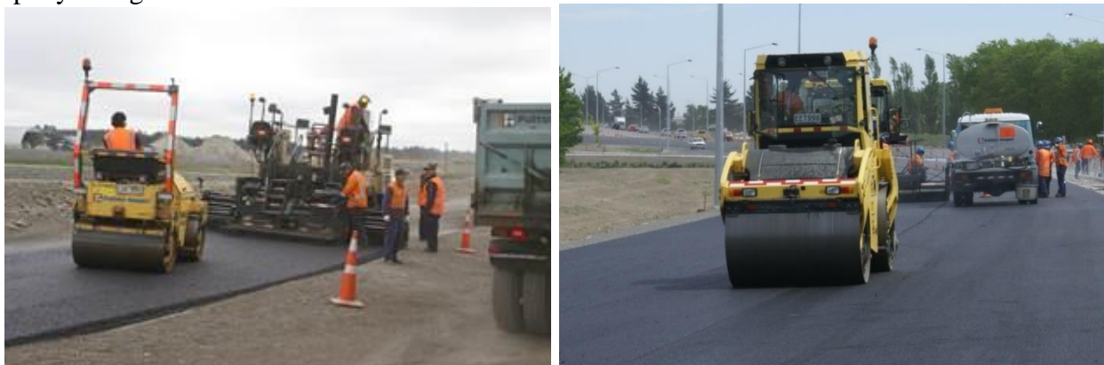
Figure 30. Compaction of EMA OGFC Pavements in New Zealand (Waters et al., 2018)
