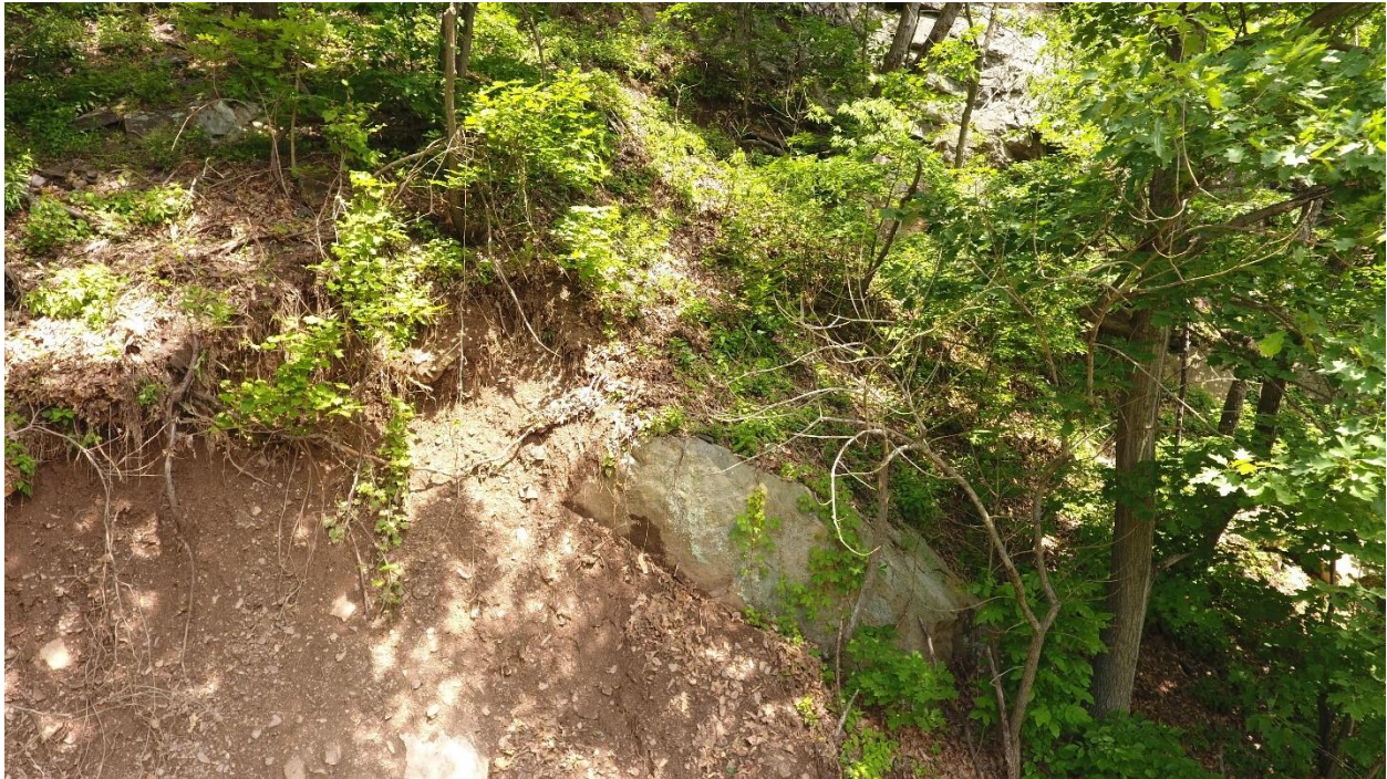
Figure 5. View of the Landslide Point of Origination Recorded by the UAV
