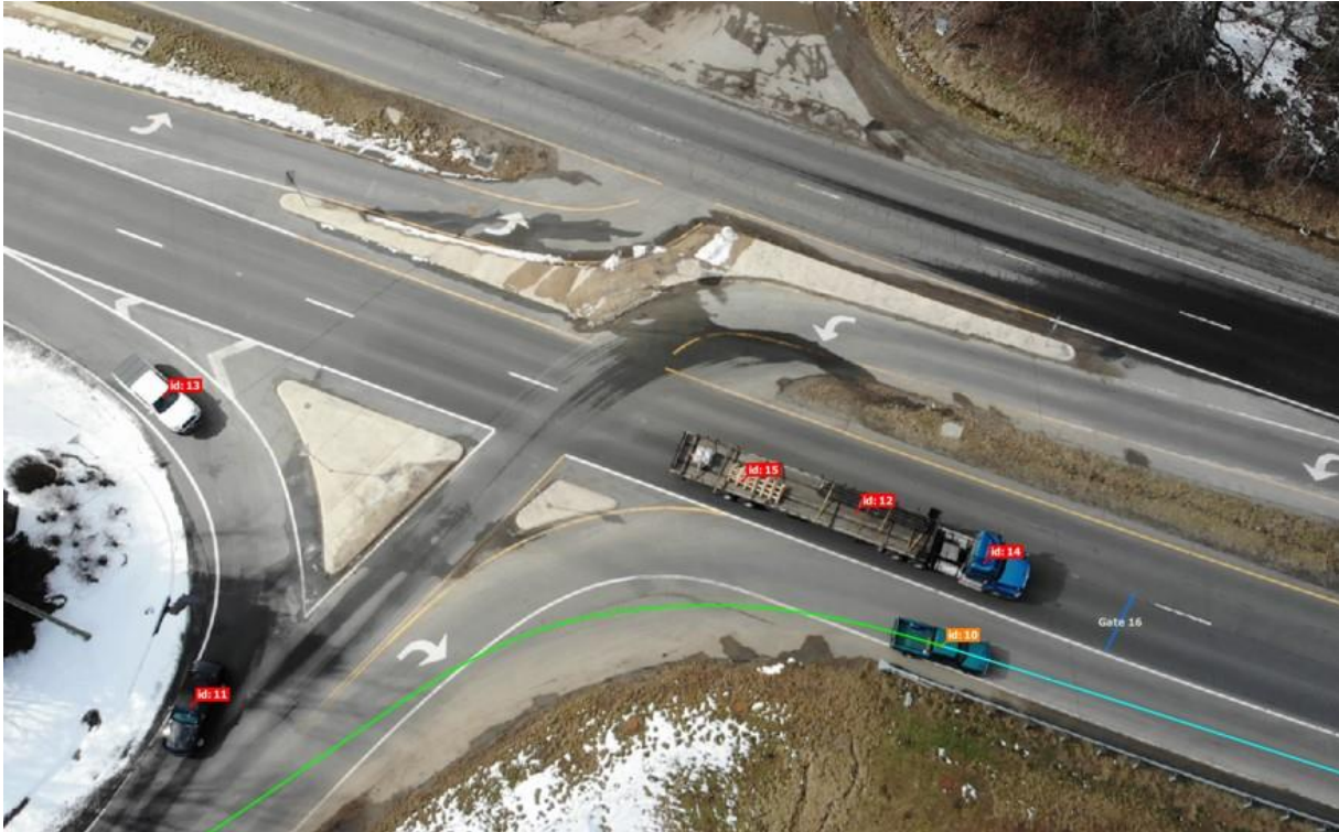
Figure 20. View of Intersection 1 (US 460 at North Main Street (Business 460) in the DFS Software Showing Vehicles and Respective Identification Tags (Red)
