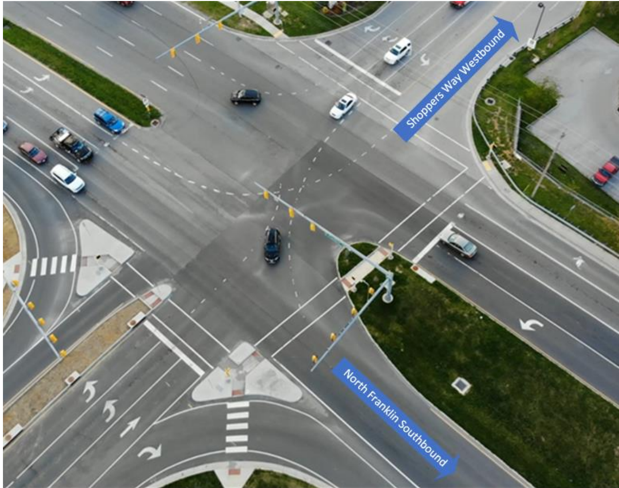
Figure A5. Aerial View of Intersection 6 at North Franklin St. and Shoppers Way in Christiansburg, VA
