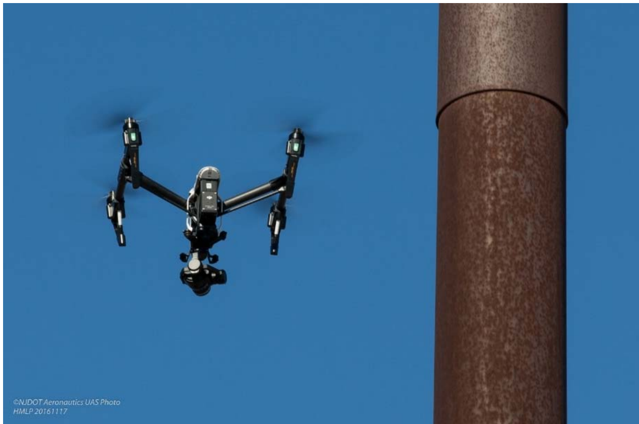
Figure 6. UAS Inspecting a High Mast Light Pole Source: NJDOT Aeronautics, 2016.
