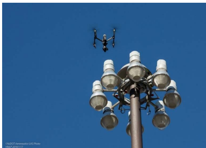
Figure 2. Unmanned Aerial Vehicle and High Mast Light Pole
