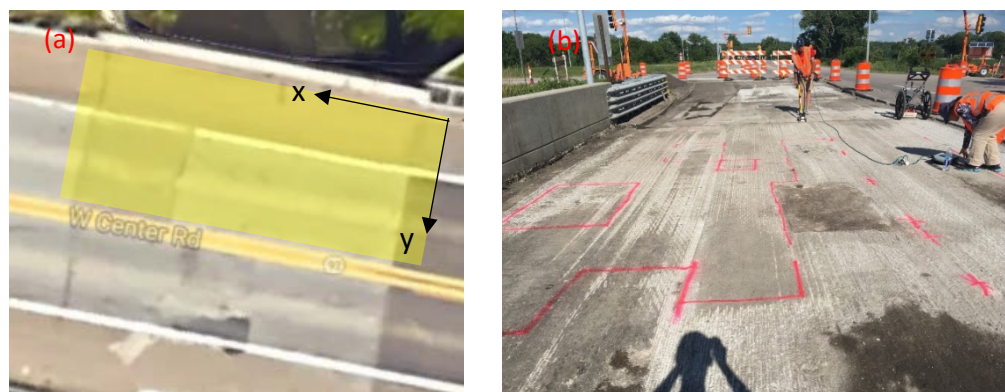
Figure 5-16 Bridge 2: (a) Google map and the scanned area, (b) Concrete deck after asphalt removal
