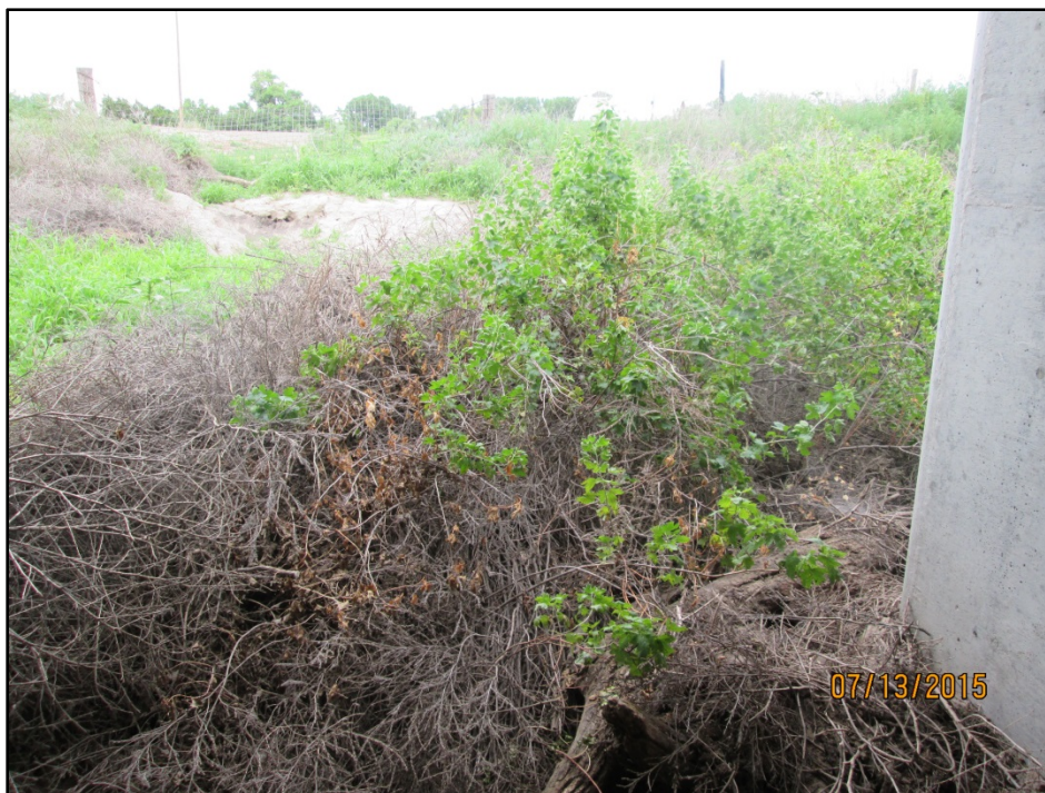
Photo 2: Vegetation surrounding structure. Orientation: North
