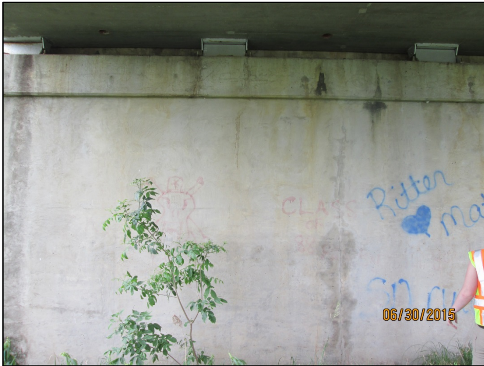
Photo 3: Side of structure. Orientation: West
