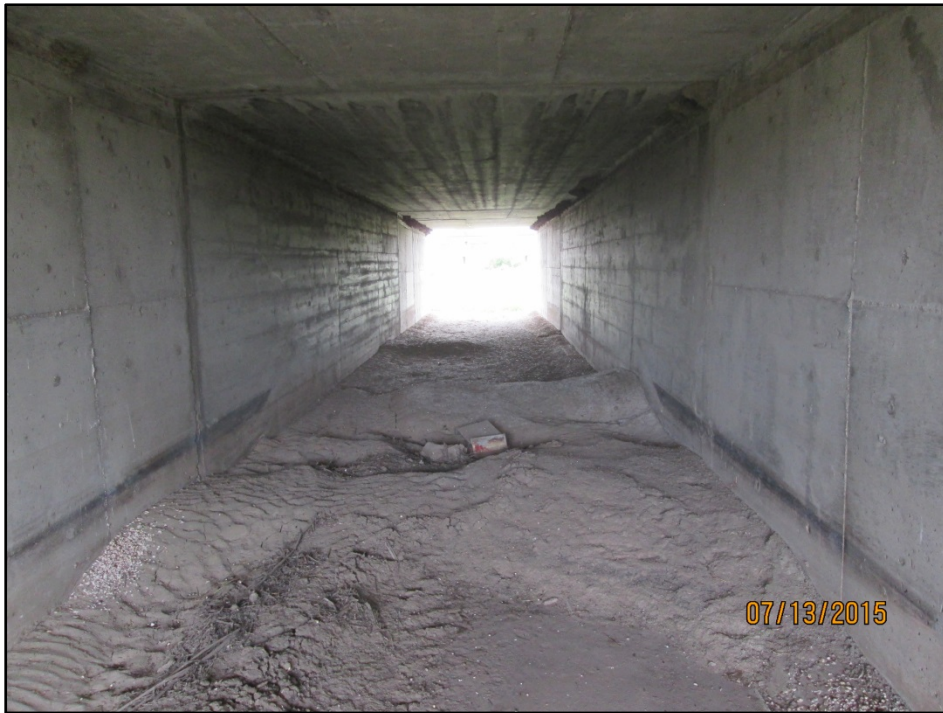
Photo 3: View inside the structure Orientation: South
