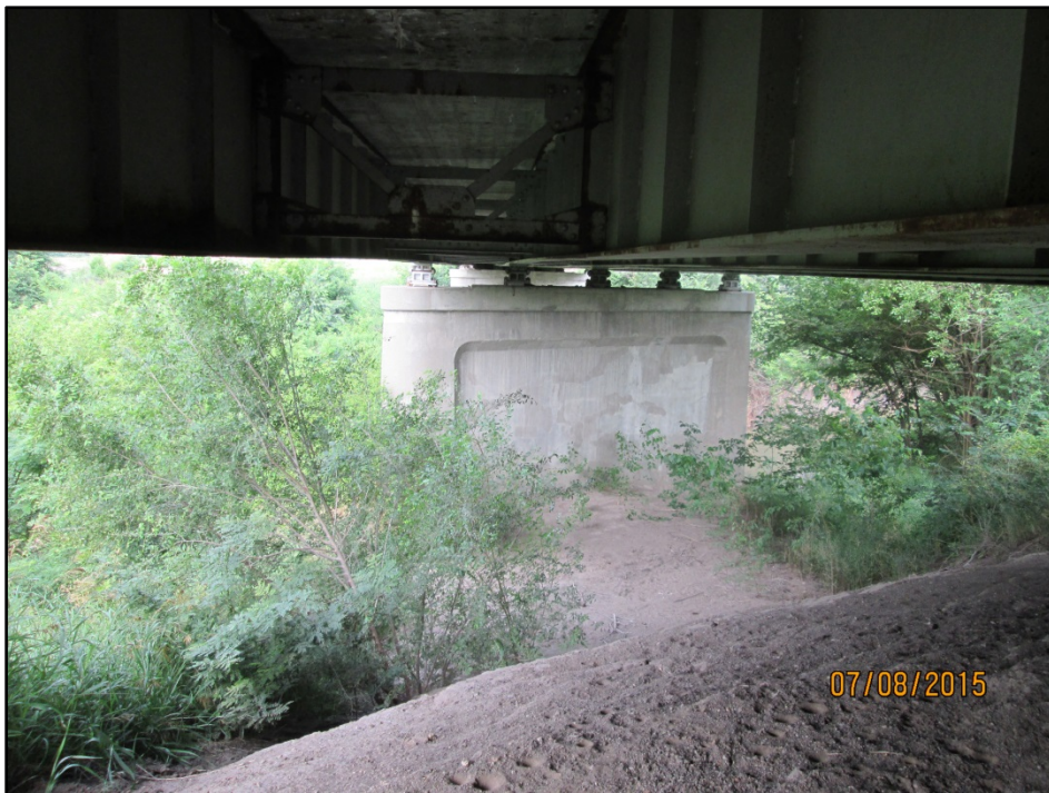
Photo 5: Midsection underneath bridge Orientation: West
