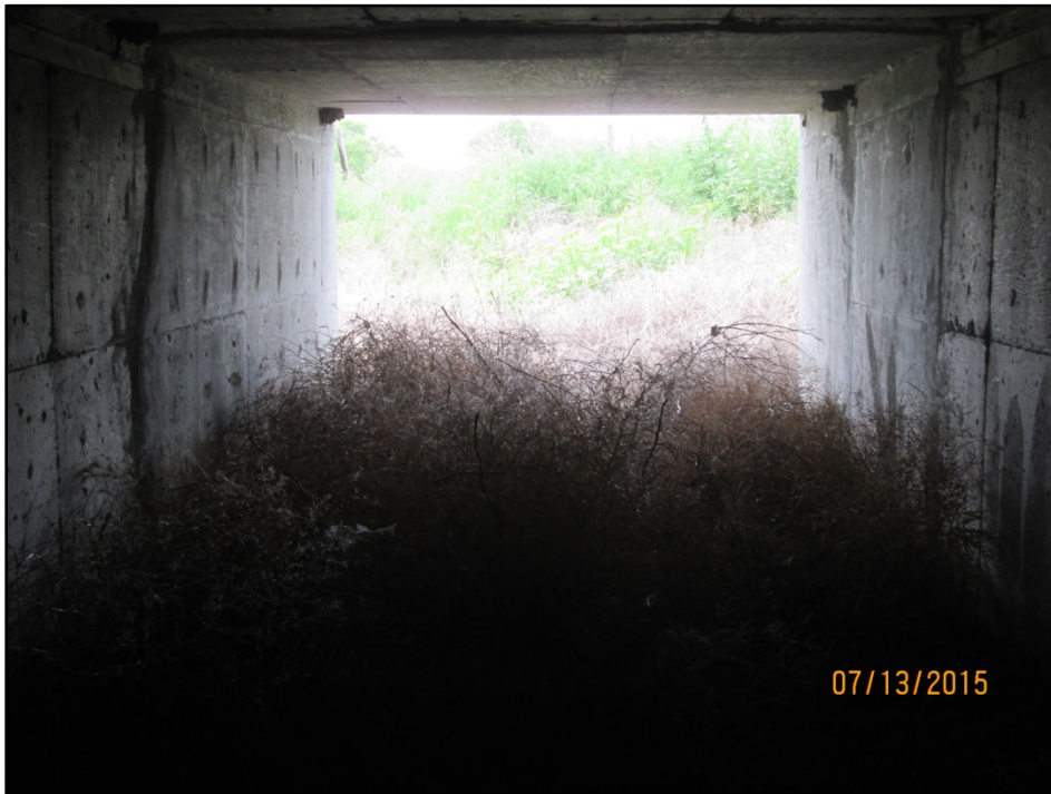
Photo 4: Looking south inside the structure. Orientation: South
