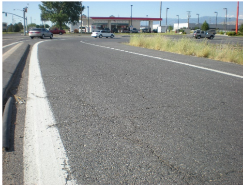
(a) Ramp facing north
