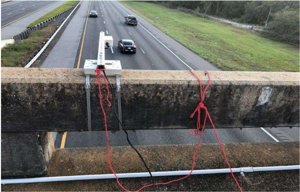
Figure 93: Capture Unit During Installation
