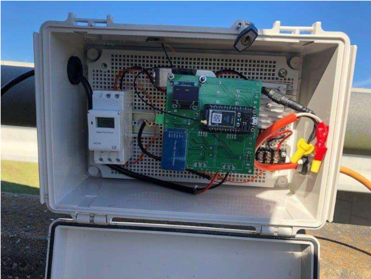
Figure 76: Gateway Showing Modern and Relay Units
