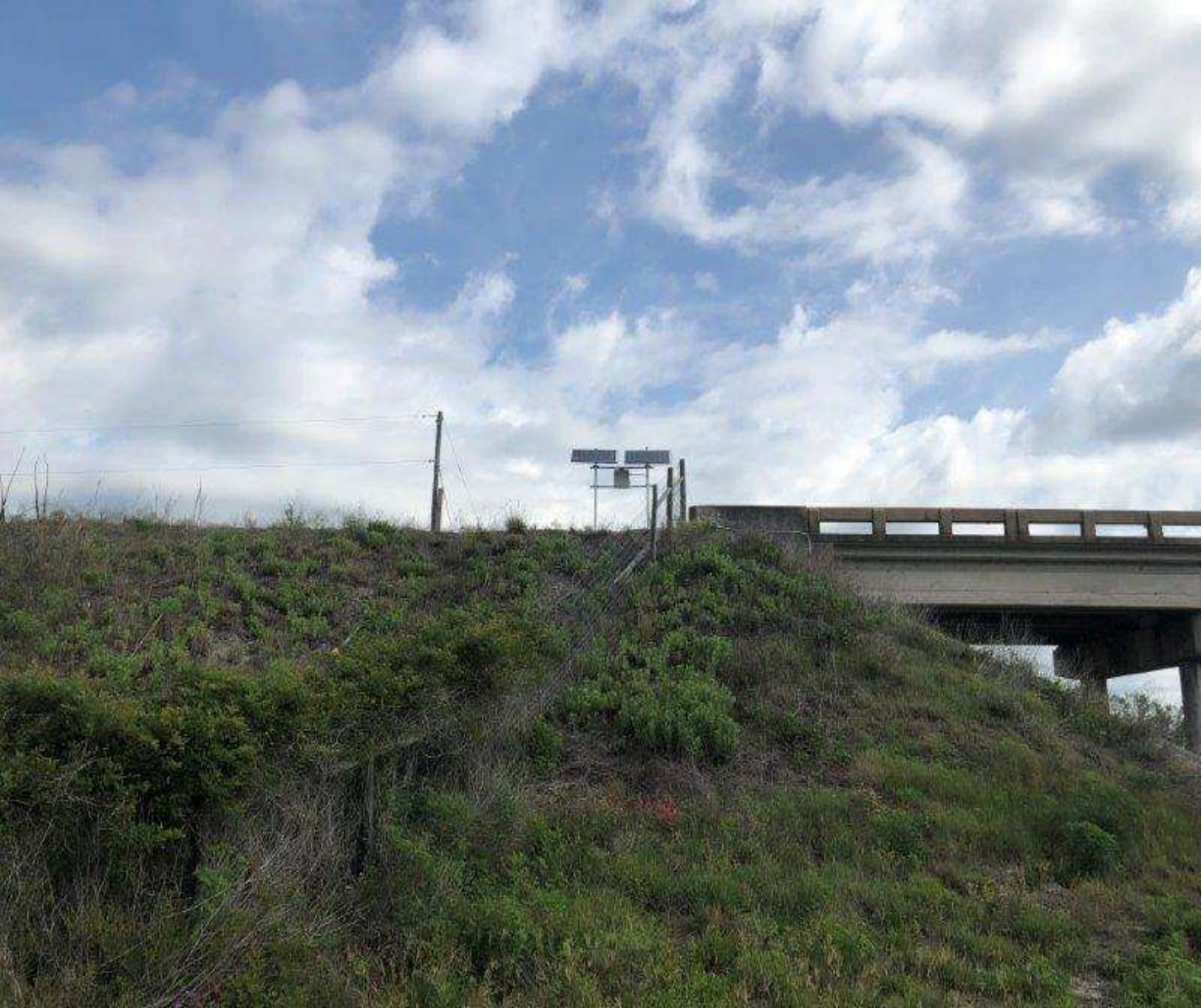
Figure 87: Solar Unit: Site 2
