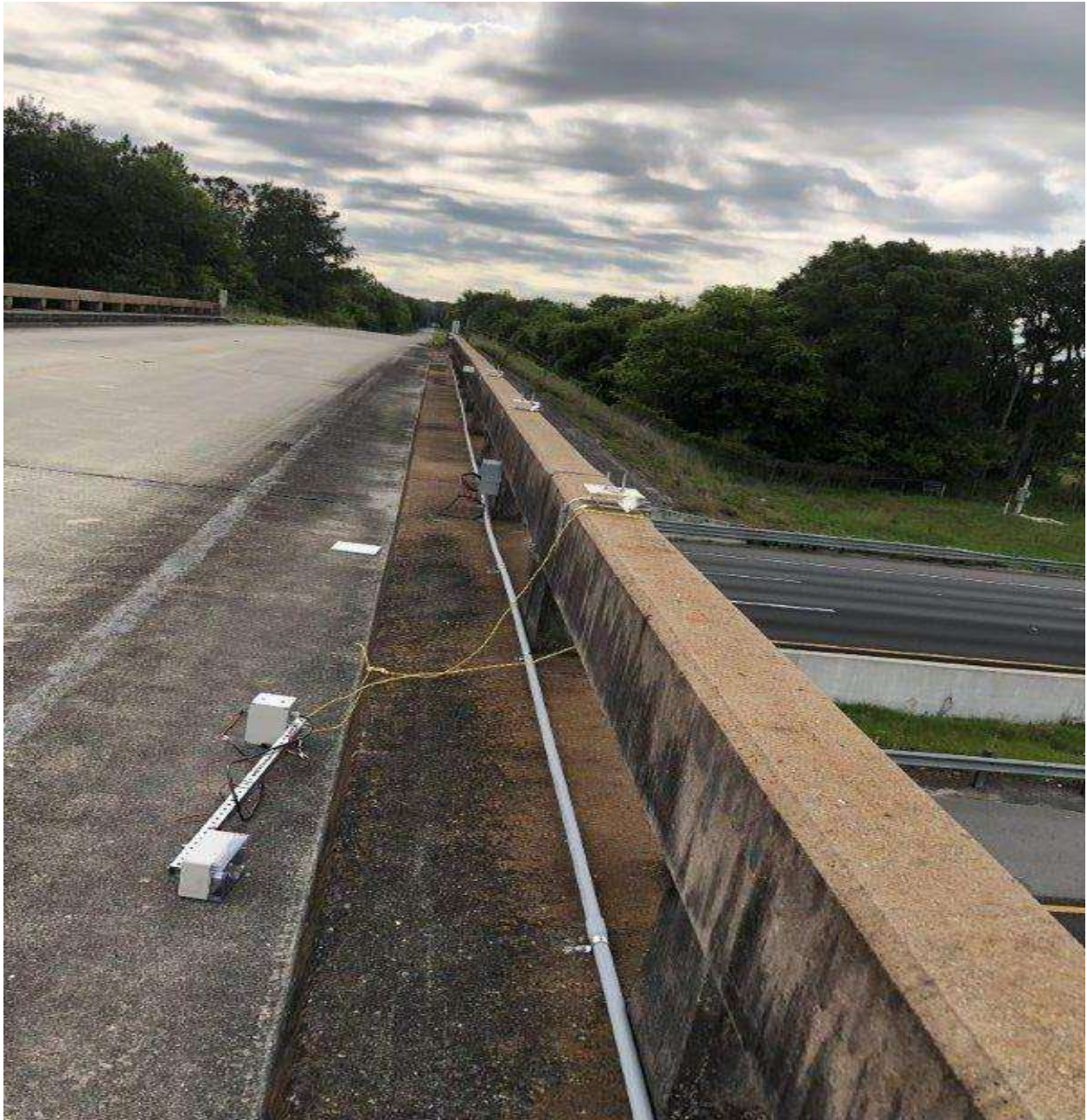
Figure 104: Tethered Bracket before Installation
