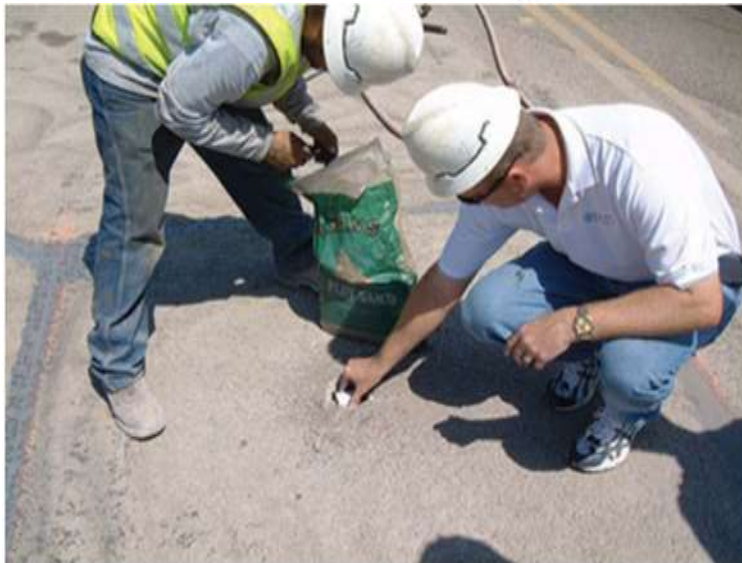
Figure 2: Wireless Magnometer and the Installation Process
