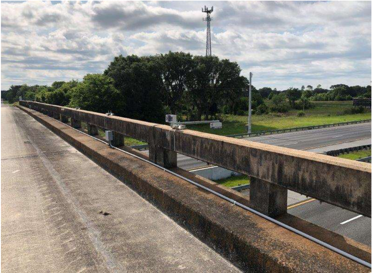
Figure 91: Site 2: Gateway Unit and Capture Unit
