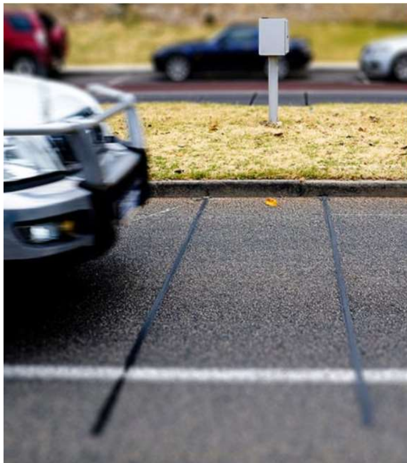
Figure 5: Fixed and Embedded Types of Pneumatic Detectors
