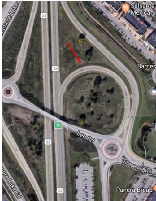
Figure 5-60 The Lee Rd Bridge and the merge onto Lee from US-23 NB
