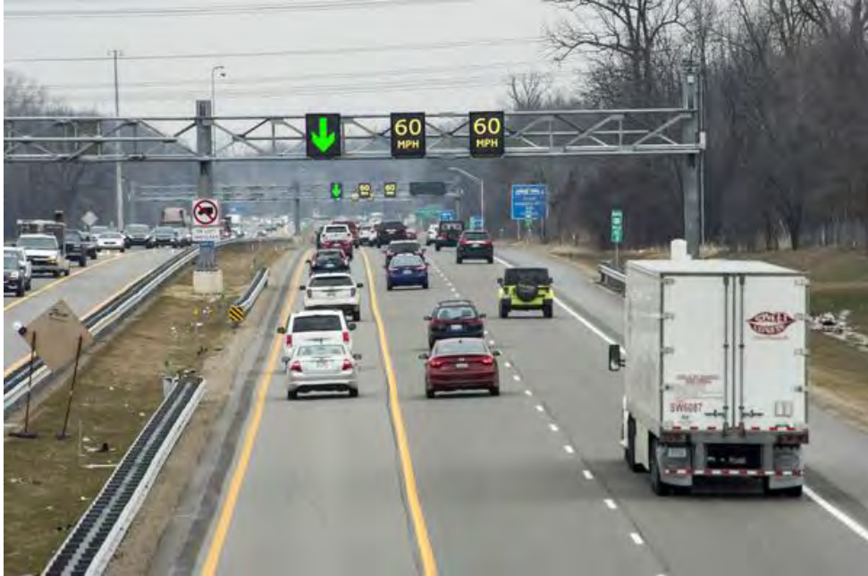
Figure 1-1 US-23 Flex route in operation
