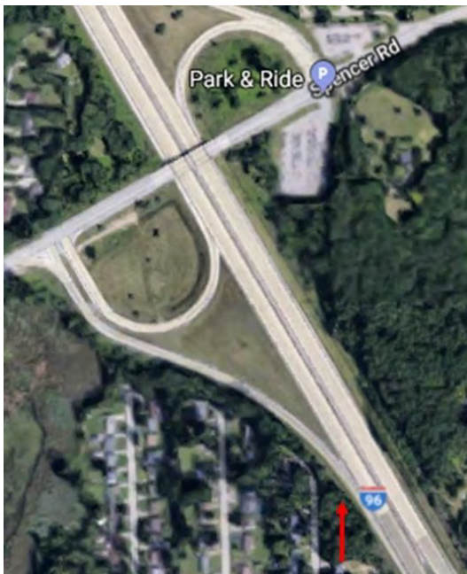
Figure 5-57 The entrance onto I-96 EB from Spencer Rd, which continues east and is where Spencer comes to a dead stop from 70 down to 0
