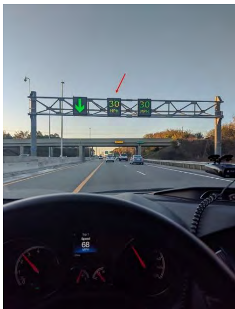
Figure 5-61 Gantries after the rest stop that changed to 30 from 40 mph
