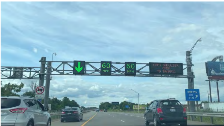
a. ii) Gantry at MM 51.3 northbound
