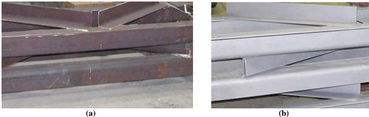
Figure 19. Secondary Members: (a) before being blast cleaned; (b) after being blast cleaned with garnet media to remove mill scale and surface stains
