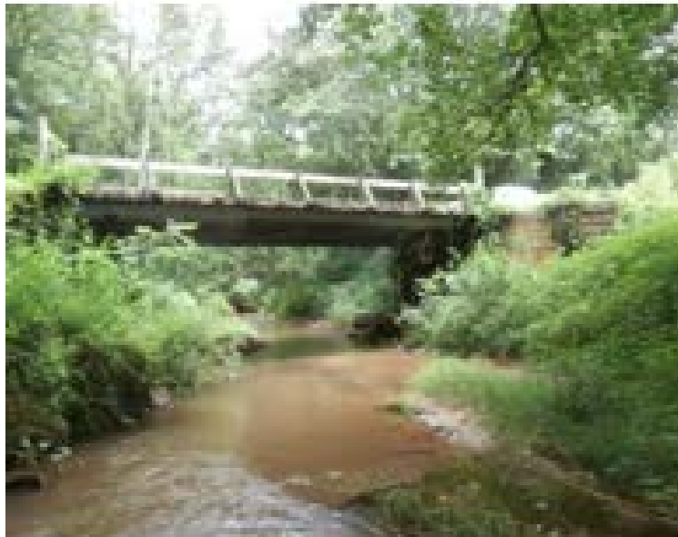
Figure 1. Bridge From Which the 20 I-Beam Samples Were Taken
