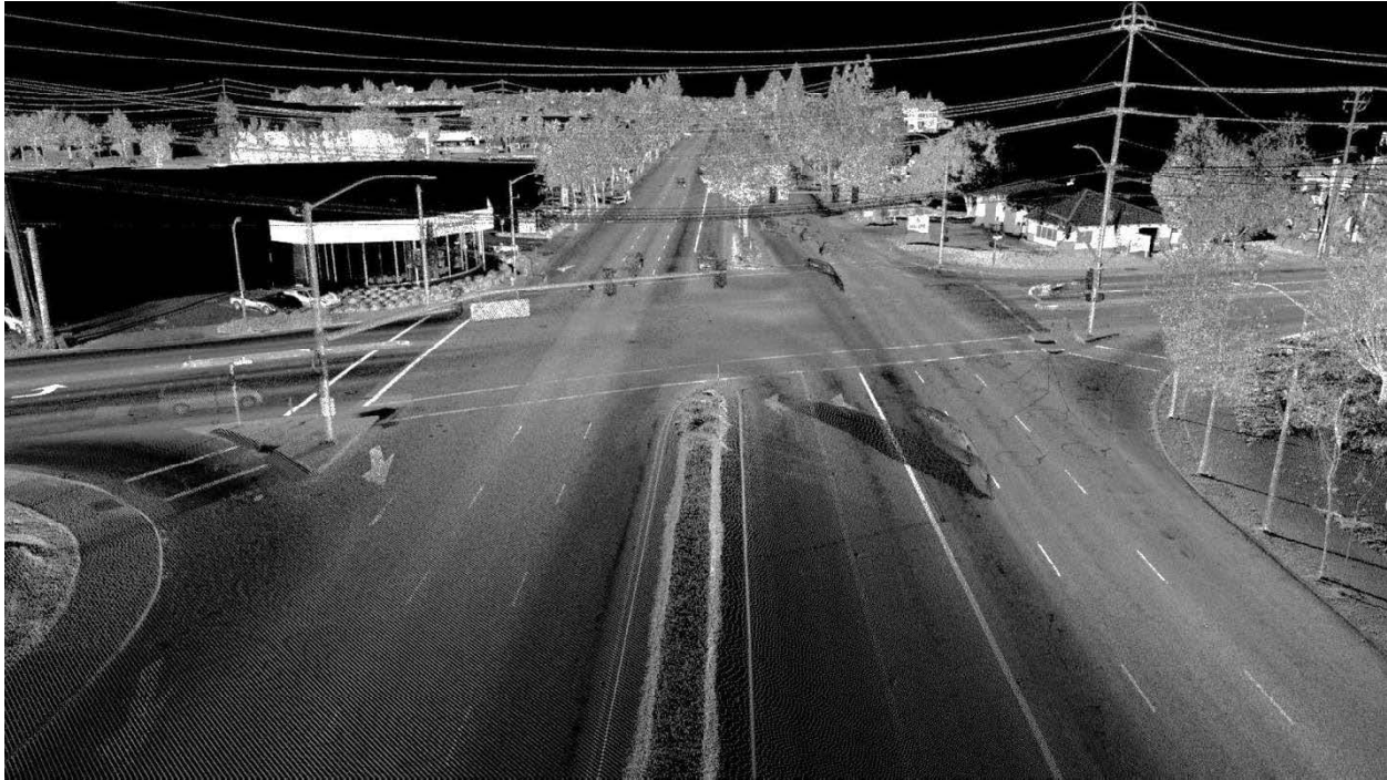
Figure 6.7: Point cloud rendering of the El Camino Real Boulevard/West Charleston Road intersection
