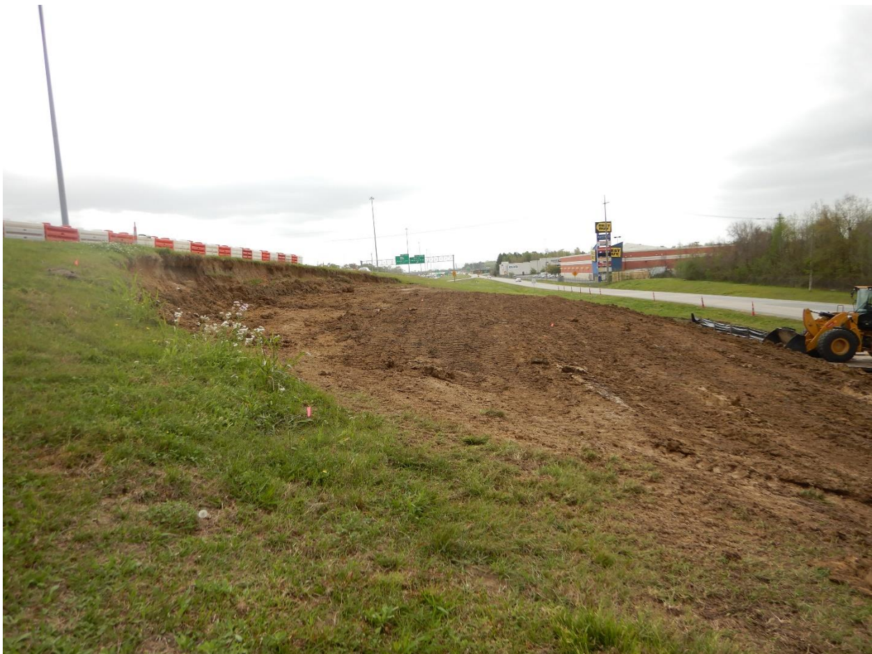
Figure 1. Failed embankment site at I-10 and Bluebonnet Blvd., Baton Rouge, LA.
