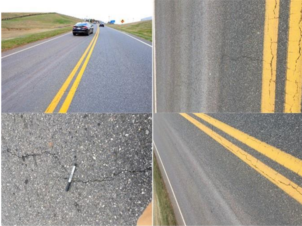
Figure 13. Surface Conditions at Albemarle County Site in 2018
